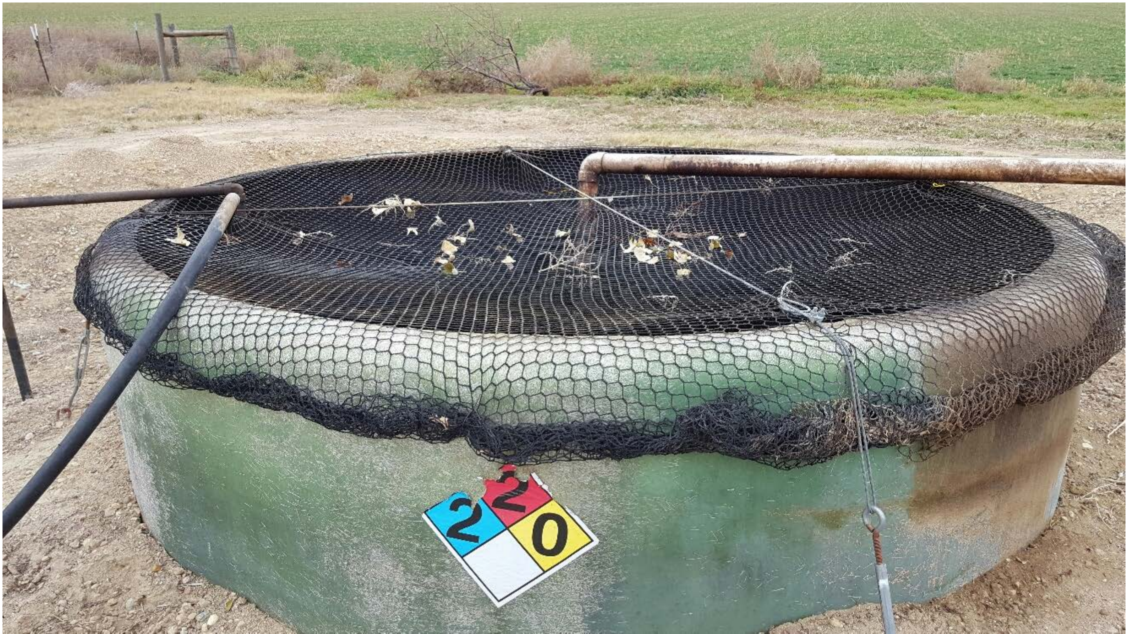
Figure #5 Wildlife netting has been repaired.
