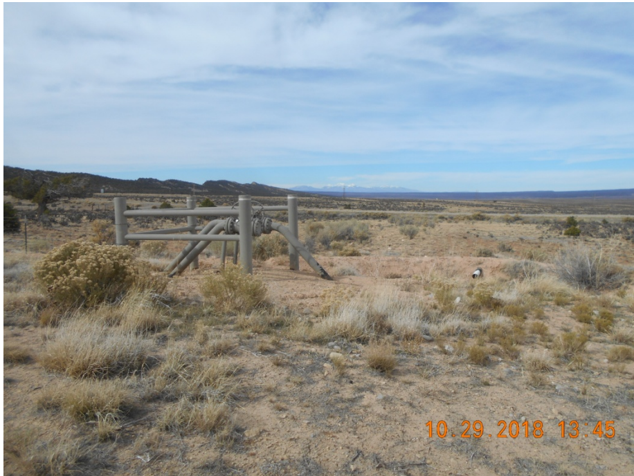
6" flowline risers with valves
