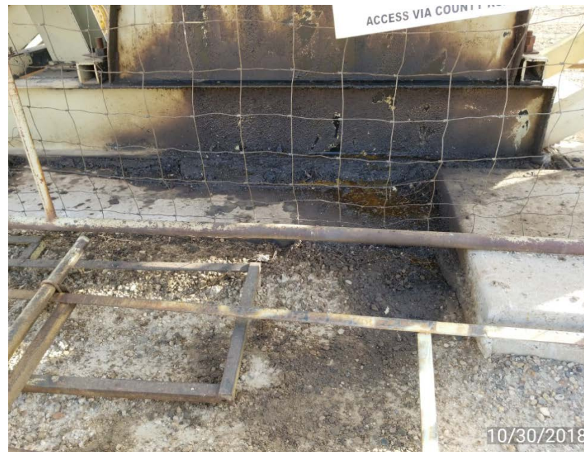
Oil from pump jack on ground – south side
