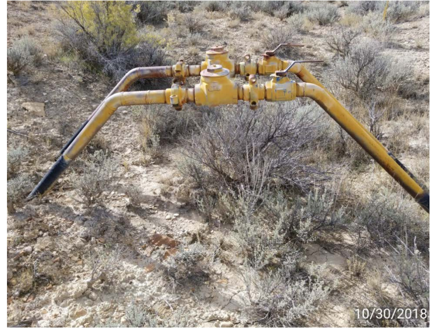
Well flow line located 200' north of building. Gas movement is audible.
