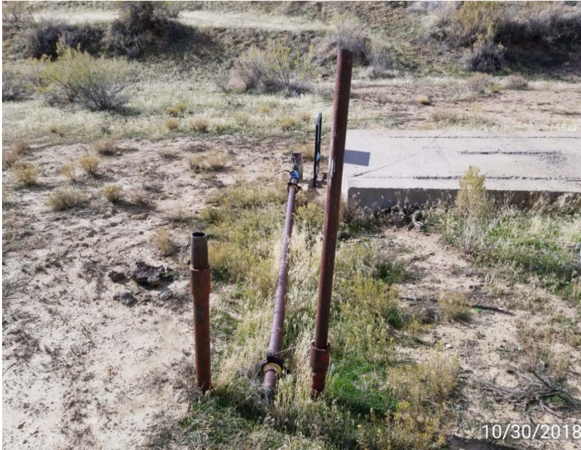
Uncapped risers at well head
