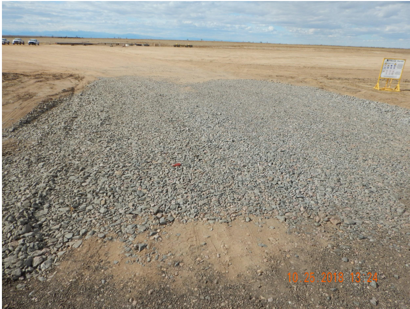
Photo 1. Photo taken from the entrance of the location, facing West. Tracking pad devices installed at the entrance off County Road 51 appears to be in proper functioning condition.
