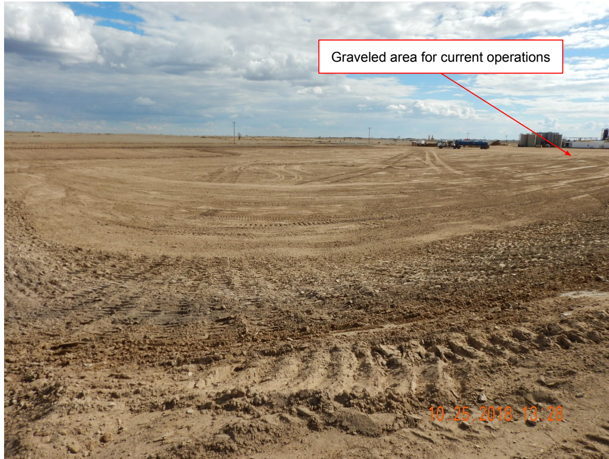
Photo 11. Photo taken from the northwestern location, facing Southeast. Photo illustrates the northern well pad area which has been compacted but not necessarily stabilized from wind erosion. Operator shall ensure compliance with Rule 1002.e.(1) to reasonably control dust and minimize erosion which includes wind erosion.
