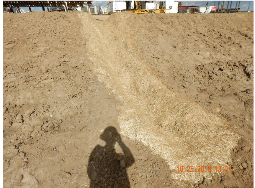
Photo 4. Photo taken from the southern location, facing North. Photo illustrates a temporarily stabilized outlet along the fill slope that is directed to the ditch and berm BMP. Fill slopes have been temporarily stabilized with equipment tracking.
