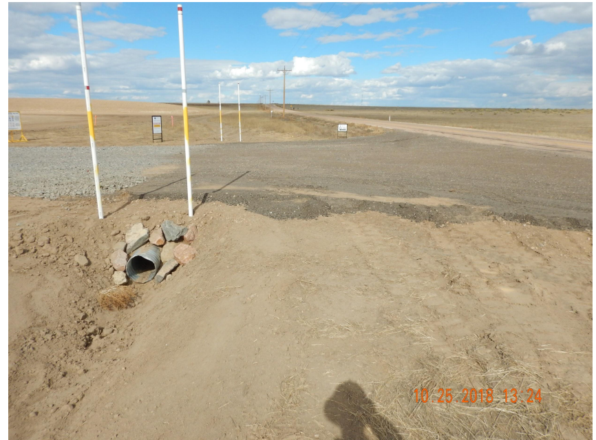
Photo 8. Photo taken from the entrance of the location, facing North. Photo illustrates a culvert installed in conjunction with the ditch and berm BMP. Also, photo illustrates the vehicle tracking devices.
