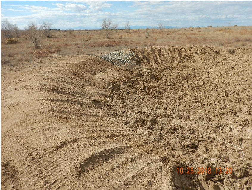
Photo 3. Photo taken from the southwest location, facing West. Photo illustrates a retention area with a stabilized outlet.
