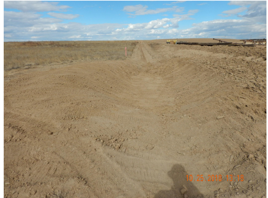
Photo 2. Photo taken from the western location, facing North. Photo illustrates a retention area installed in conjunction with a ditch and berm BMP. Appears portions of the berm have been tracked with equipment for temporary stabilization but portions have been left unconsolidated.
