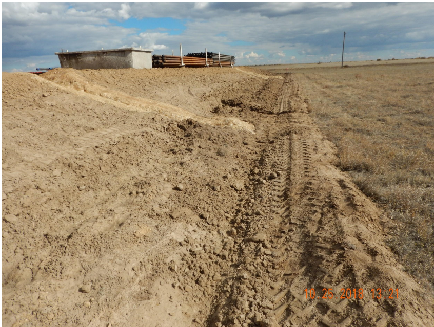
Photo 5. Photo taken from the southern location, facing East. A total of three temporary outlets have been installed along the southern fill slope. See comments under Photo 4. Photo illustrates the ditch and berm BMP. Does not appear portions of the berm have been sufficient stabilized.
