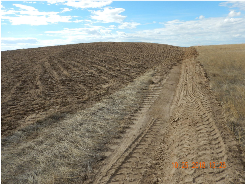
Photo 9. Photo taken from the northeastern location, facing West. Photo illustrates the topsoil stockpile that has been temporarily stabilized with equipment tracking.
