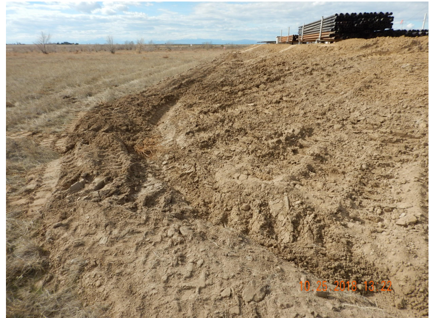
Photo 6. Photo taken from the southeastern location, facing West. Photo illustrates equipment that has damaged the ditch and berm BMP. Operator shall ensure stormwater BMPs are in proper functioning condition.
