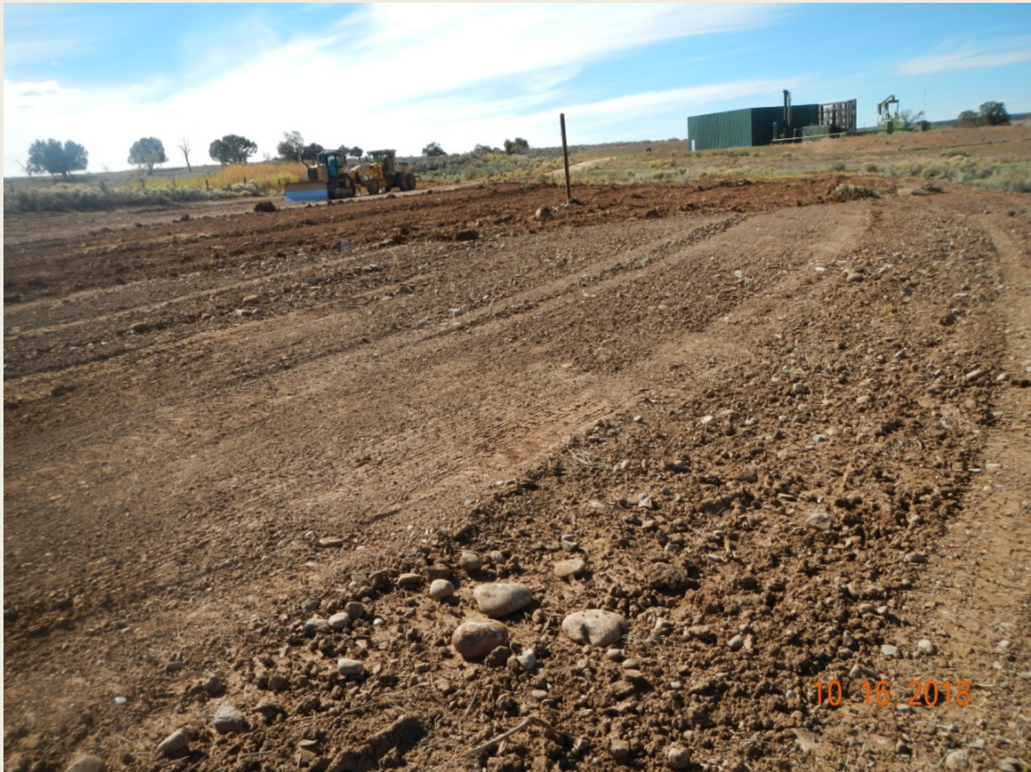
Photo 1. View of the project area from the northeastern corner facing center. Well pad is recently countoured. It appears topsoil is being spread.
