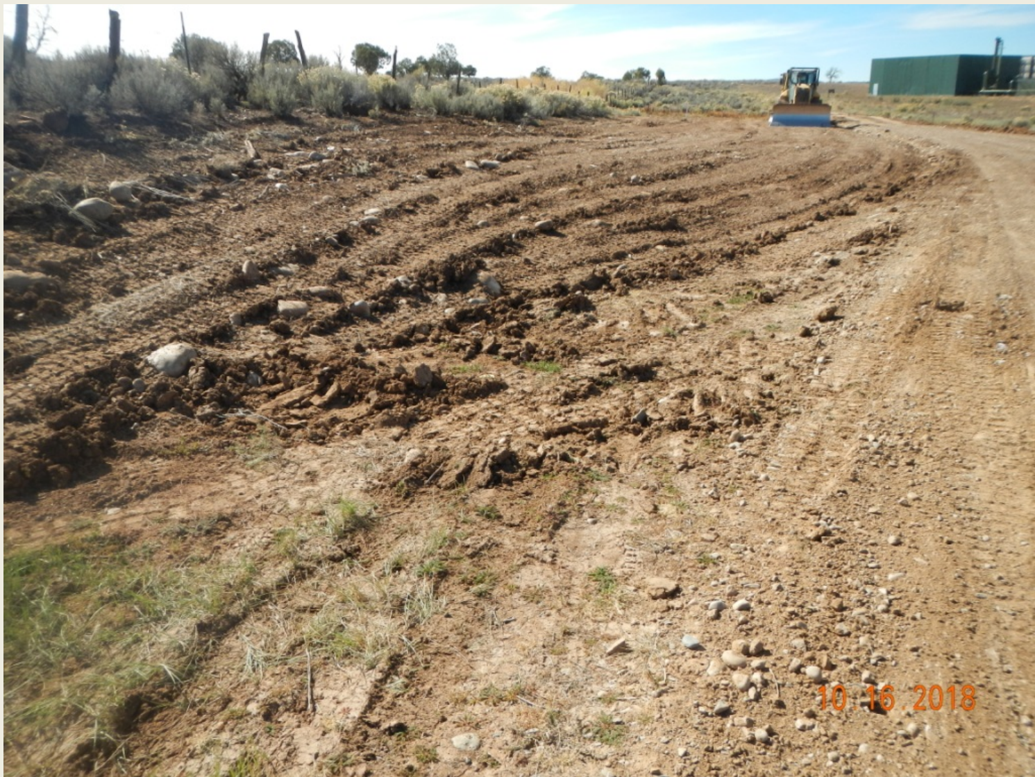
Photo 4. View of southern project area from the southeastern corner facing westward. Recontouring and other reclamation is in process.
