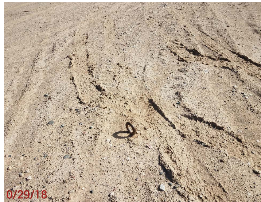
Location Photo #10, unmarked deadman on South side of location
