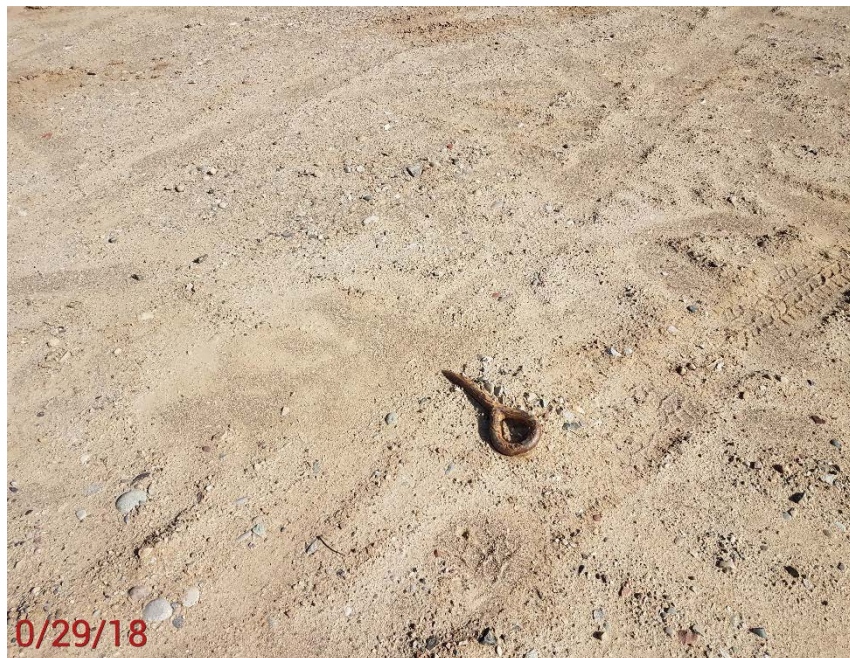
Location Photo #9, unmarked deadman on South side of location
