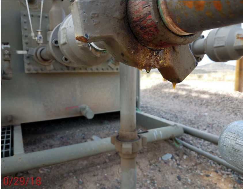
Location Photo #5, dripping fitting on flowline
