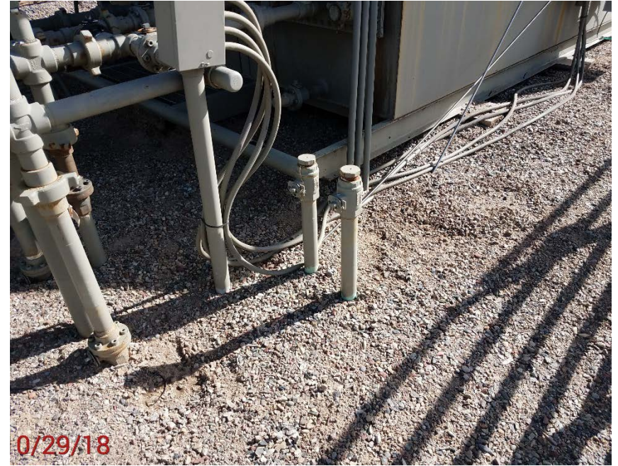
Location Photo #4, unmarked flow lines.
