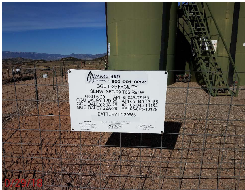
Location Photo #5, Missing access road information on battery sign
