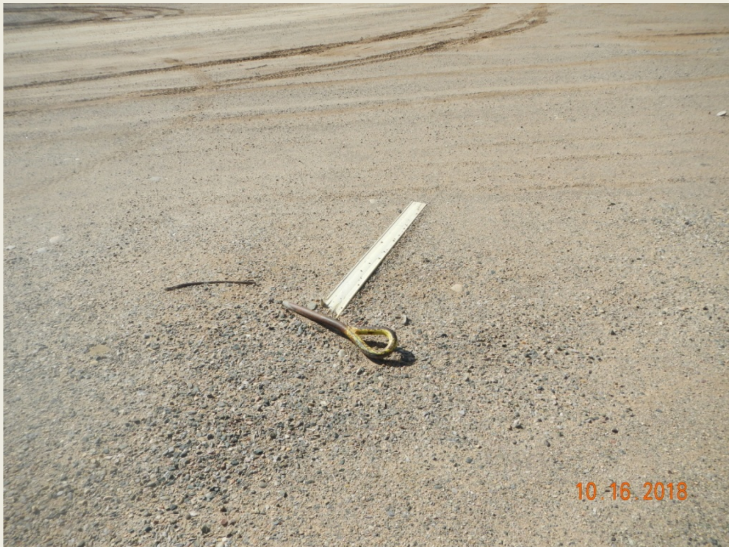
Photo 5. View of anchor marker that is broken and needs to be replaced.
