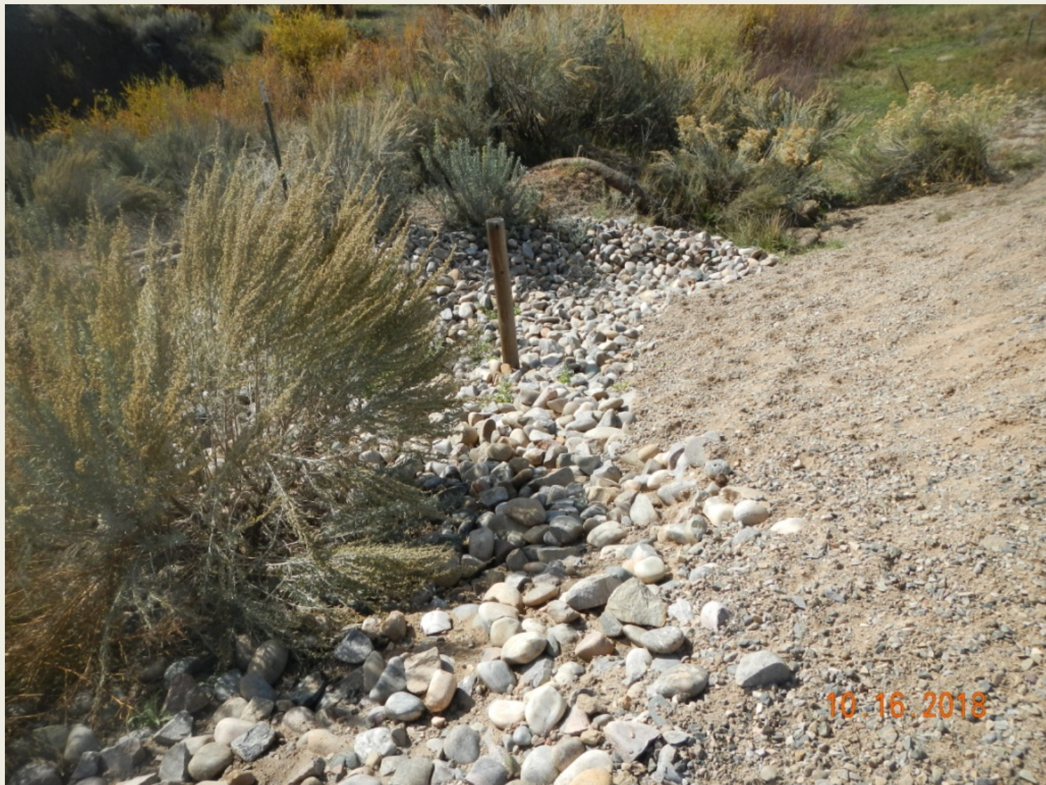
Photo 6. View of cobble run-down in the southwestern project area, appears to be functioning.
