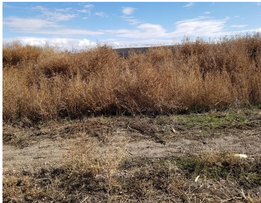
Photo 6 – Perimeter berm not visible below weeds; thin crust of transported bentonitic material on top of native soil.
