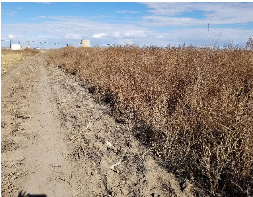
Photo 5 – Perimeter berm not visible below weeds; thin crust of transported bentonitic material on top of native soil.
