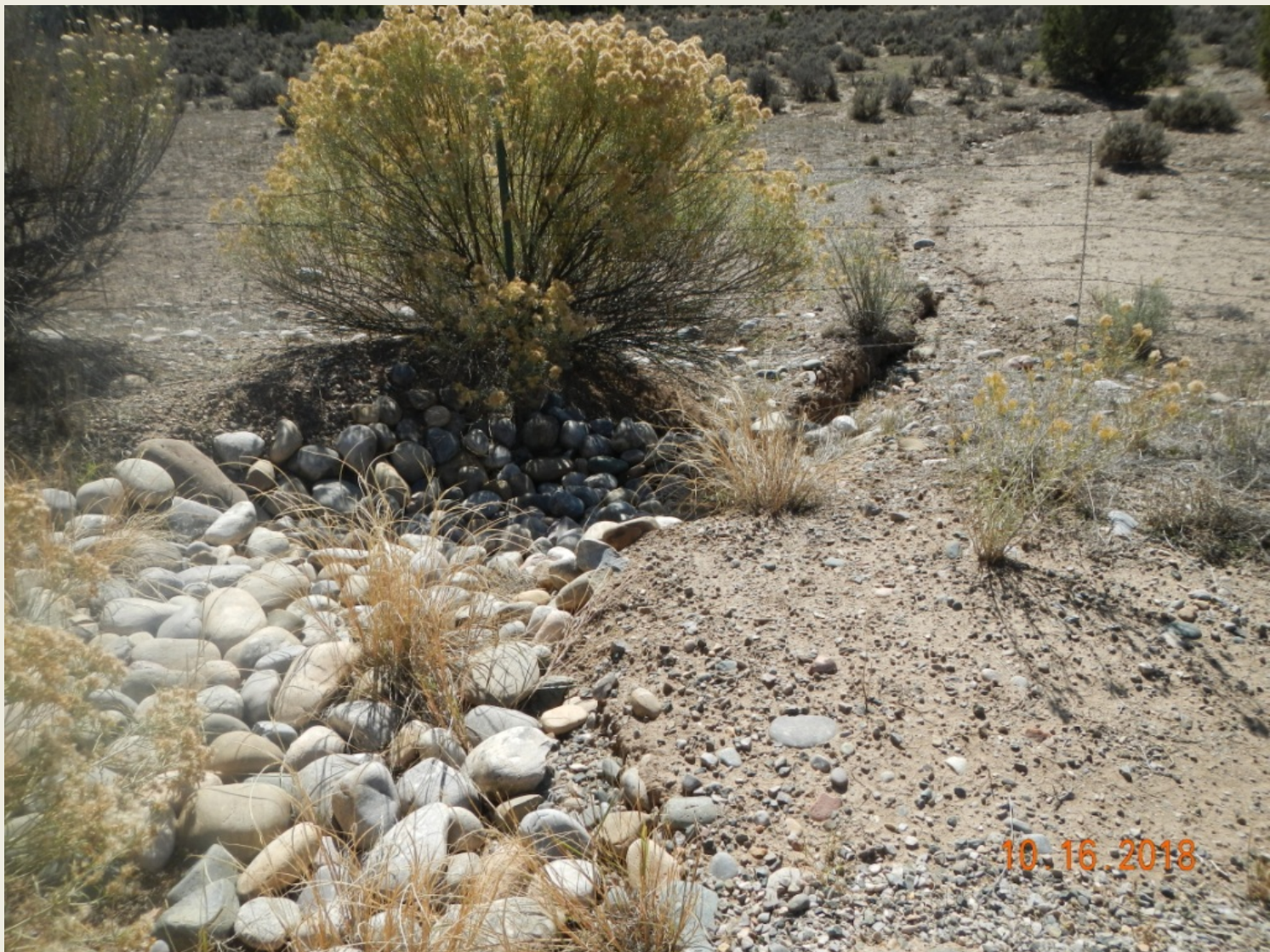
Photo 5. View of cobble run-down within the southern project area. Appears to be installed after formation of erosional channel. This needs to be monitored.
