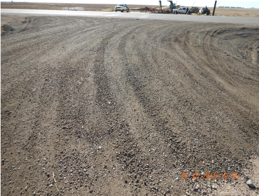
Photo 1. Photo taken from the entrance of location off Highway 14, facing South. Operator has installed a culvert along the roadside ditch and gravel at the entrance.
