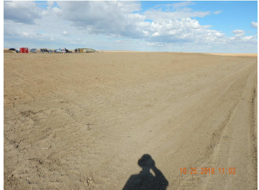
Photo 4. Photo taken from the northeastern perimeter of the location, facing North. Photo illustrates the topsoil stockpile which has been temporarily stabilized with equipment tracking.
