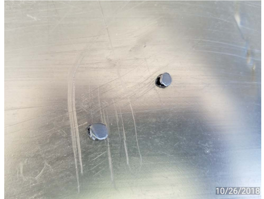
Holes in side of berm liner
