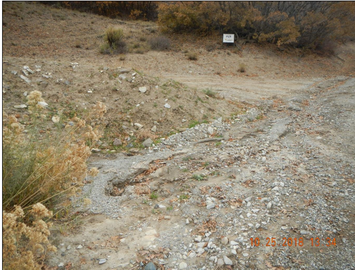
Sediment blockage in ditch at main and lease road intersection.
