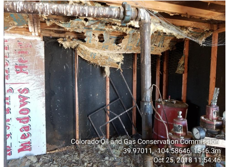
Photo 4 Ceiling falling down on equipment and trash
