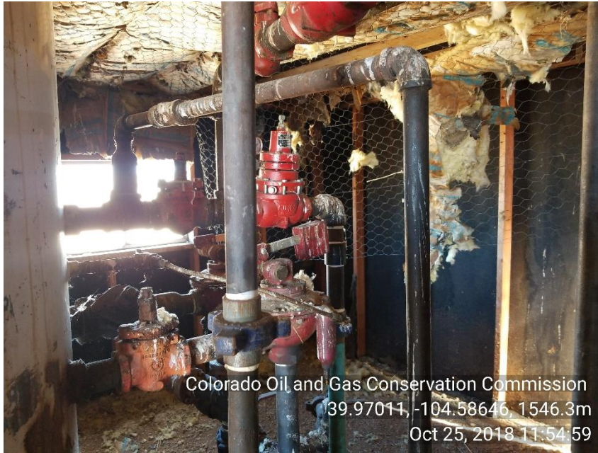
Photo 5 Ceiling falling down and trash on equipment
