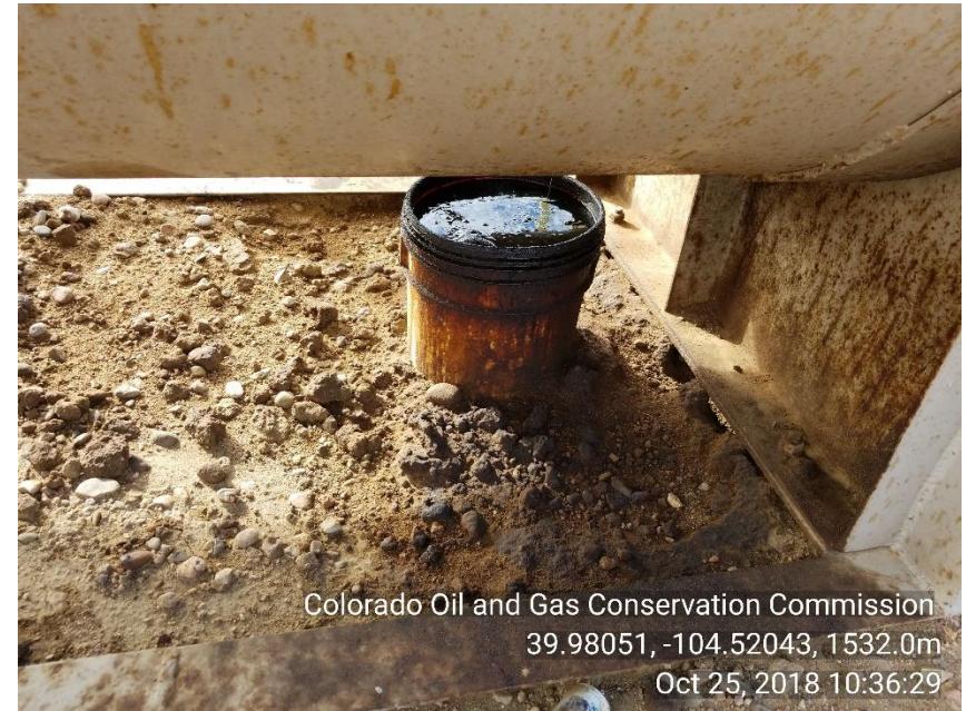
Photo 4 Stained soil under sep
