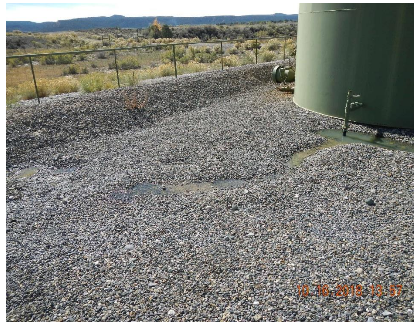
Fluid observed in secondary containment berm. Reportedly storm water.
