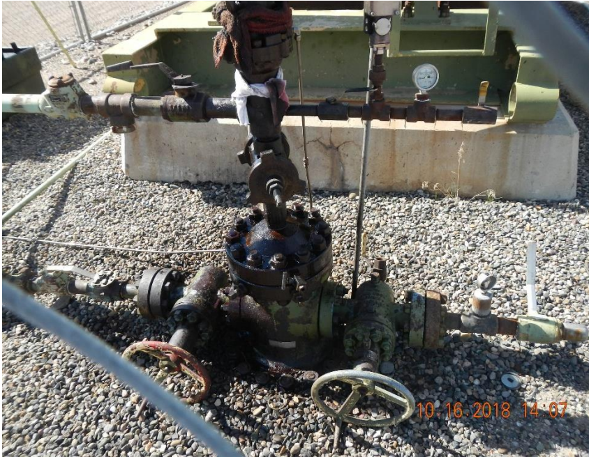
Well head is wet and stained.
