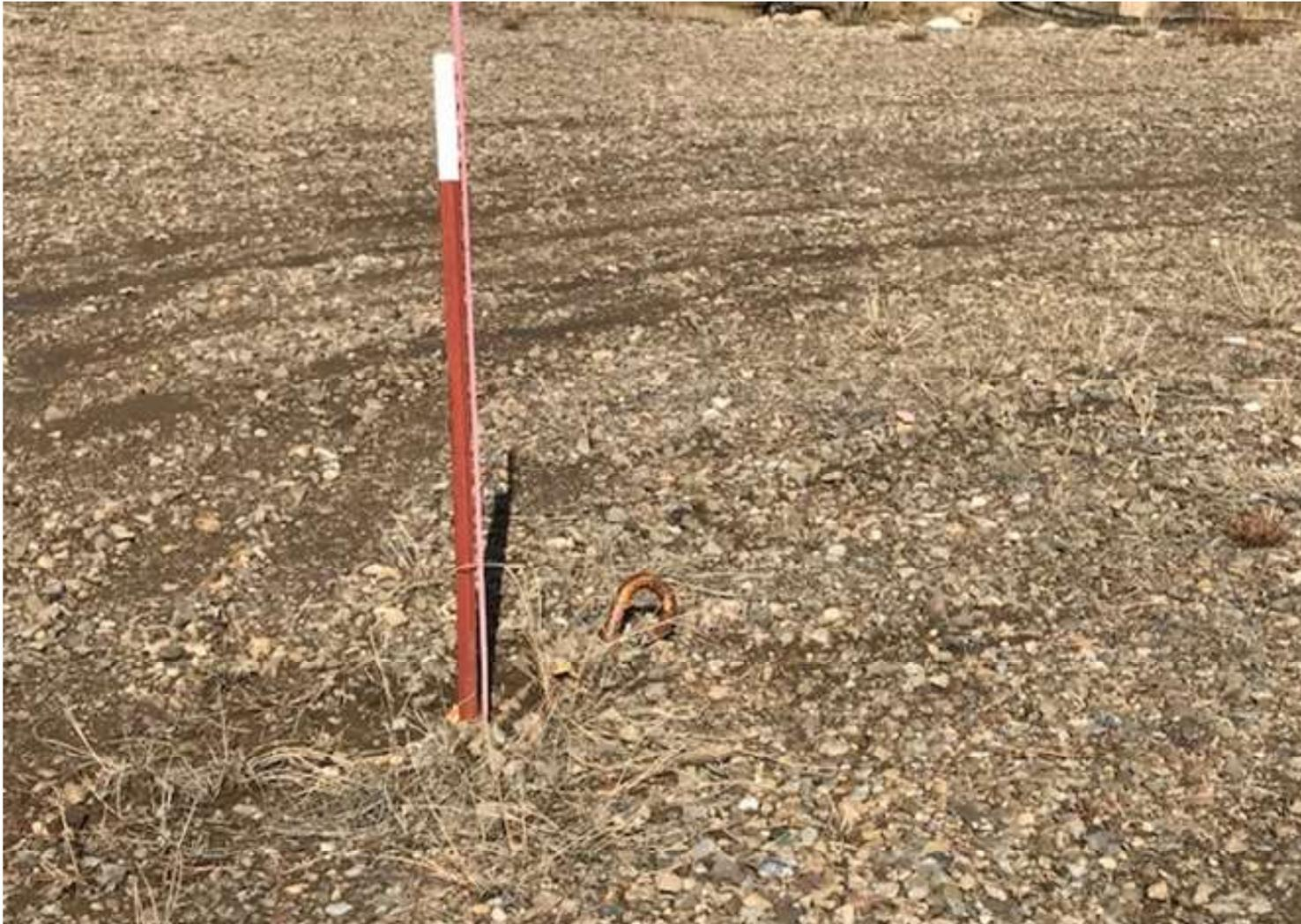
A NEW MARKER WAS INSTALLED ON THE UNMARKED DEADMAN ANCHOR IN COMPLIANCE WITH RULE 604.c.Q.
