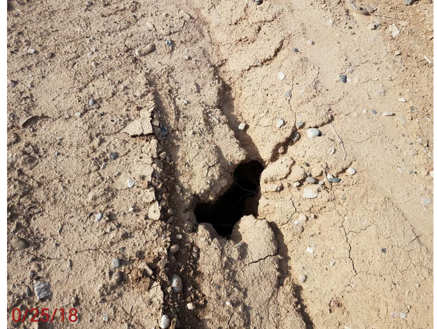
Location Photo #4, Storm water draining into holes along the ditch.
