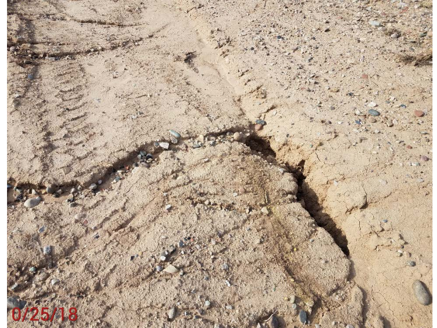
Location Photo #6, Storm water draining into holes along the ditch.
