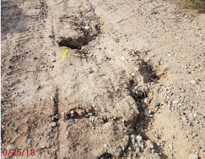
Location Photo #3, Storm water draining into holes along the ditch.
