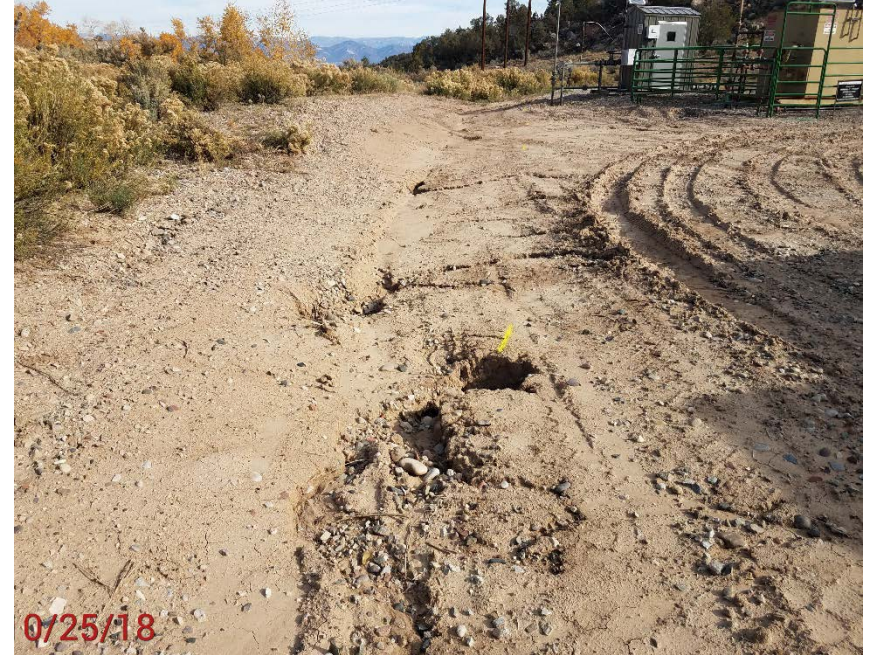
Location Photo #2, Storm water draining into holes along the ditch.
