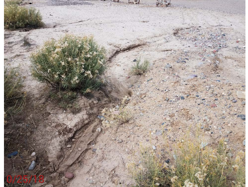
Location Photo #3, Sediment being moved off location, Repair with BMP's
