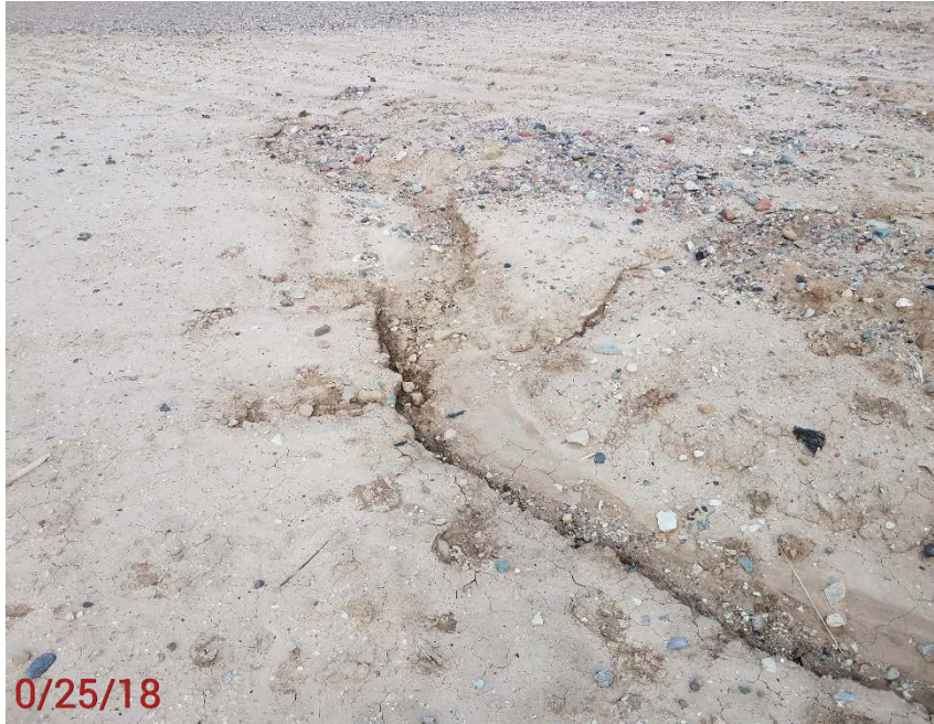
Location Photo #3, Sediment being moved off location, Repair with BMP's
