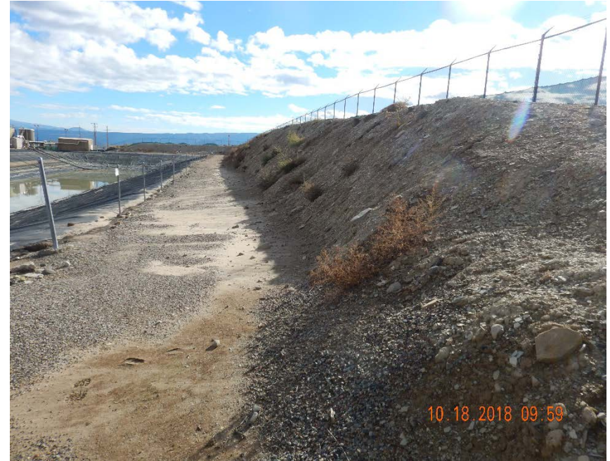
Photo #12 – View of earthen berm along south and southeast sides of facility. Note visible sediment transport from berm approaching Pit Facility #435835.
