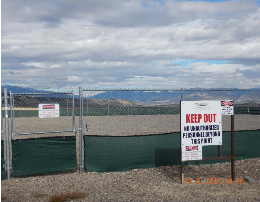
Photo #15 – Chain link fence with wildlife mesh and controlled entry at Pit Facility #433571.
