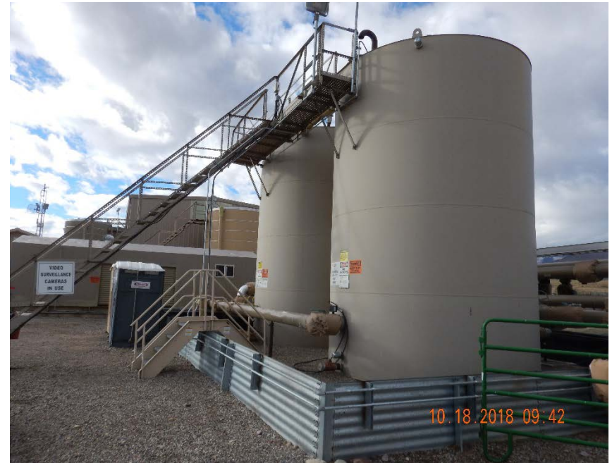
Photo #2 – View of 500 bbl produced water ASTs from northeast corner of SPCC.
