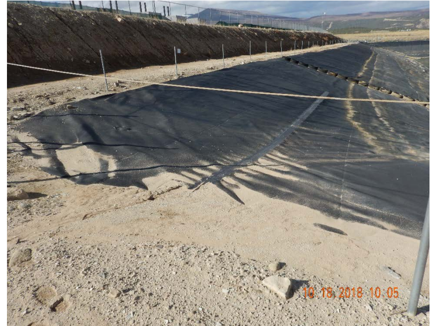
Photo #14 – Sediment transport into Pit Facility #435835 from east side.
