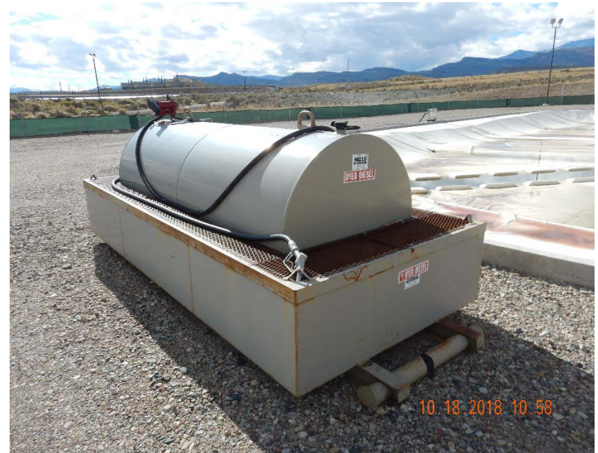
Photo #18 – Diesel tank with secondary containment located at SE corner of Pit Facility #433571.
