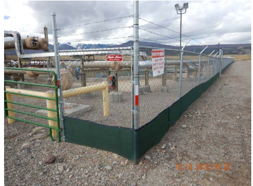
Photo #8 – View of fence surrounding pit complex from NE corner. Note chain link fence with barbed wire on north side of pit complex (right side of photo) joins with steel panel fence on east side of pit complex (left side of photo).
