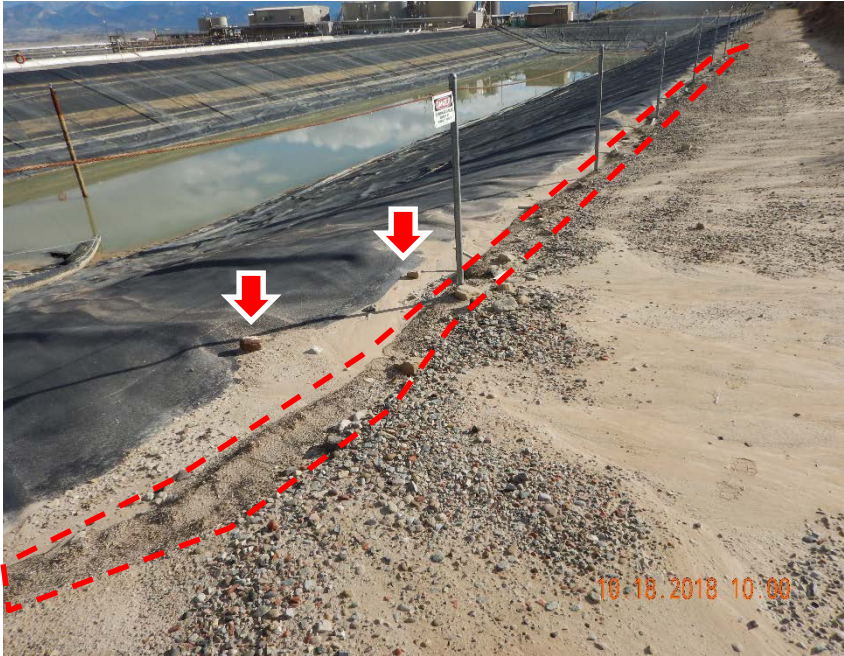
Photo #13 – Straw wattle along south side of Pit Facility #435835 (red outline) needs repair or replacement. Note evidence of sediment transport and rocks (red arrows) on top of pit liner.
