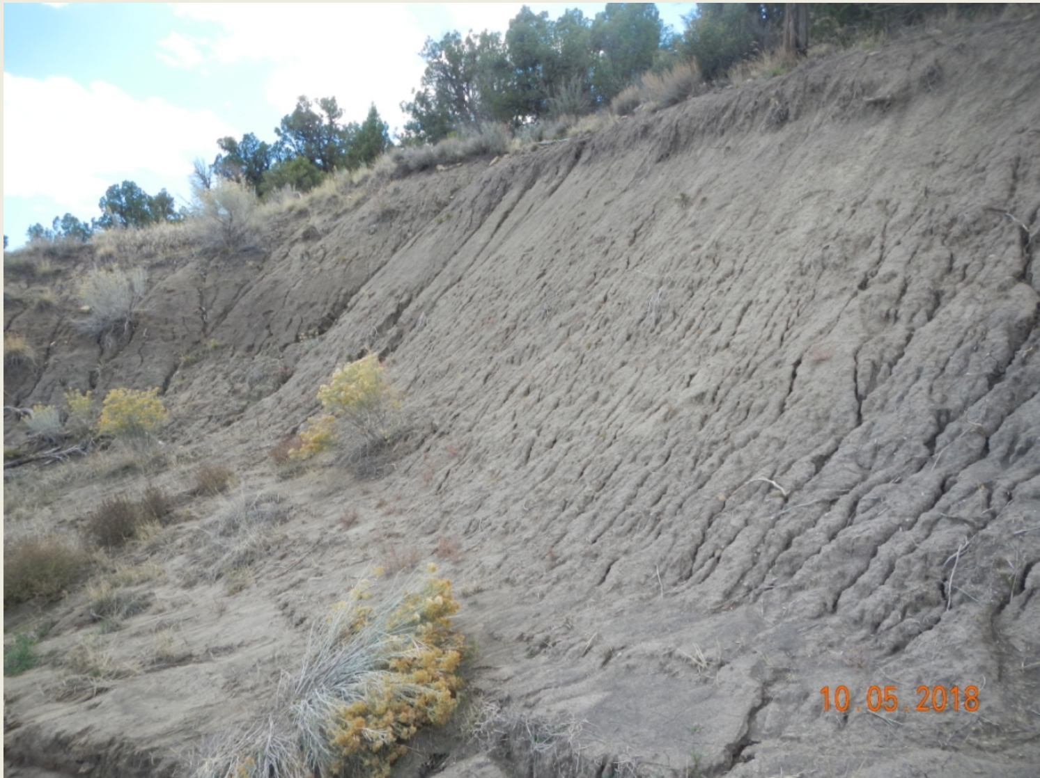
Photo 4. View of the southwestern portion of the project area. Erosional channels and deep rills are forming within the cut-slope. Exposed roots are visible.
