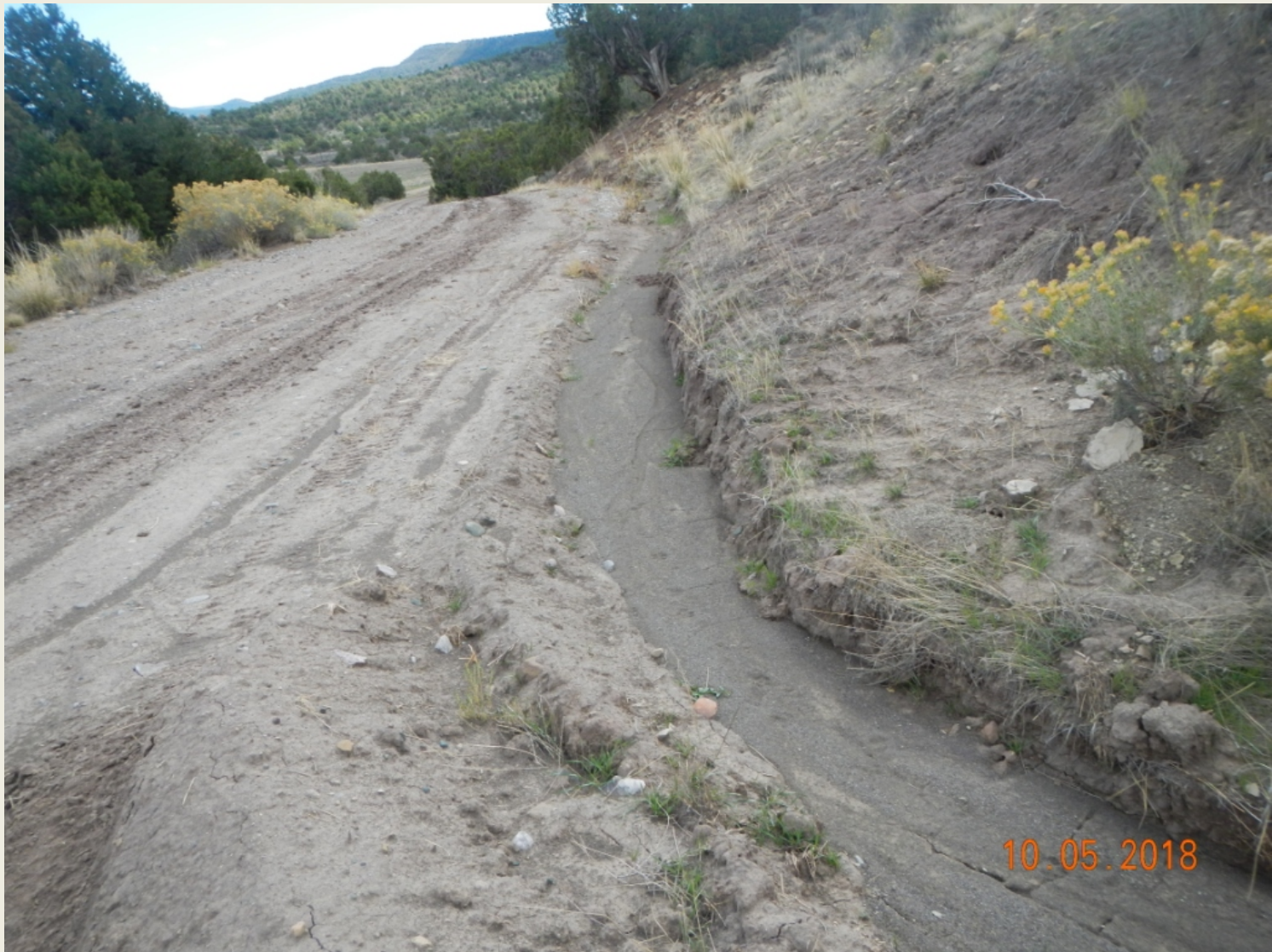
Photo 6. View of diversion ditch from western and southwestern cut-slope, full of sediment and not properly stabilized.
