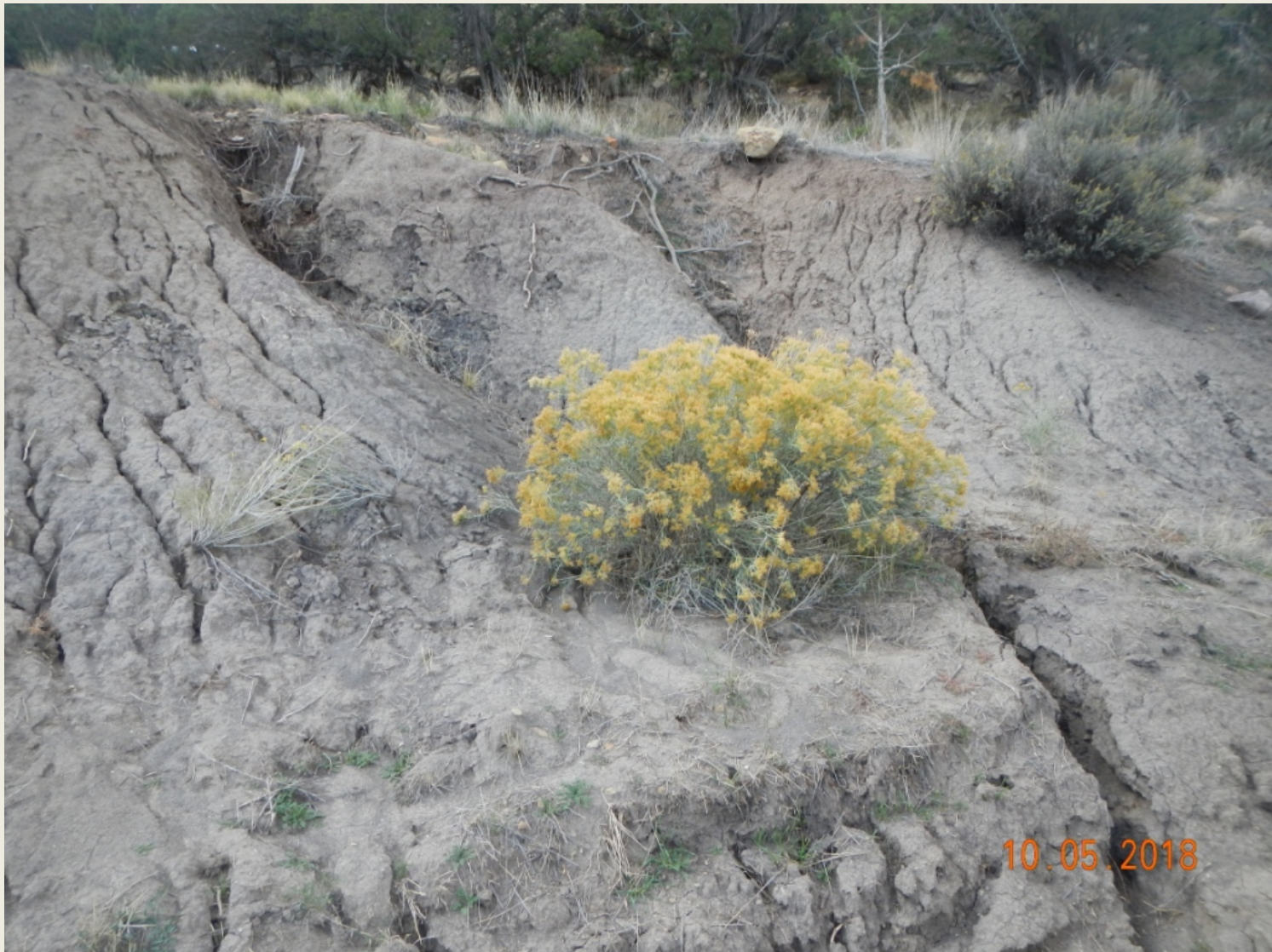
Photo 5. View of erosional channels in the southwestern cut-slope, approximately 2 to 3 feet wide and deep.
