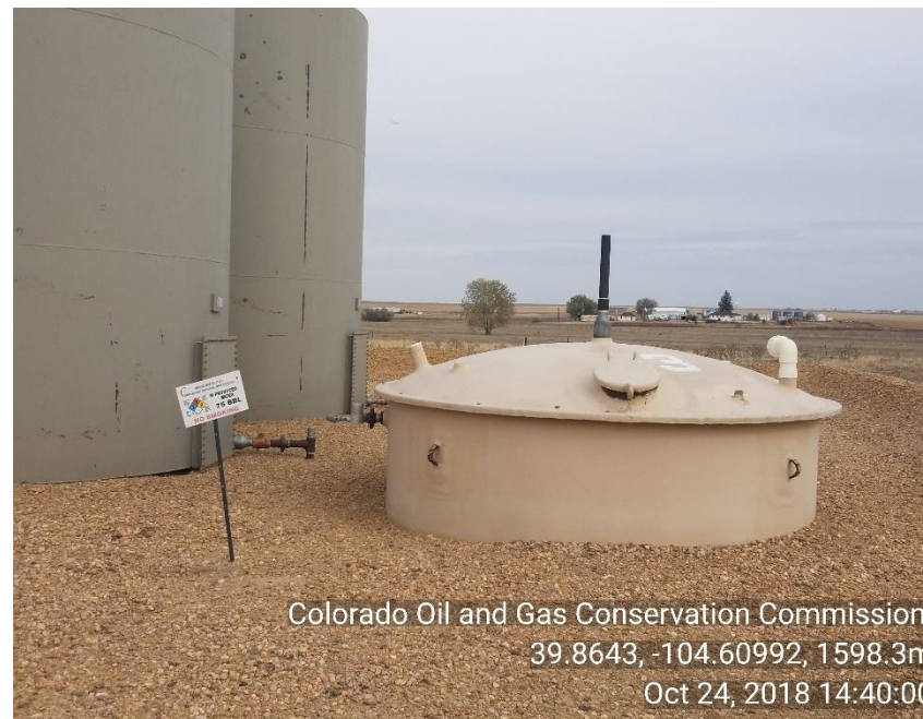
Photo 2 Produced water tank
