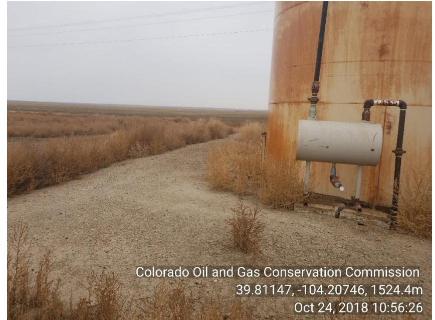
Phot 6 no berm around crude oil tank
