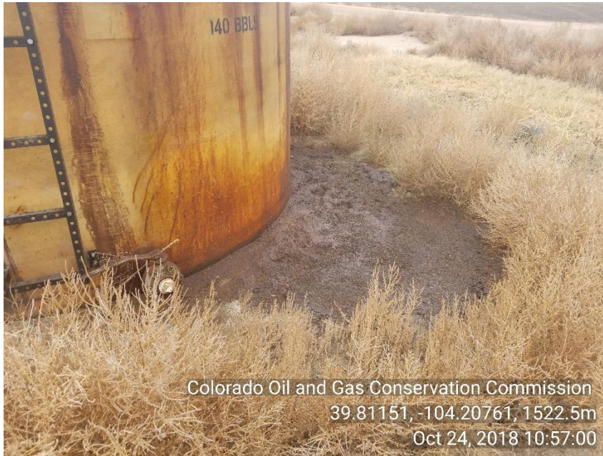
Photo 7 Stained soil around Pro water fiberglass tank
