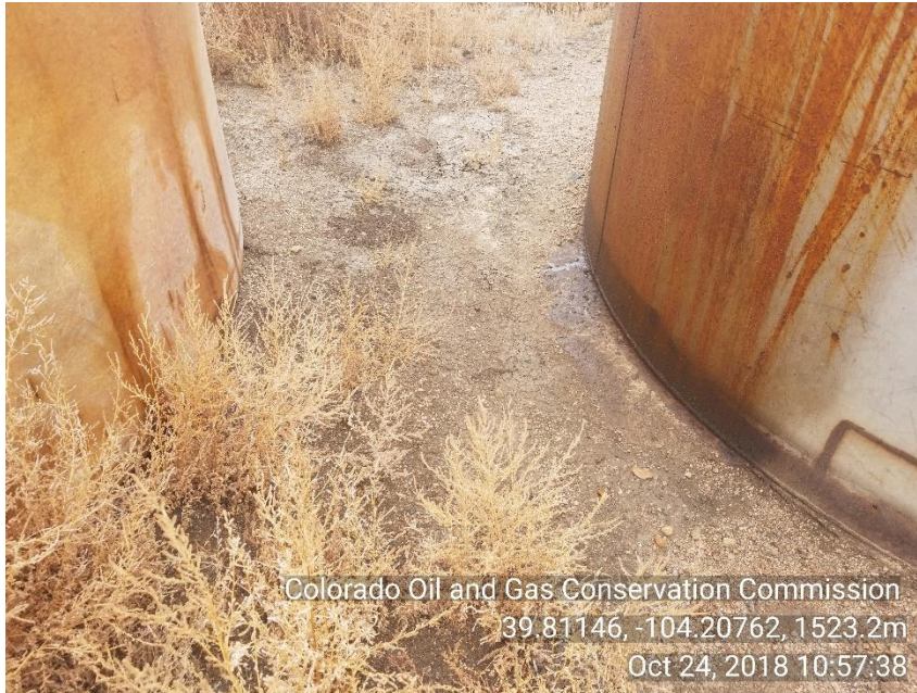
Photo 9 Stained soil around Produced water steel tank
