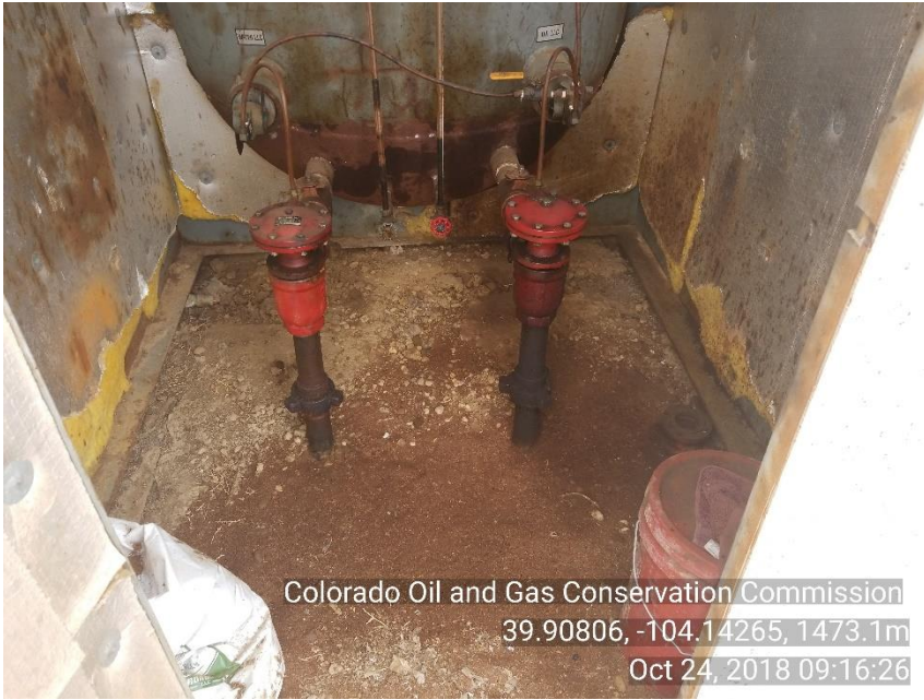
Photo 5 Stained soil in side sep house
