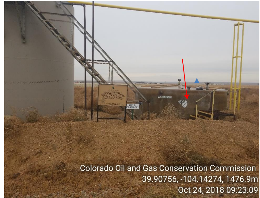
Photo 2 TNK BTRY Pro tank faded placards and no volume sign
