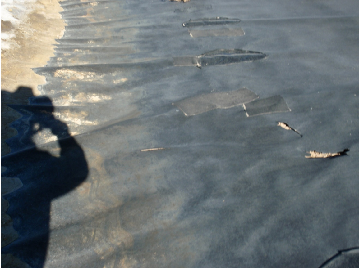
Photo 75. Damage to liner along north side of pit
