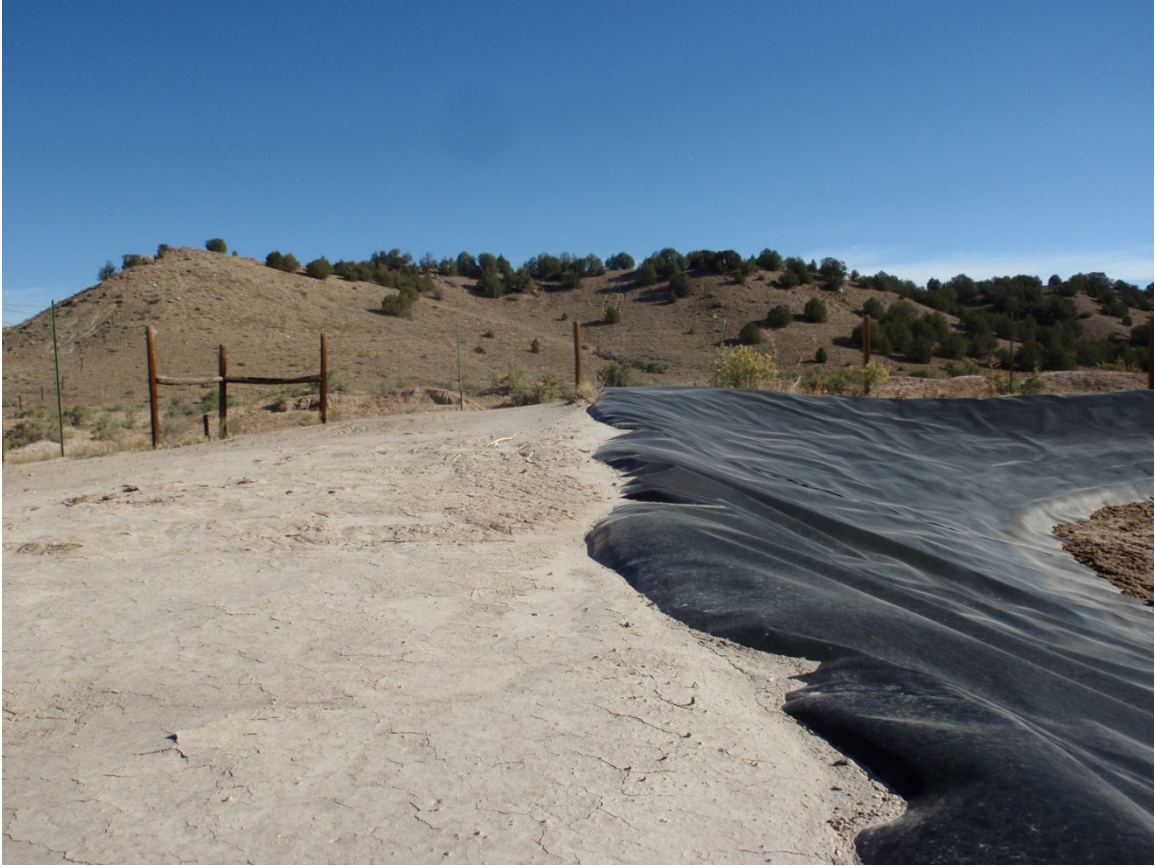
Photo 49. Erosion on northwest corner of pit
