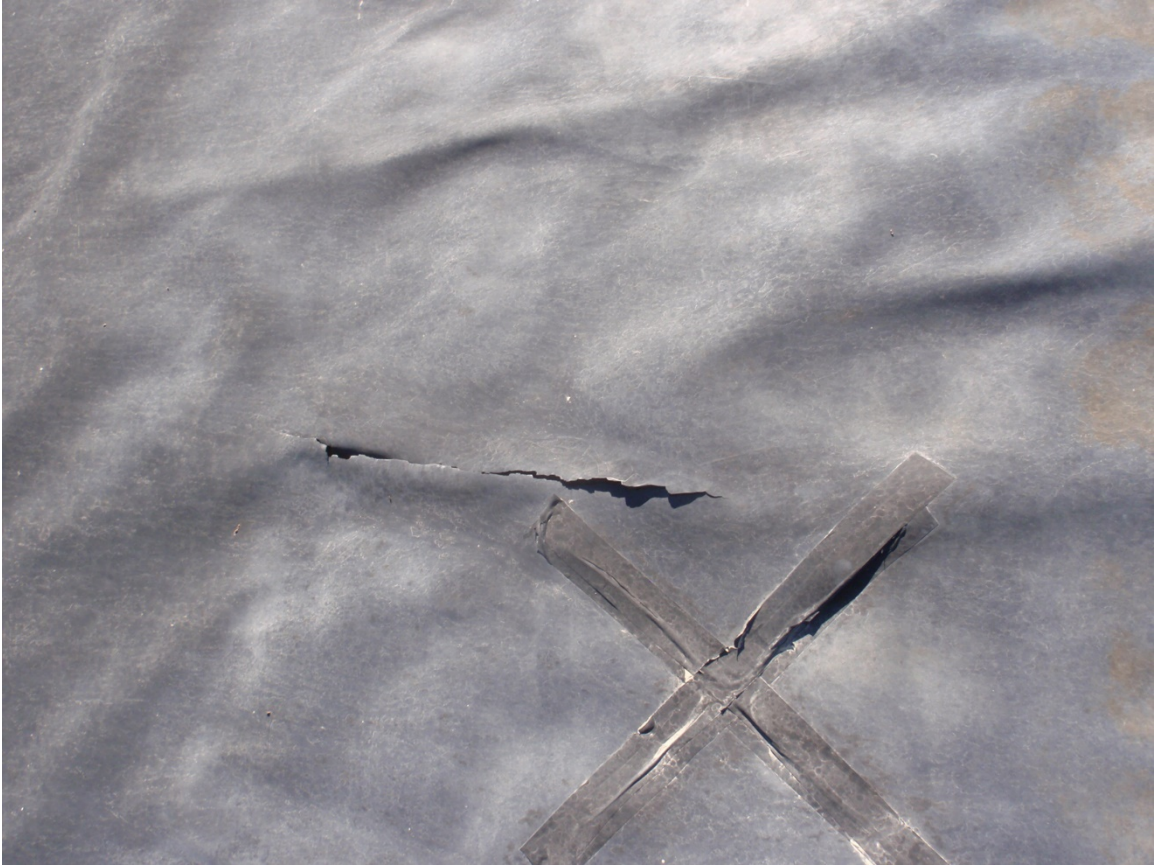
Photo 63. Damage to liner along north side of pit
