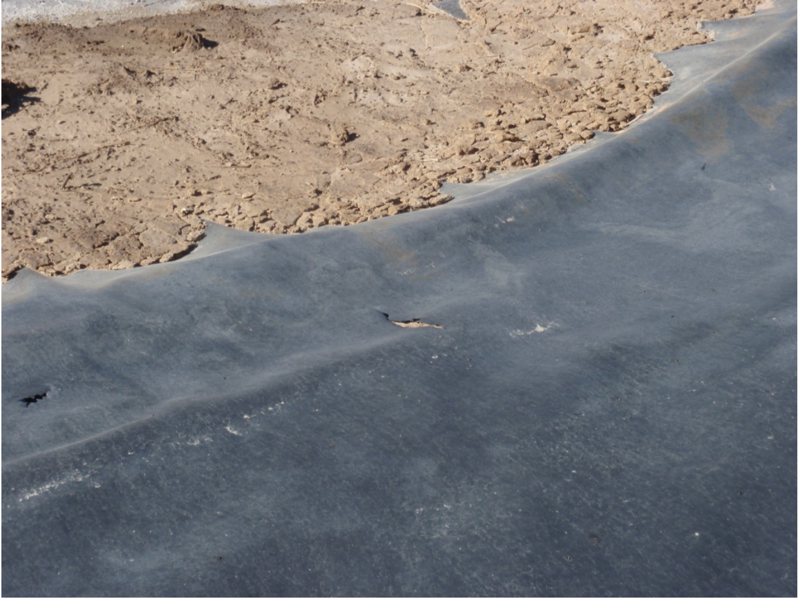
Photo 53. Damage to liner along north side of pit
