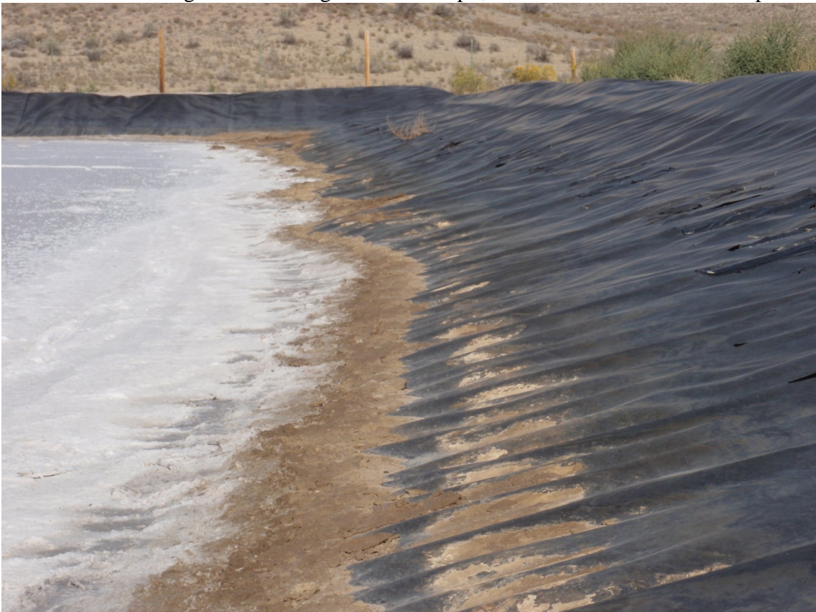
Photo 83. Damage to liner along north side of pit, accumulation of sediment in pit
