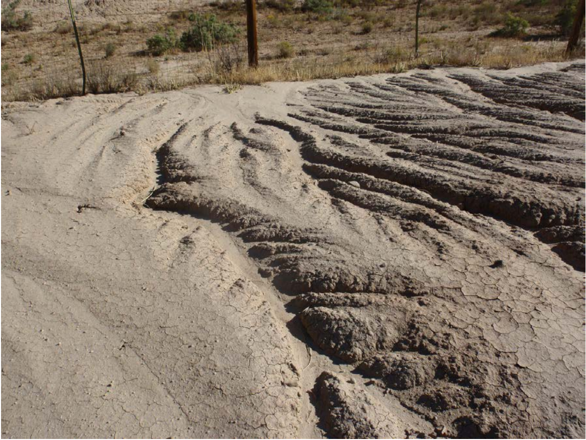
Photo 51. Erosional rills along the north side of pit.
