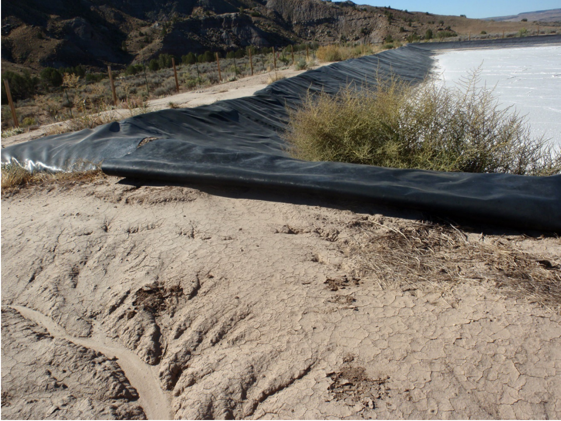
Photo 96. Damage to liner and erosion issues at northeast corner of pit.
