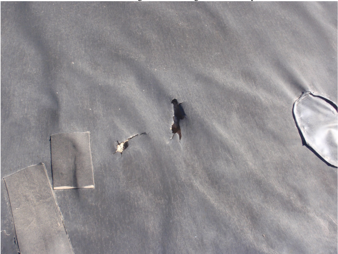
Photo 72. Damage to liner along north side of pit
