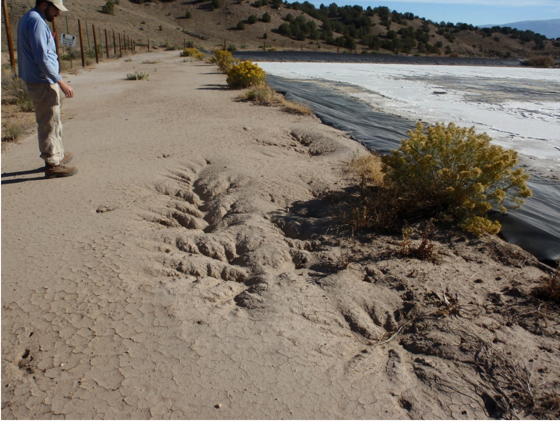
Photo 41. Erosion on berm on west side of pit
