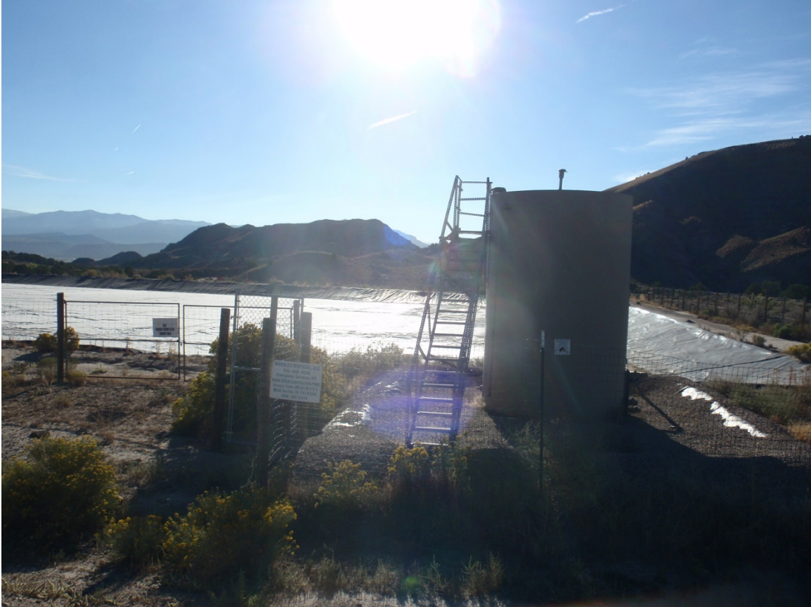
Photo 5. 300 barrel storage tank with shallow berm. Can it hold 115% capacity of liquid?
