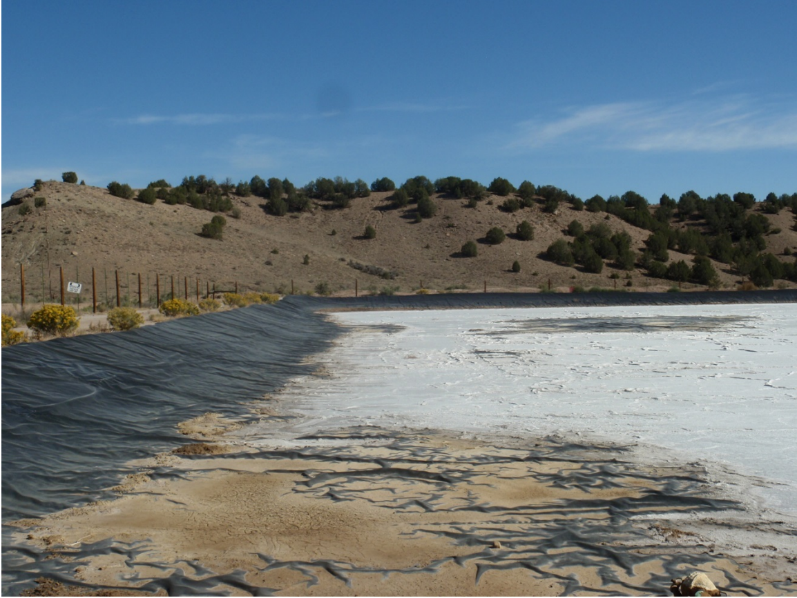
Photo 112. Accumulation of sediment in southwest corner of pit.
