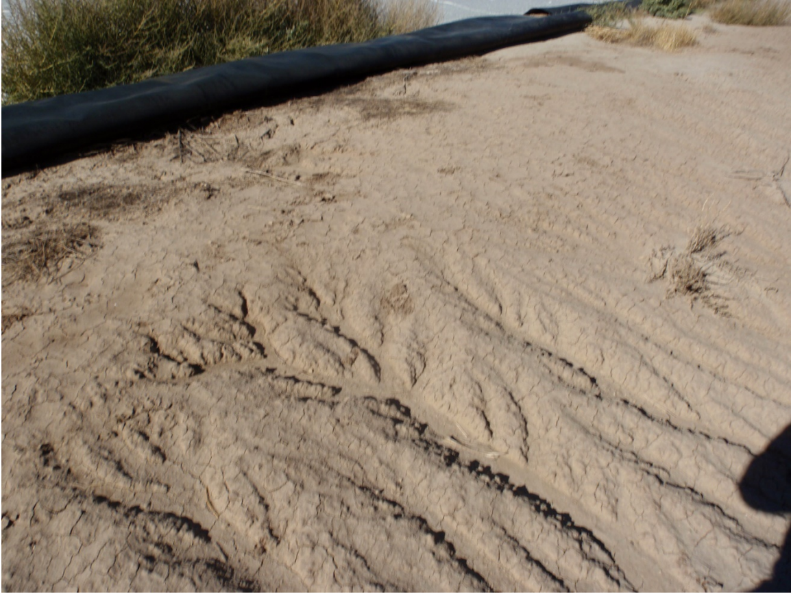
Photo 98. Damage to liner and erosion issues at northeast corner of pit.
