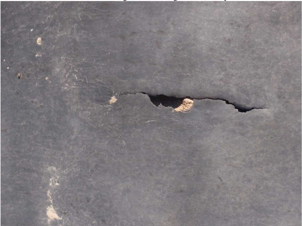
Photo 58. Damage to liner along north side of pit
