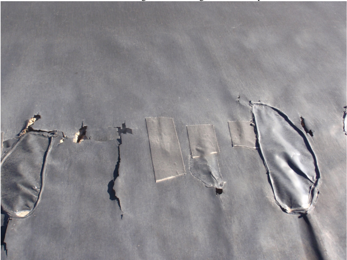
Photo 80. Damage to liner along north side of pit
