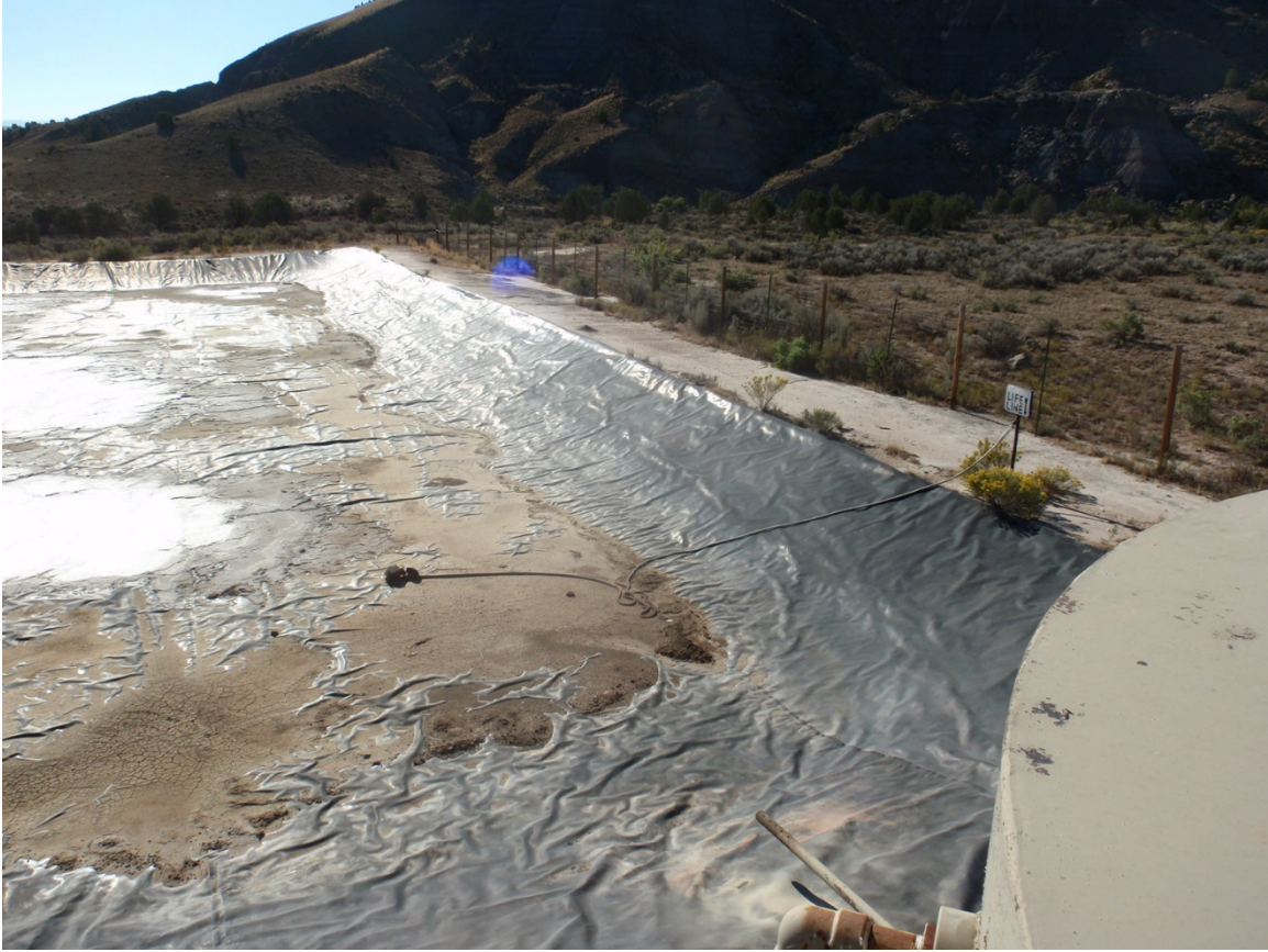
Photo 31. View of south side of pit, soil and salt accumulation in pit.
