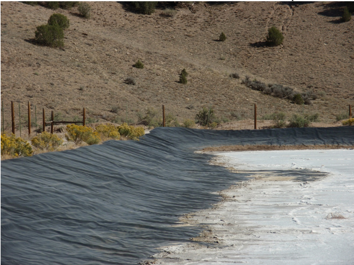
Photo 113. Accumulation of sediment in west side of pit.
