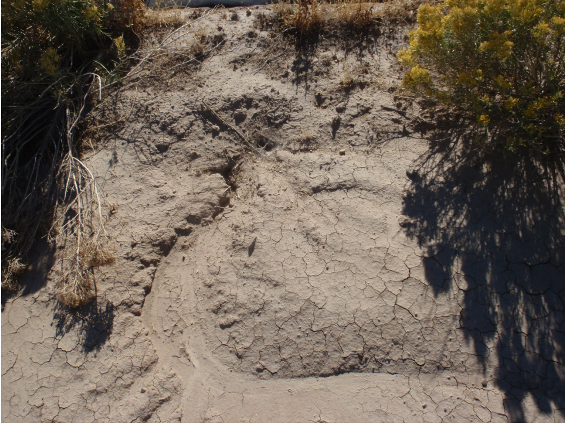
Photo 47. Erosional rill at northwest corner of pit soil migrating under liner.
