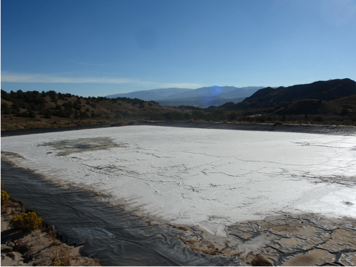
Photo 33. View of central part of pit, soil and salt accumulation in pit.
