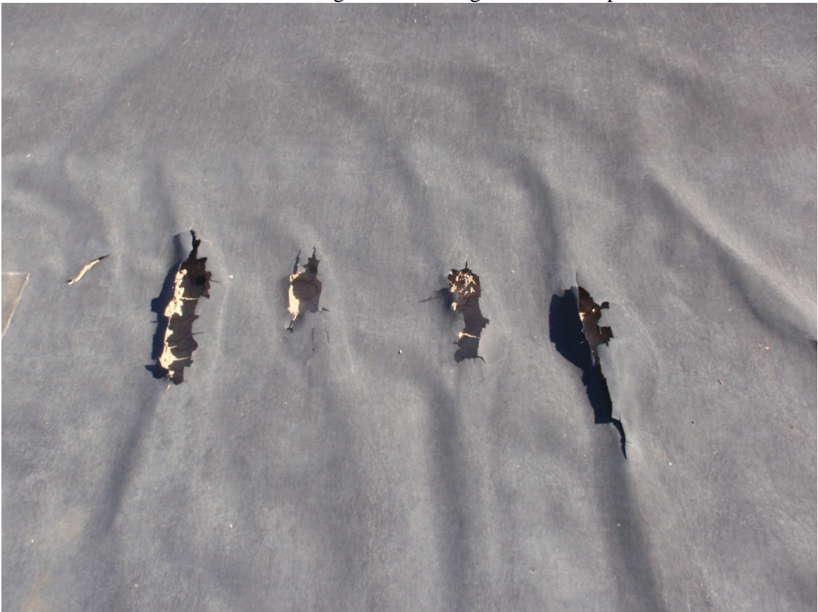
Photo 66. Damage to liner along north side of pit
