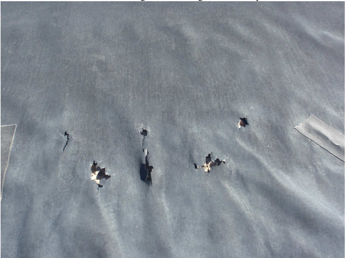
Photo 76. Damage to liner along north side of pit
