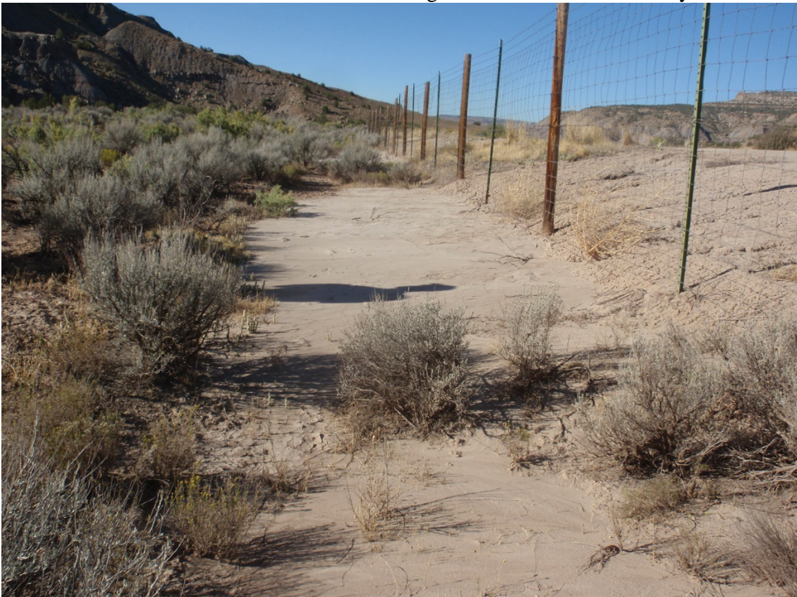
Photo 22. Erosion and offsite soil migration on east side of facility.
