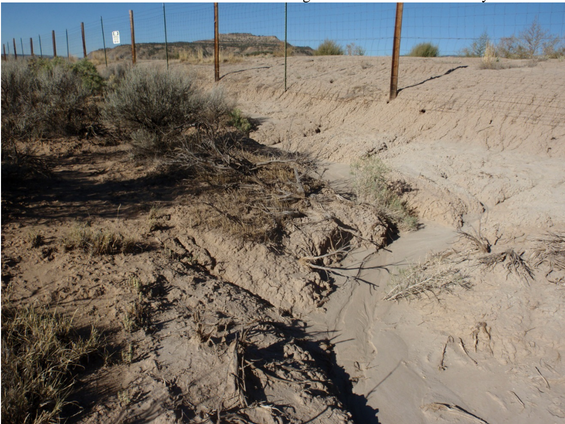
Photo 20. Erosion and offsite soil migration on east side of facility.
