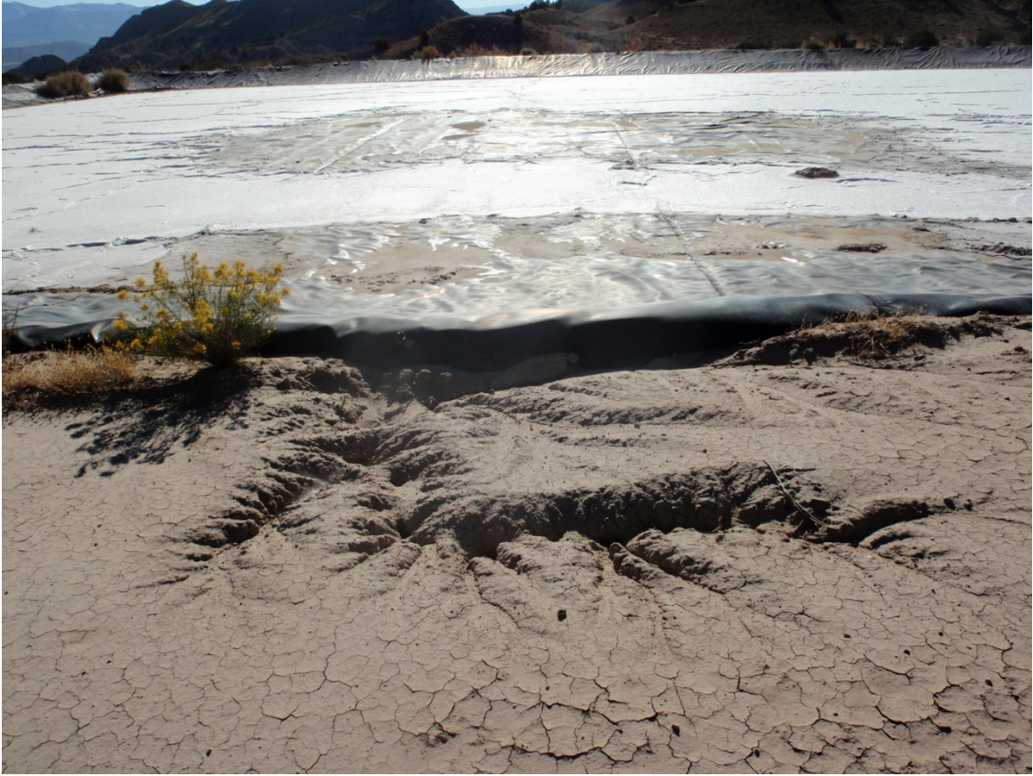
Photo 43. Erosion on berm on west side of pit
