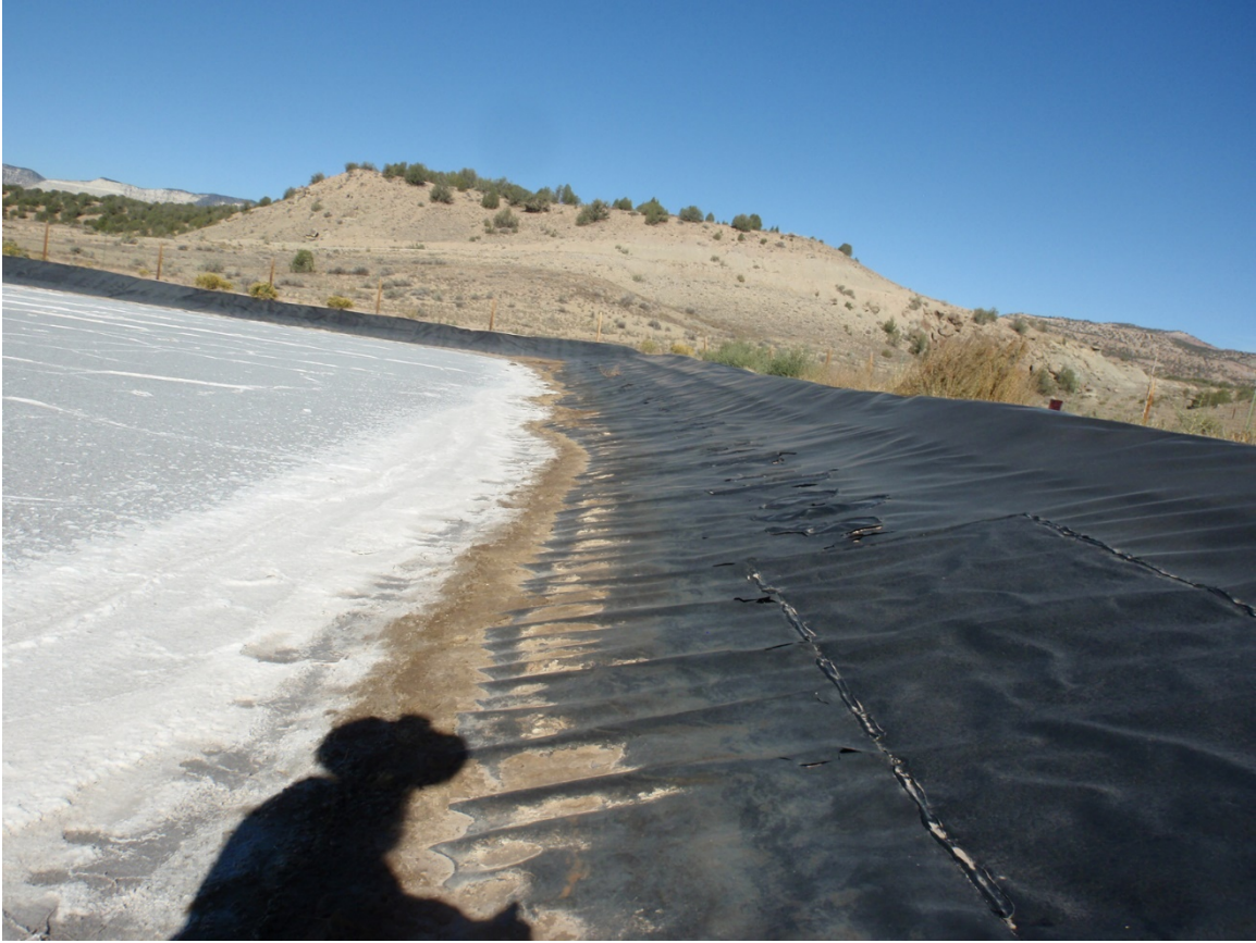
Photo 82. Damage to liner along north side of pit, accumulation of sediment in pit
