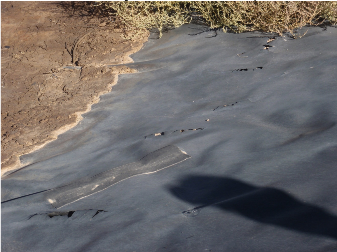
Photo 89. Damage to liner at northeast corner of pit.
