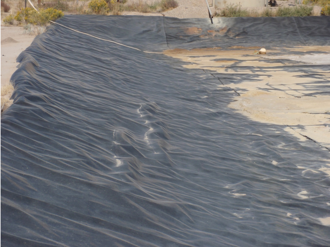
Photo 110. View of liner on south side of pit looking west. Two small rills under liner?
