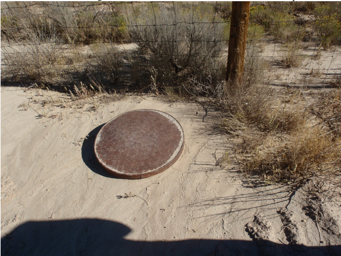
Photo 99. Cover to leak detection system on north side of pit
