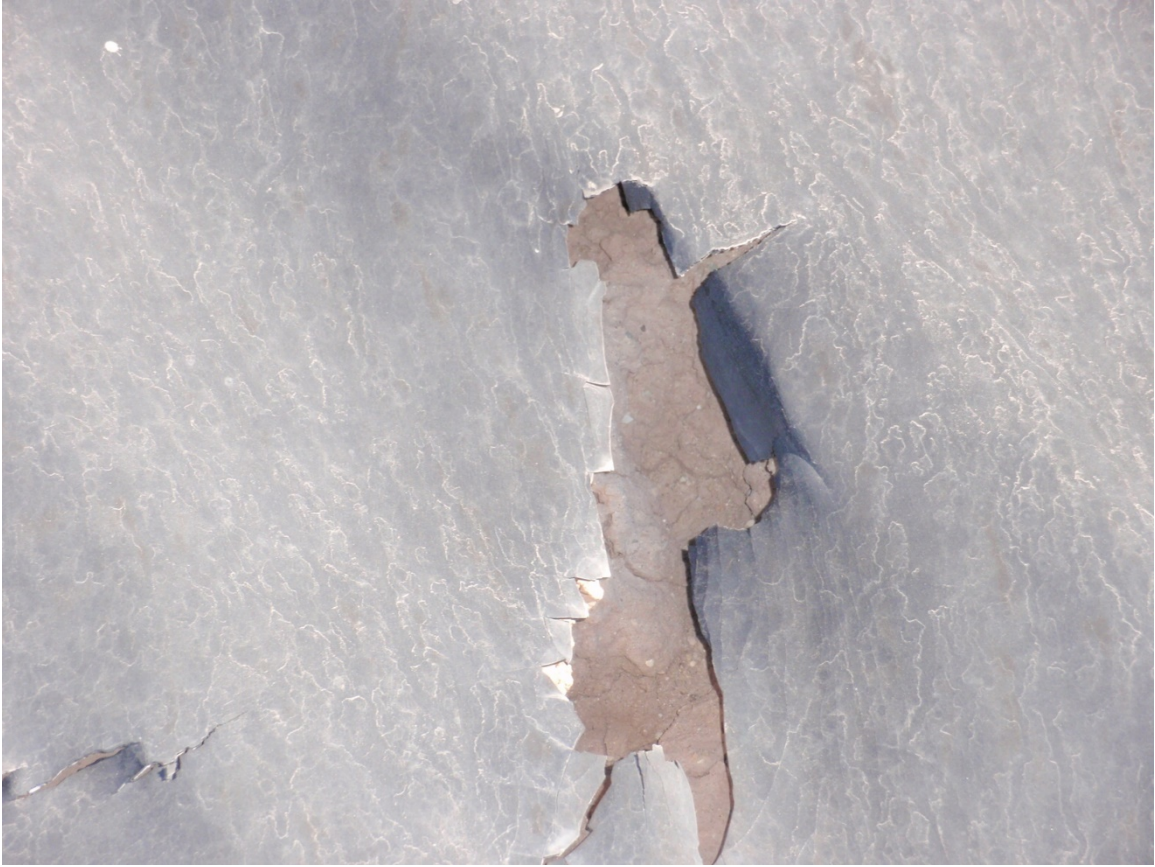
Photo 73. Damage to liner along north side of pit
