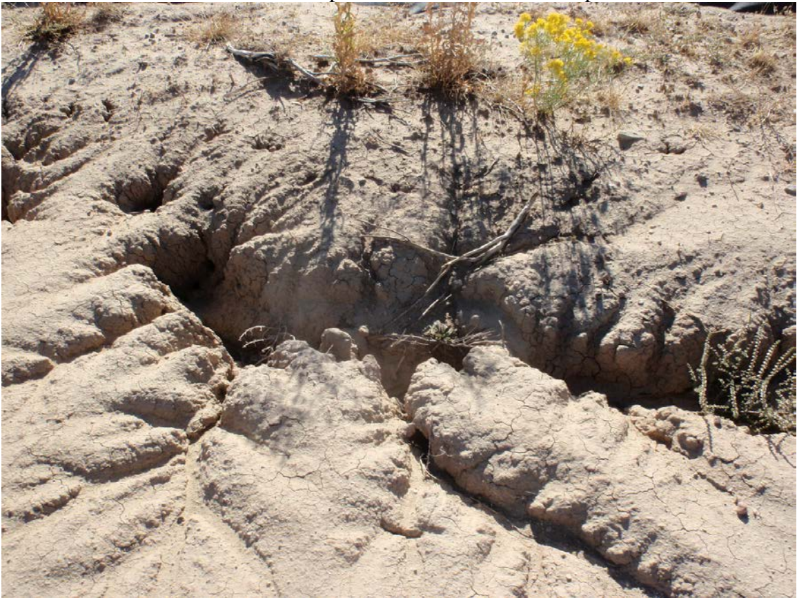
Photo 38. Erosion on berm on west side of pit
