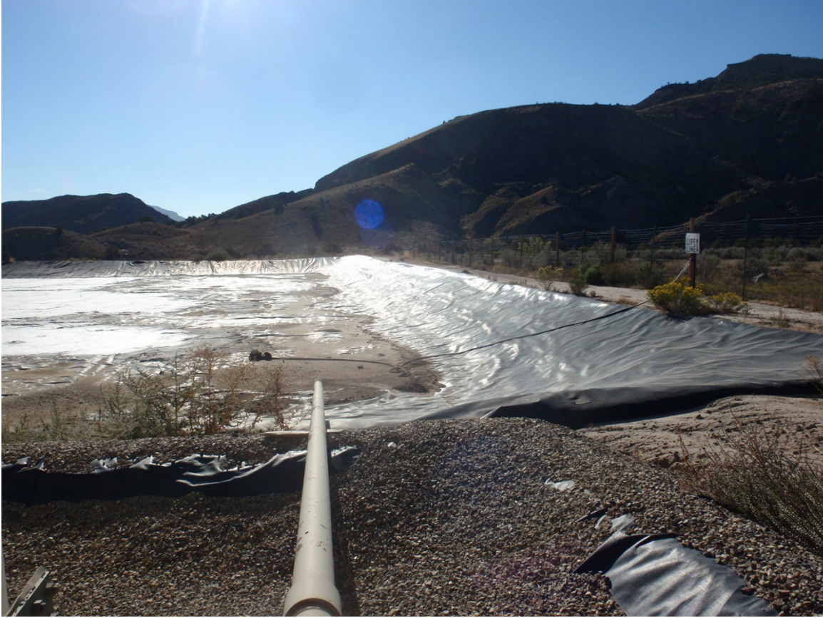
Photo 29. Tank outlet and lifeline in pit.
