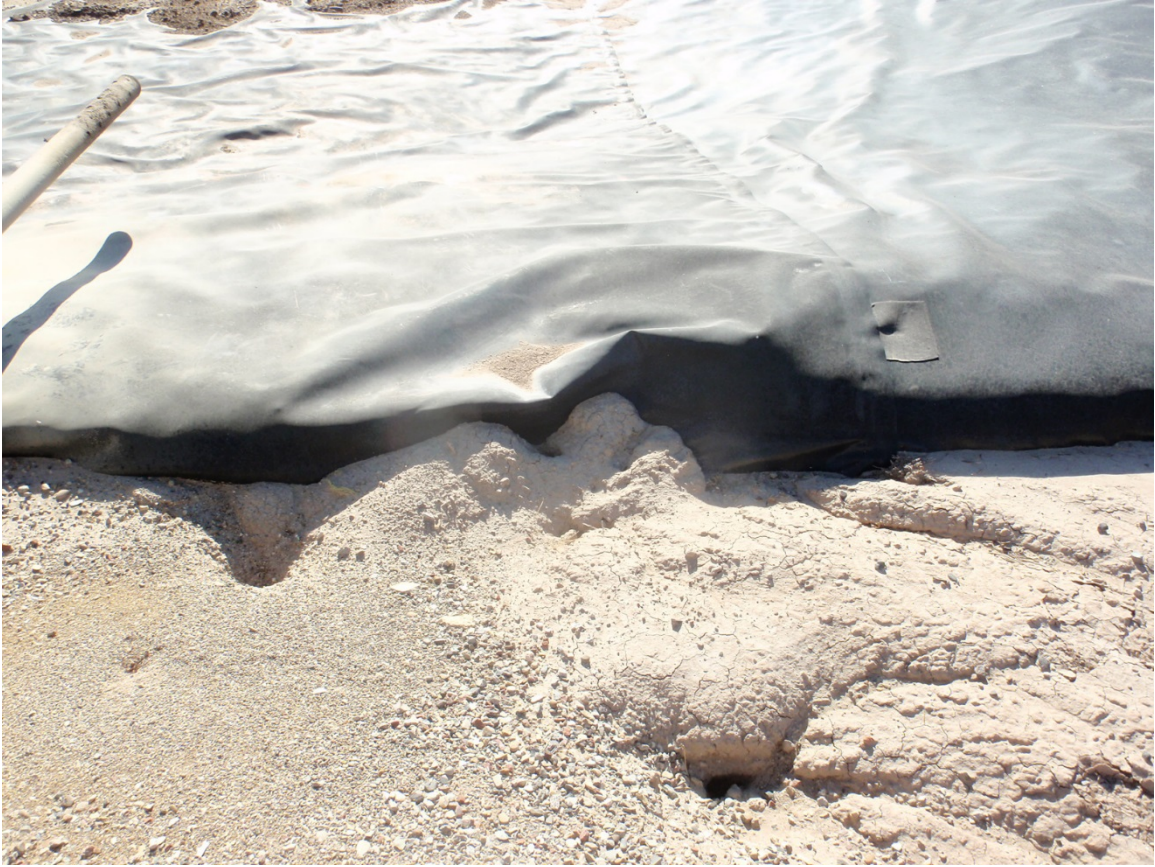
Photo 35. Erosion of soils under liner near tank liner not keyed into berm sufficiently.
