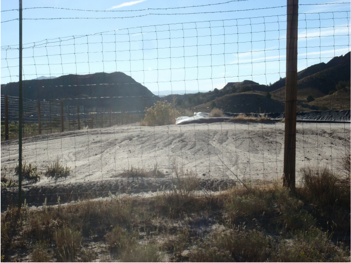
Photo 11. Northwest corner of pit. Berm eroding and soil piling up at bottom of fence
