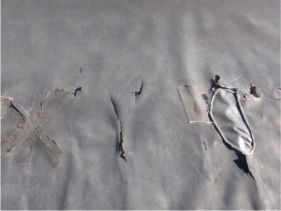
Photo 79. Damage to liner along north side of pit
