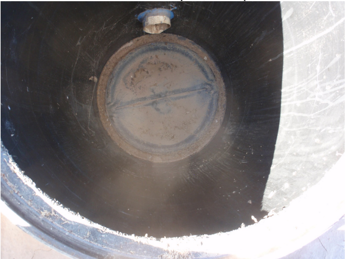
Photo 101. Leak detection system, no water present
