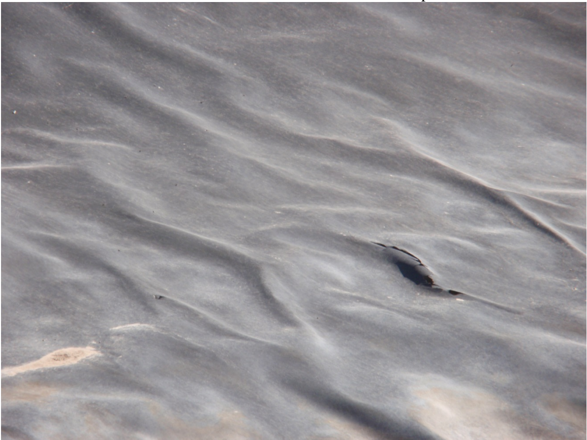
Photo 50. Visible crack in liner near northwest corner.
