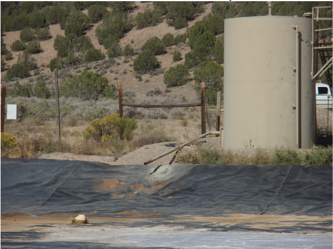
Photo 109. Erosion issue on berm next to 300 bbl tank
