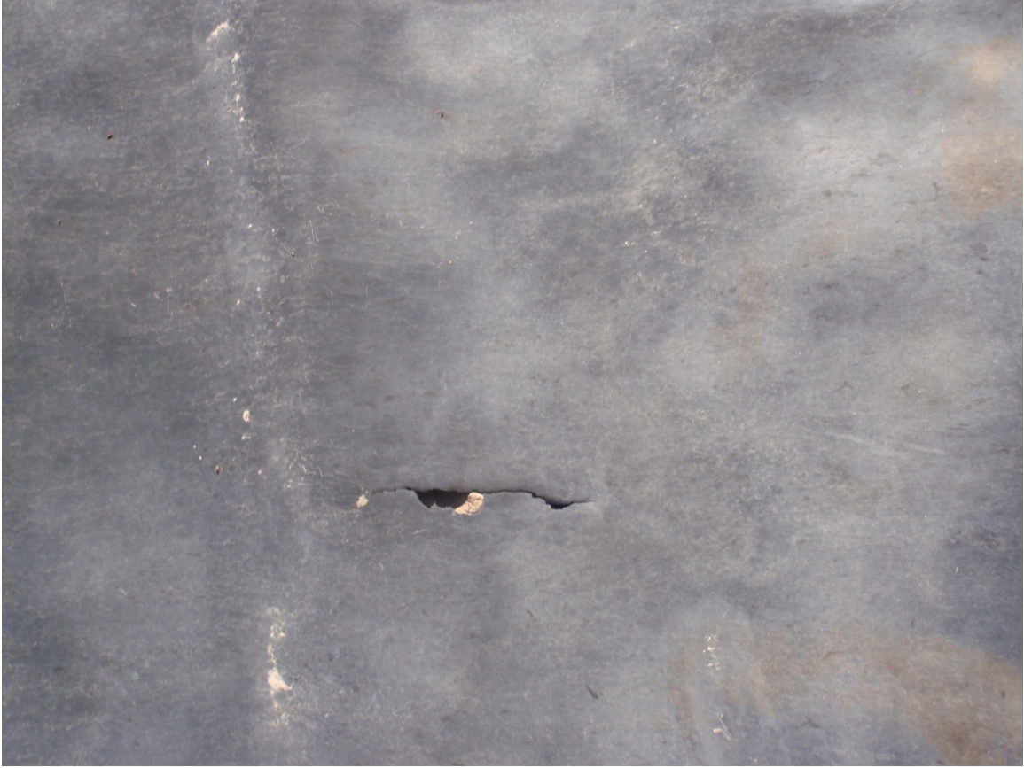
Photo 59. Damage to liner along north side of pit
