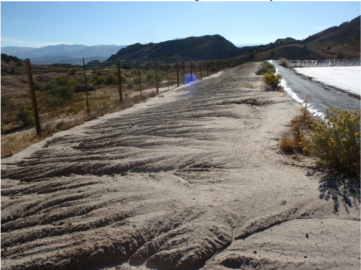
Photo 52. Erosional rills along the north side of pit.
