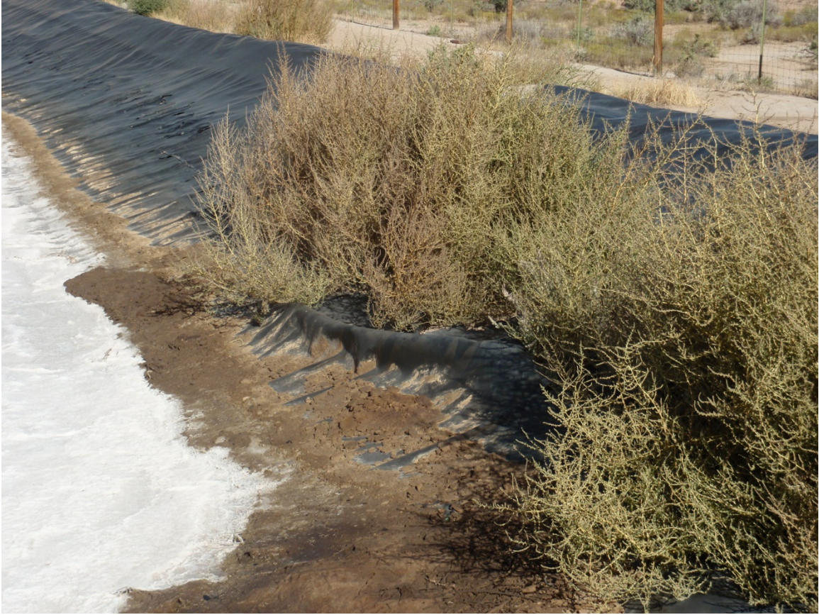
Photo 88. Large tear in liner at northeast side of pit
