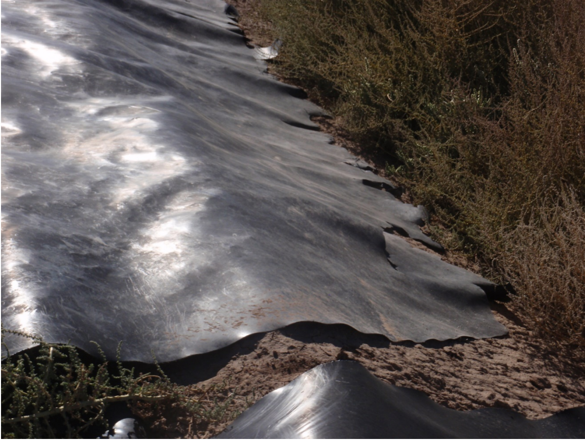
Photo 84. Large tear in liner at northeast side of pit.
