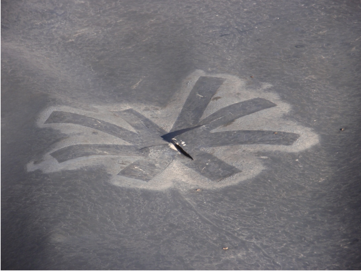
Photo 106. Damage to patch in liner near southeast corner
