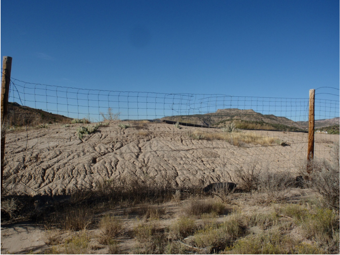
Photo 15. Erosional rills on north side of berm at facility. No vegetation to hold soil in place.
