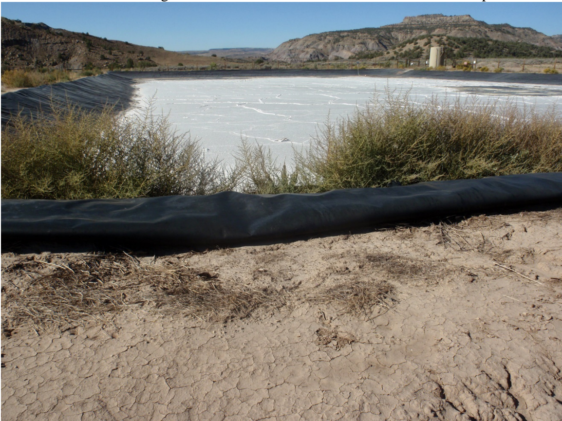
Photo 97. Damage to liner at northeast corner of the pit
