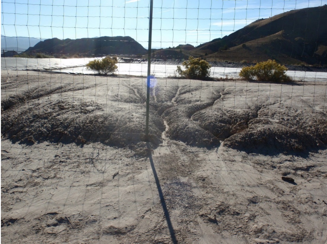
Photo 9. West side of facility berm showing erosional rills
