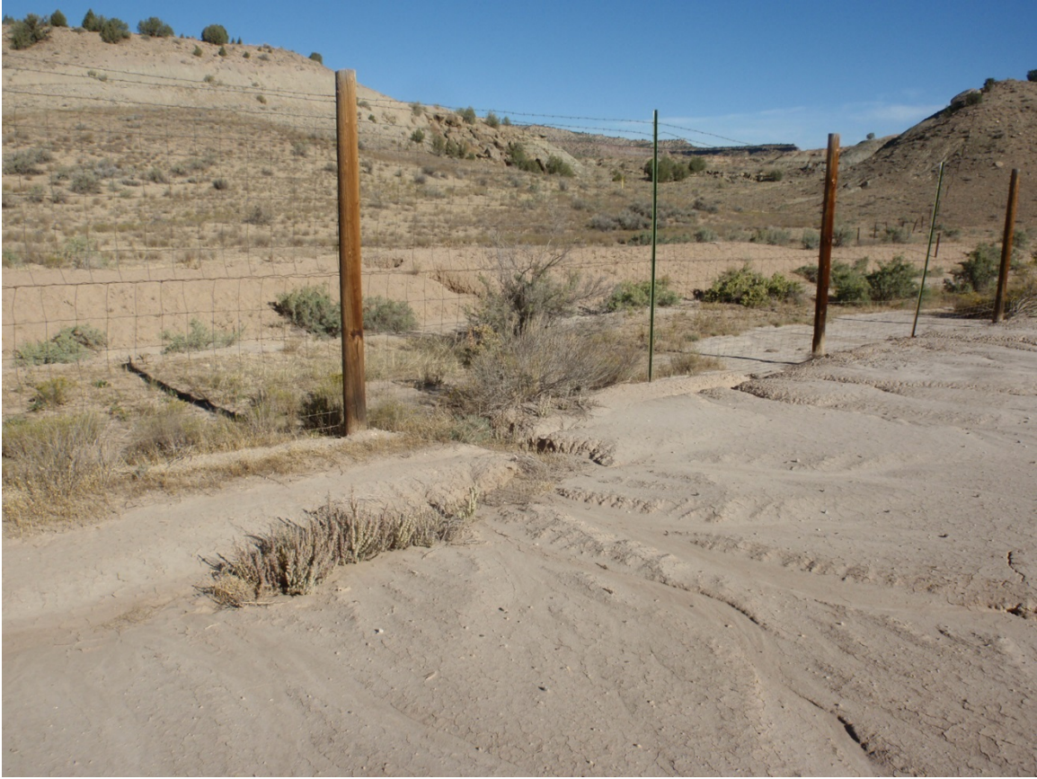
Photo 45. Erosion on berm on west side of pit, soil migrating offsite.
