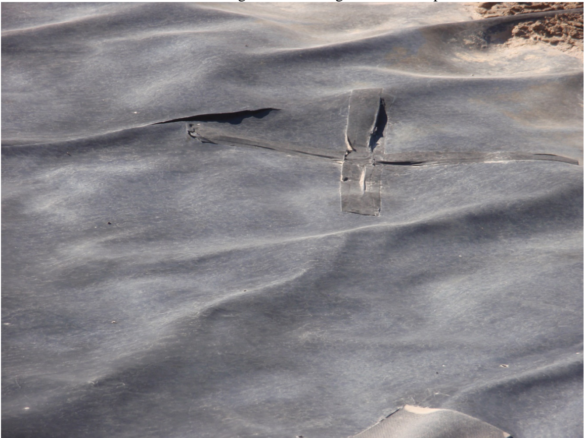
Photo 56. Damage to liner along north side of pit
