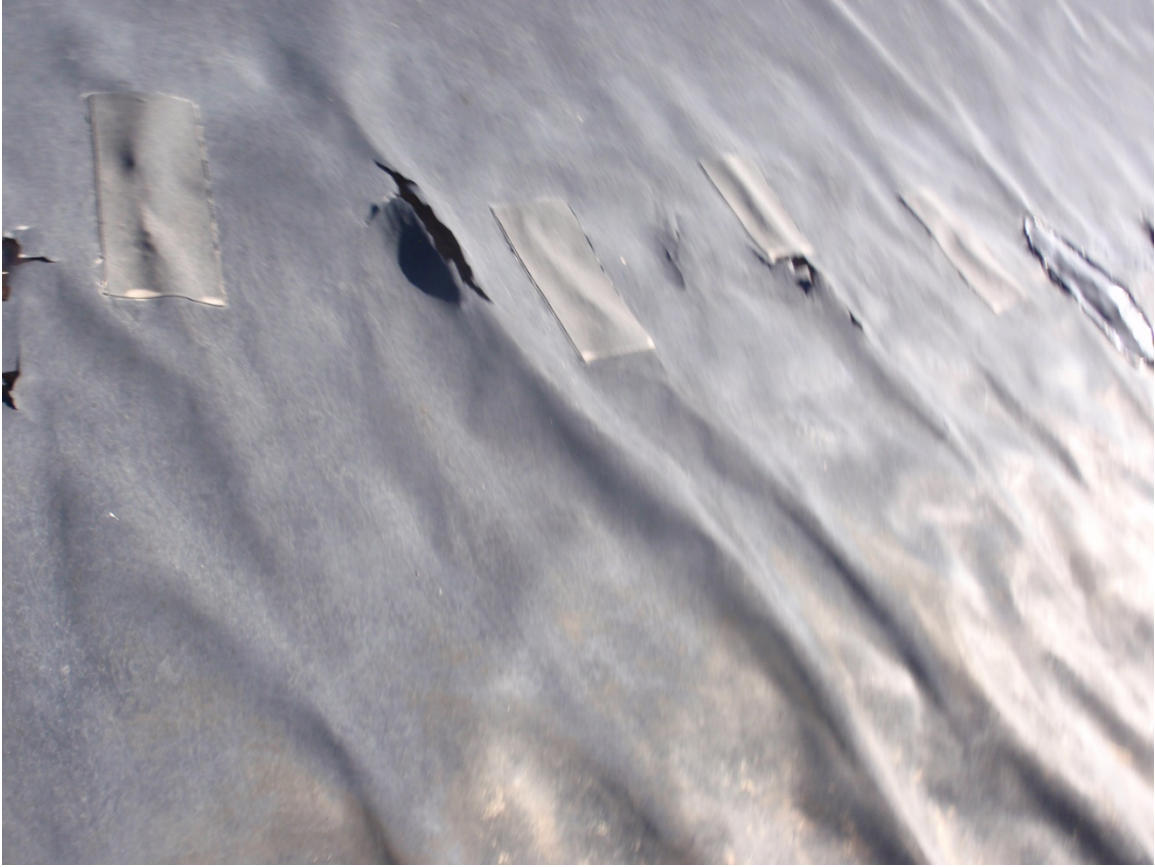
Photo 69. Damage to liner along north side of pit
