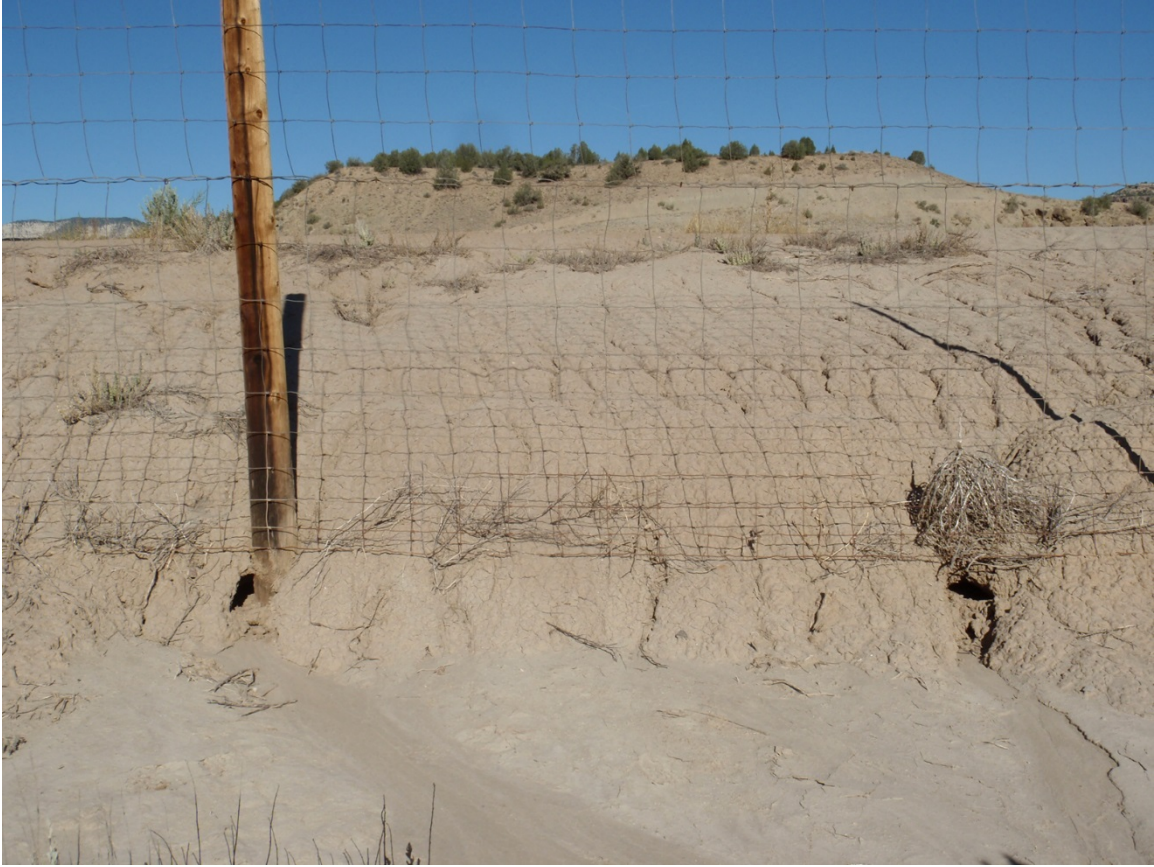
Photo 17. East side of facility looking west. Soil is migrating offsite and into drainage.
