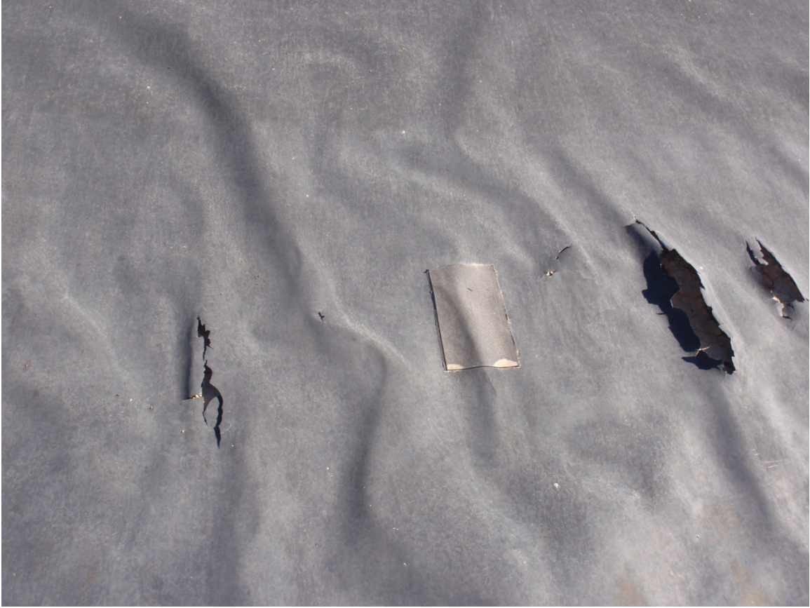
Photo 65. Damage to liner along north side of pit
