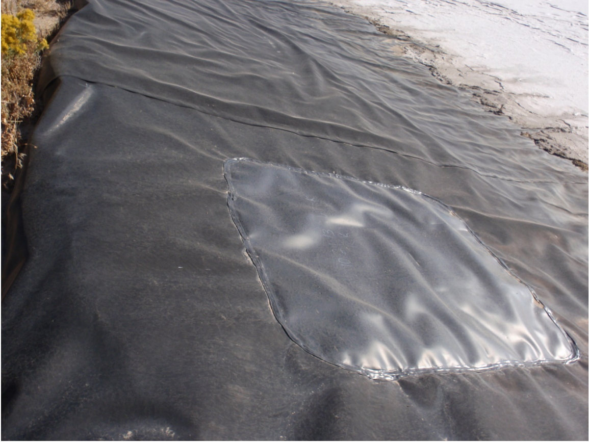
Photo 37. Older patch in liner on west side of pit.
