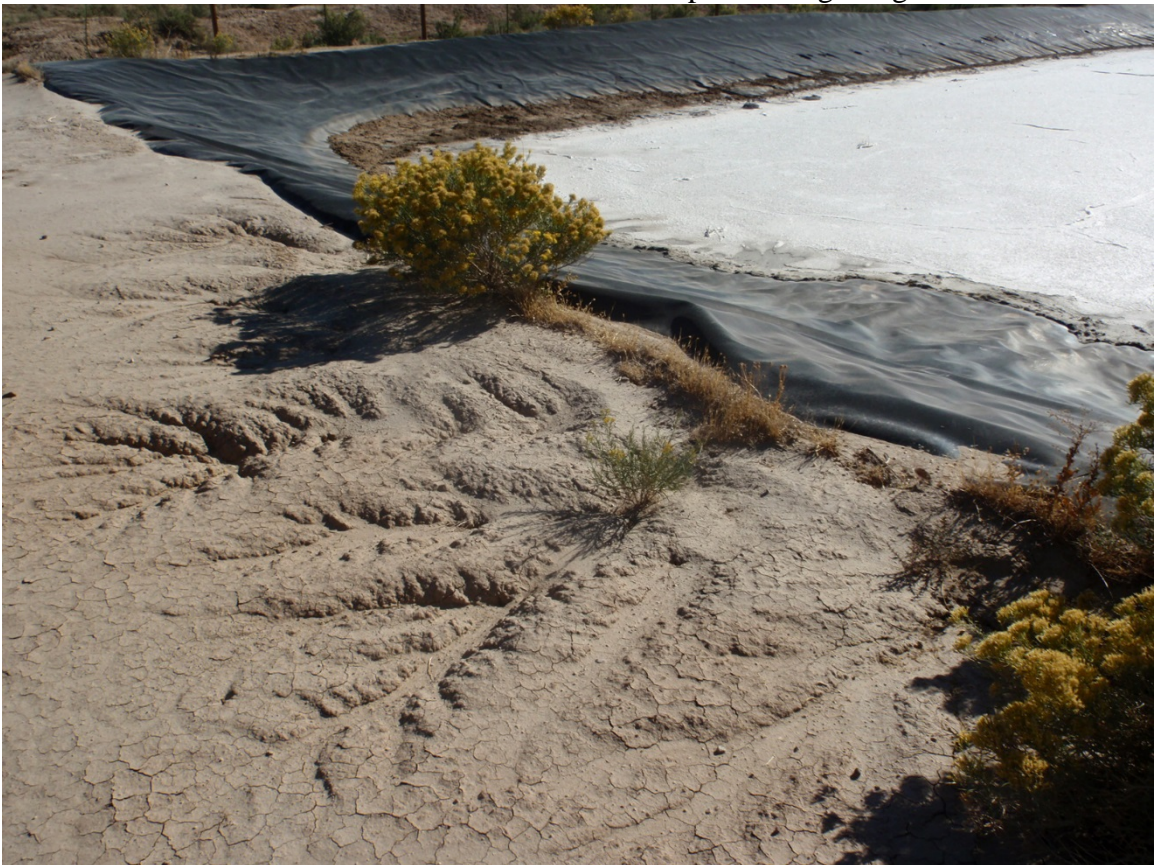
Photo 48. Erosional rill at northwest corner of pit soil migrating under liner
