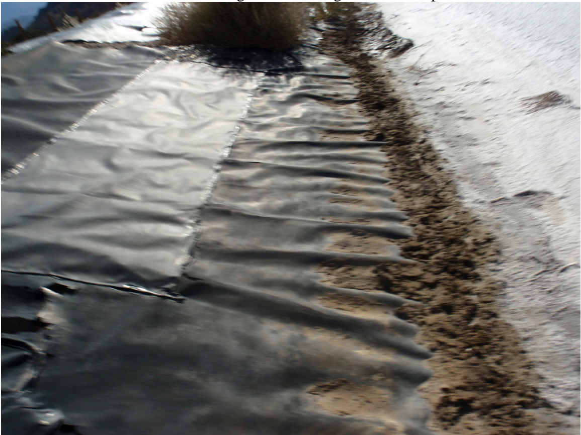
Photo 81. Damage to liner along north side of pit, accumulation of sediment in pit.
