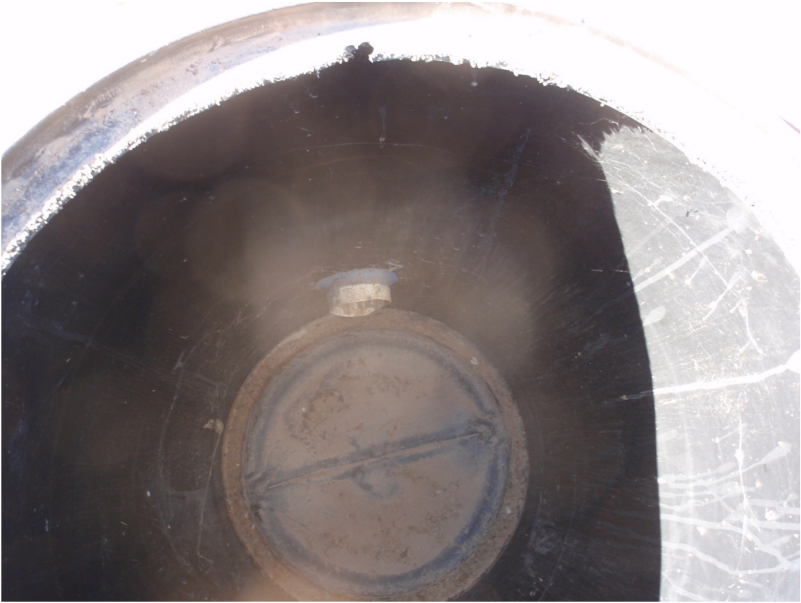
Photo 100. Leak detection system, no water present
