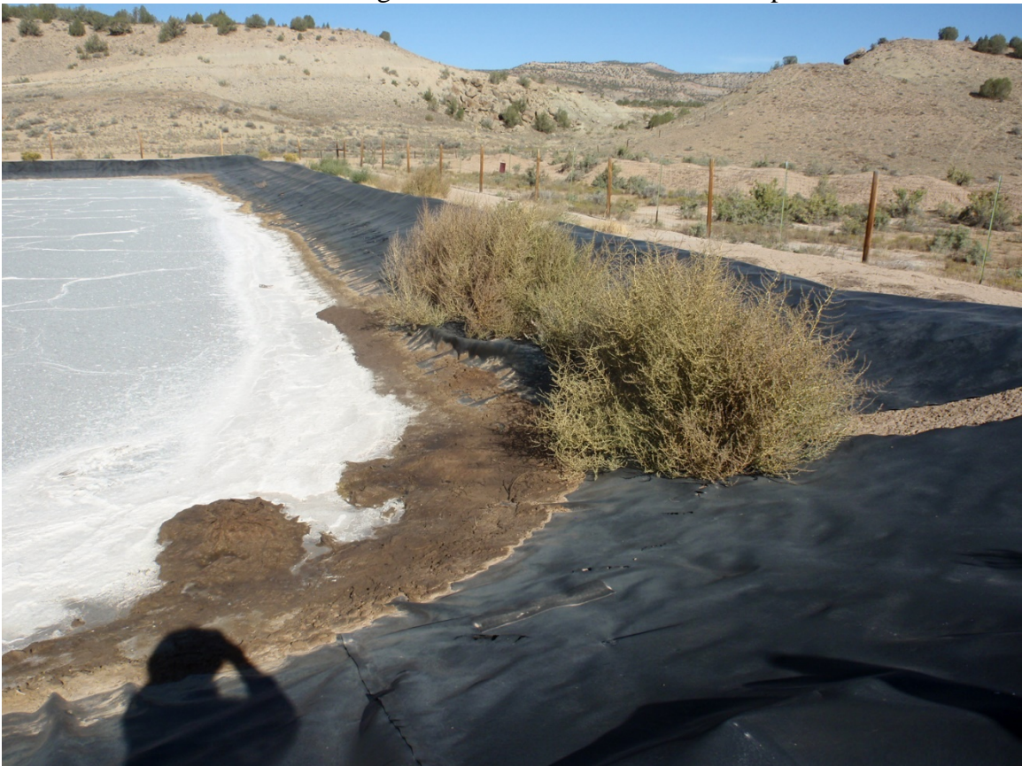
Photo 87. Large tear in liner at northeast side of pit
