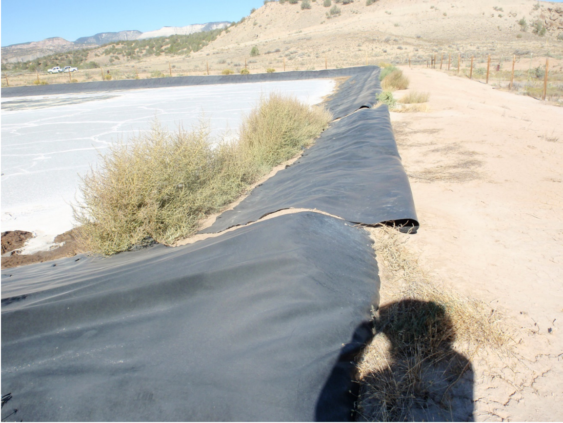
Photo 86. Large tear in liner at northeast side of pit
