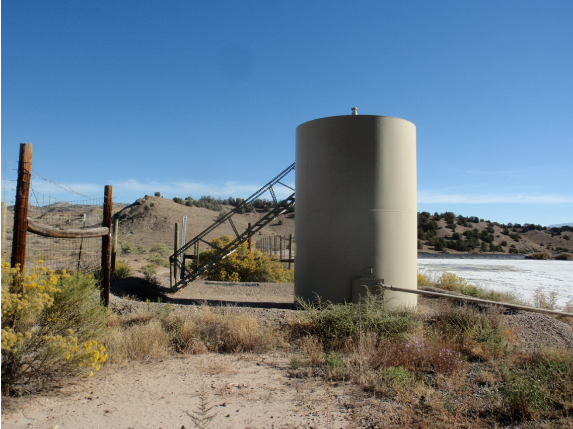
Photo 27. 300 barrel tank and shallow containment berm
