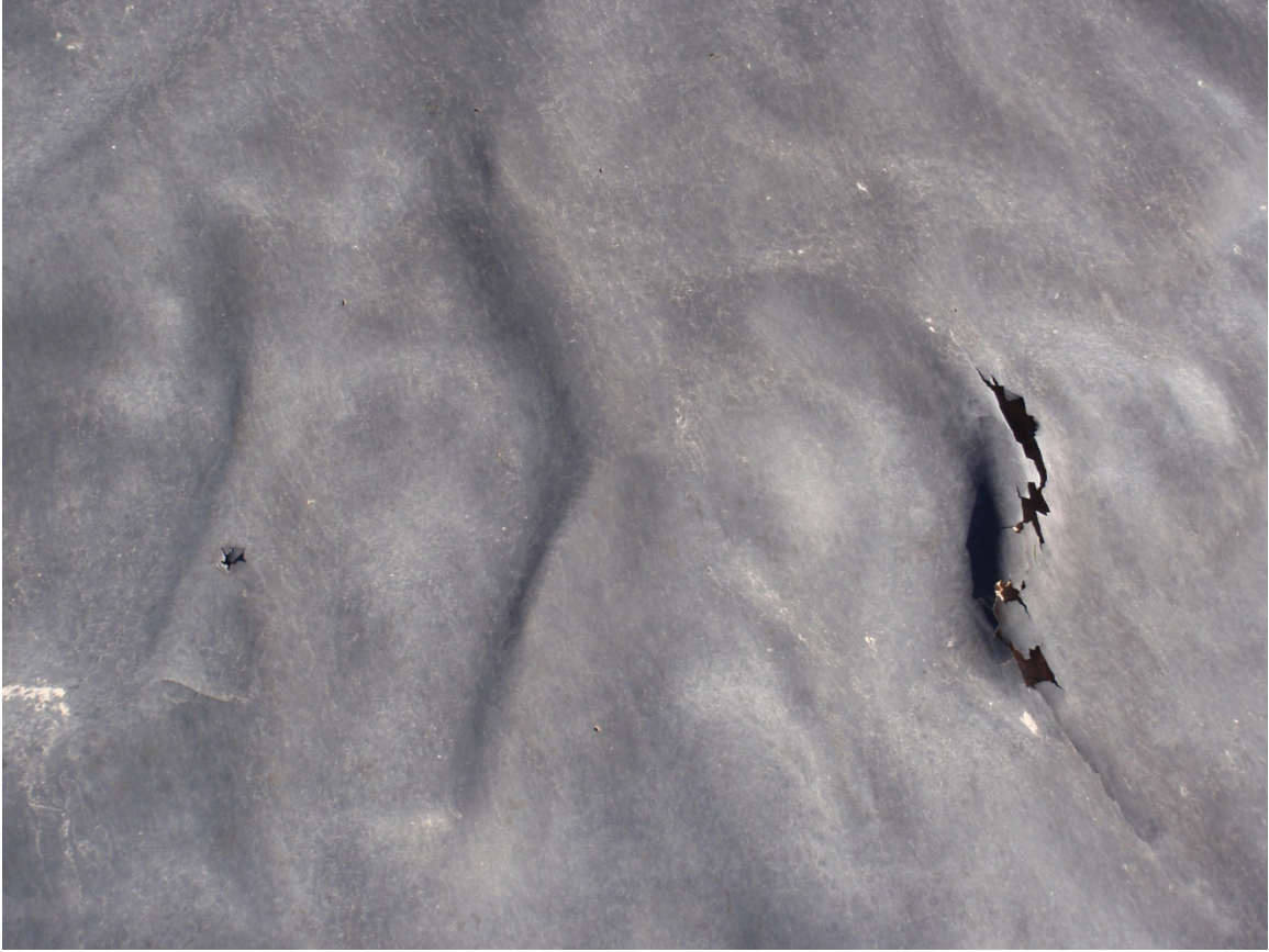
Photo 61. Damage to liner along north side of pit
