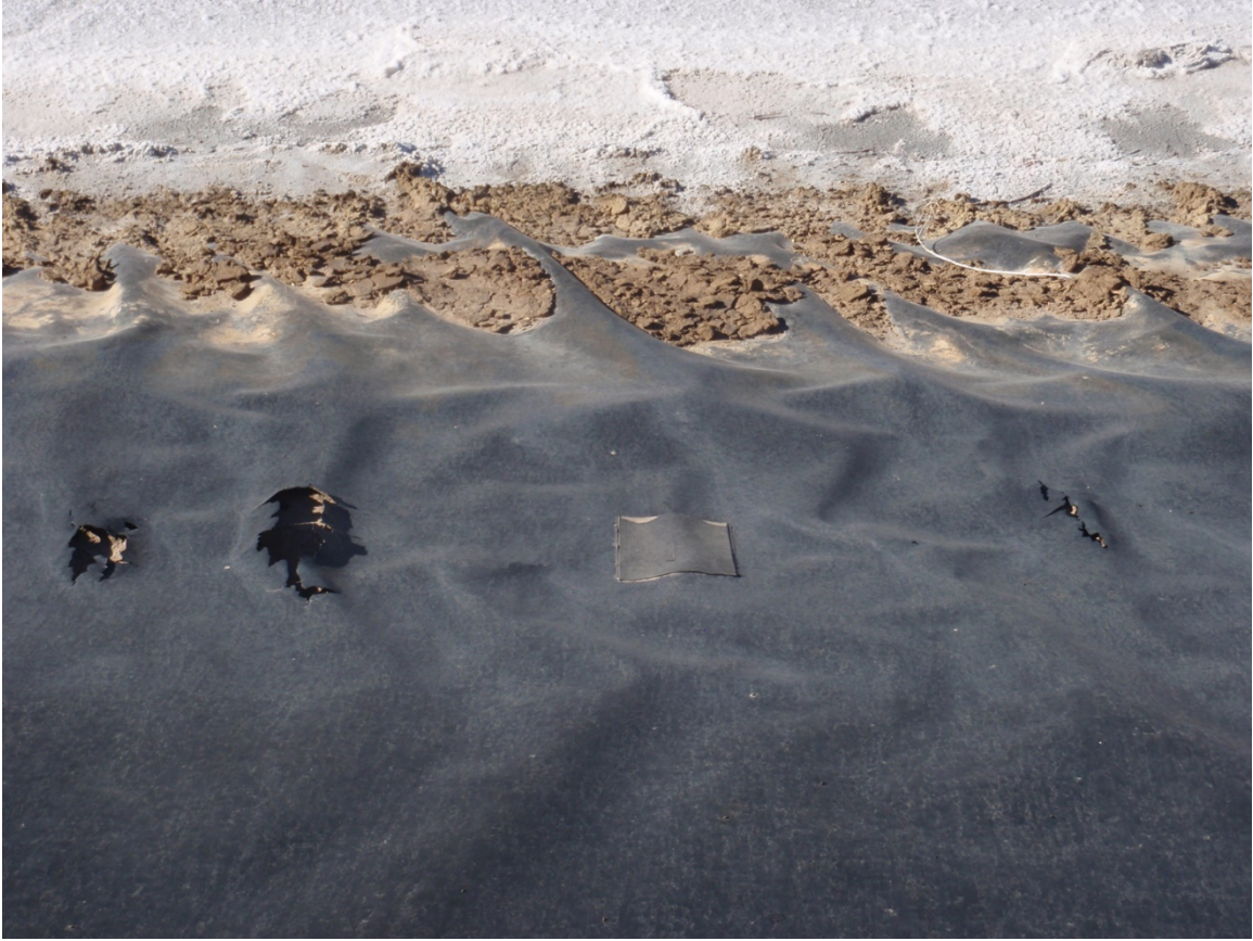
Photo 57. Damage to liner along north side of pit
