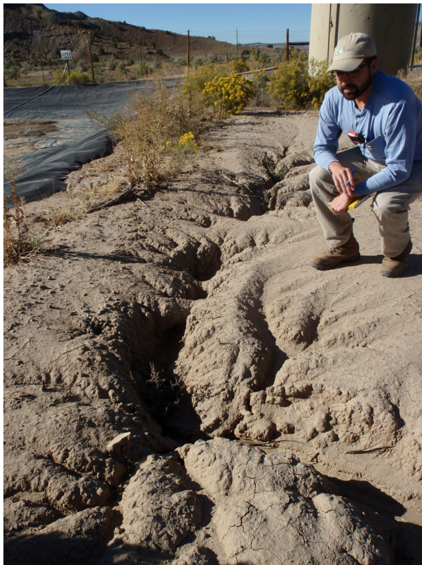
Photo 40. Erosion on berm on west side of pit
