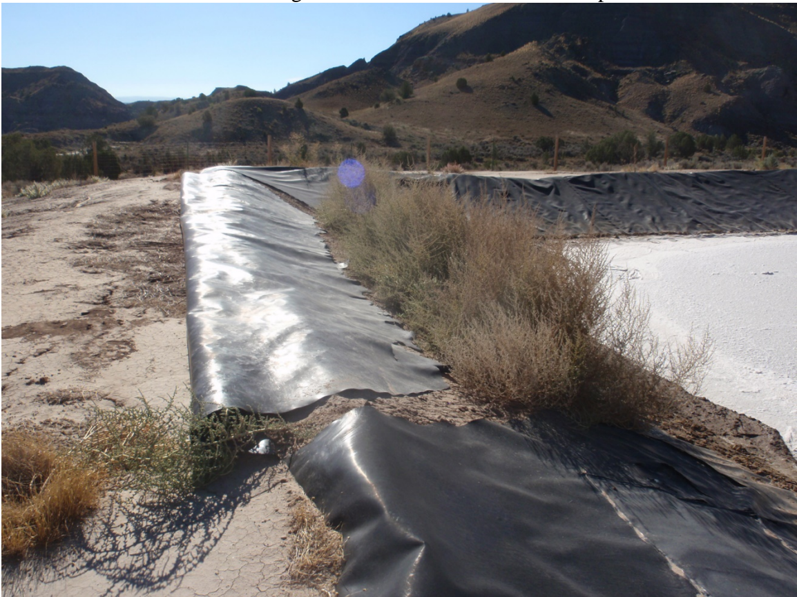
Photo 85. Large tear in liner at northeast side of pit
