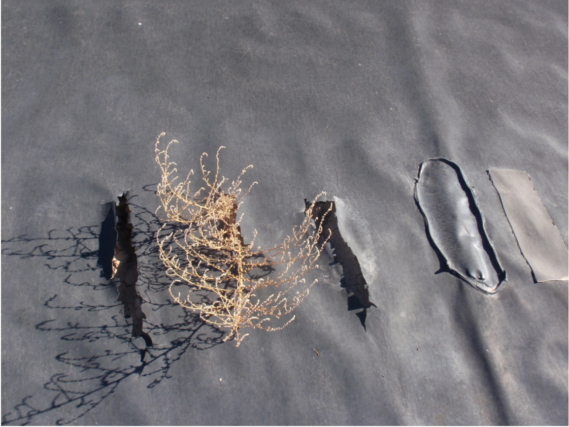
Photo 70. Damage to liner along north side of pit
