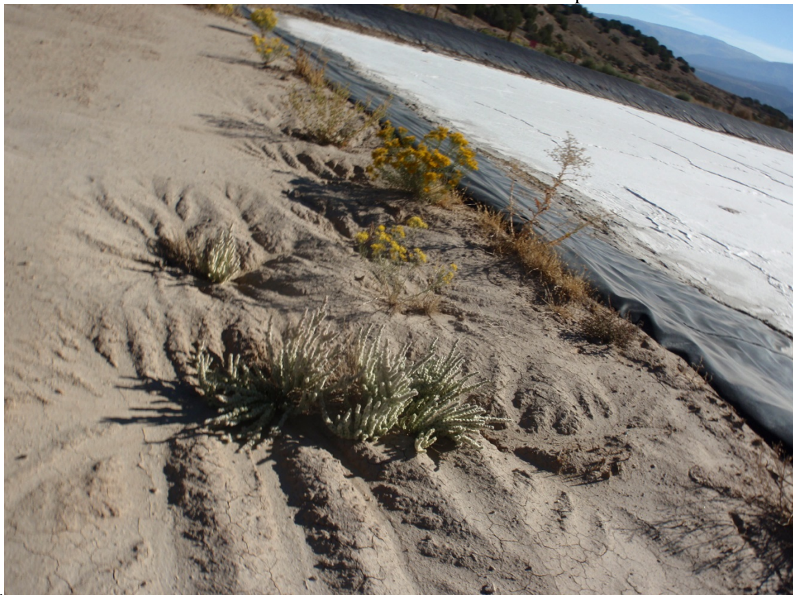
Photo 44. Erosion on berm on west side of pit
