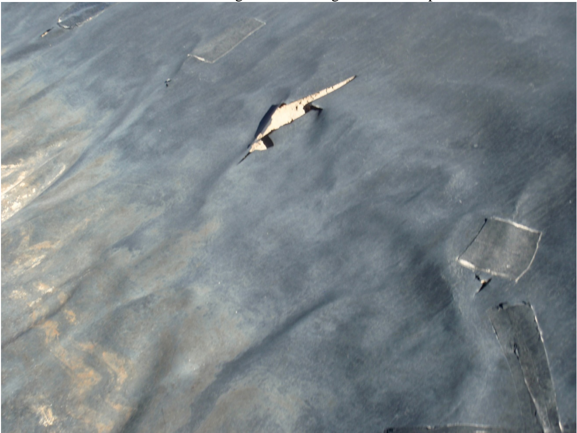
Photo 74. Damage to liner along north side of pit
