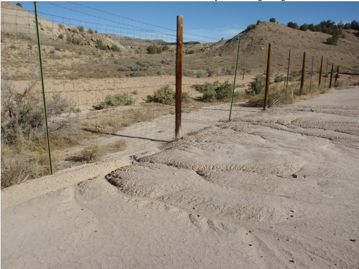
Photo 46. Erosion on berm on west side of pit, soil migrating offsite.
