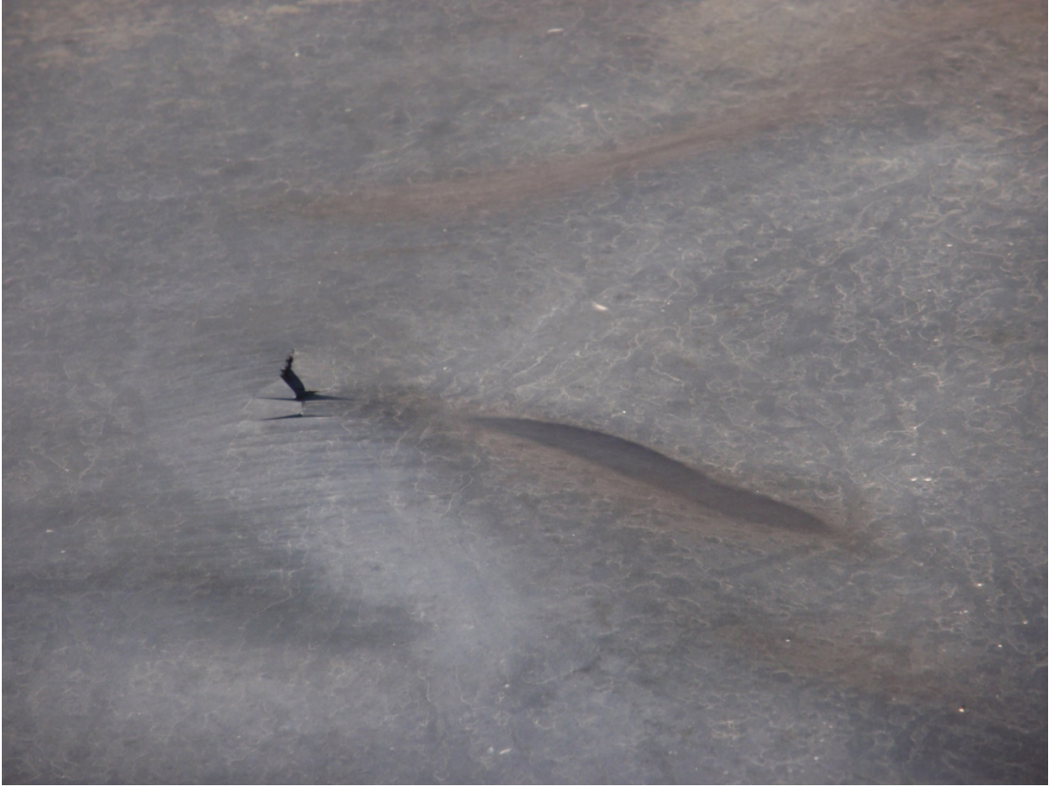
Photo 90. Damage to liner at northeast corner of pit.
