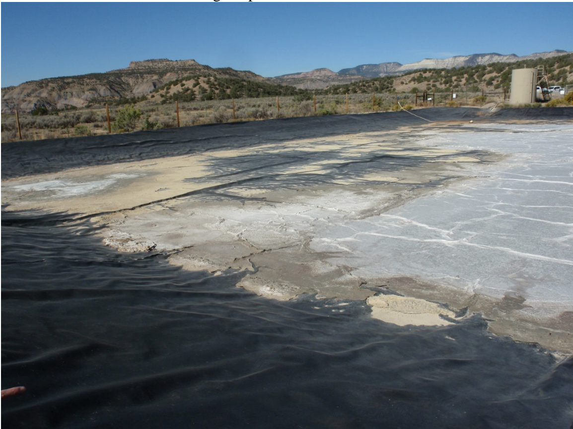
Photo 107. Sediment accumulating in pit possibly from berm erosion
