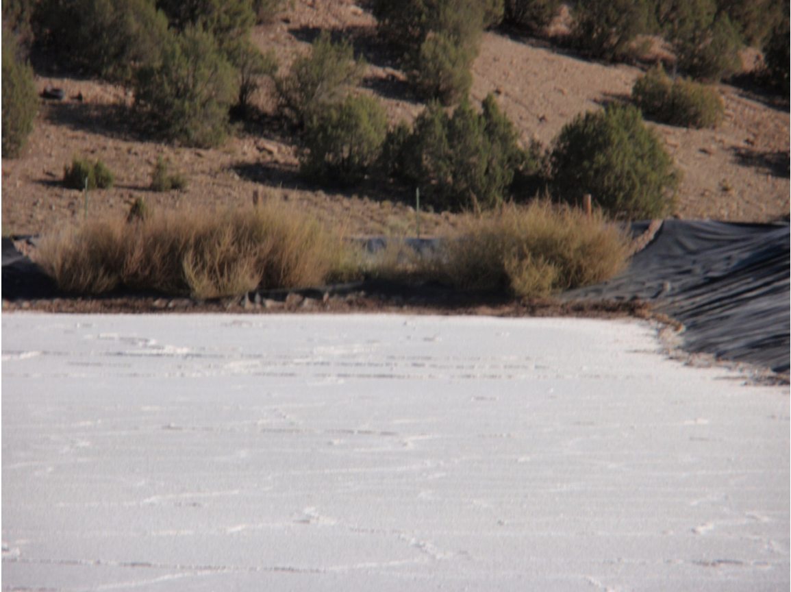
Photo 25. View of facility looking north, accumulation of salts and soils in pit. Liner torn.
