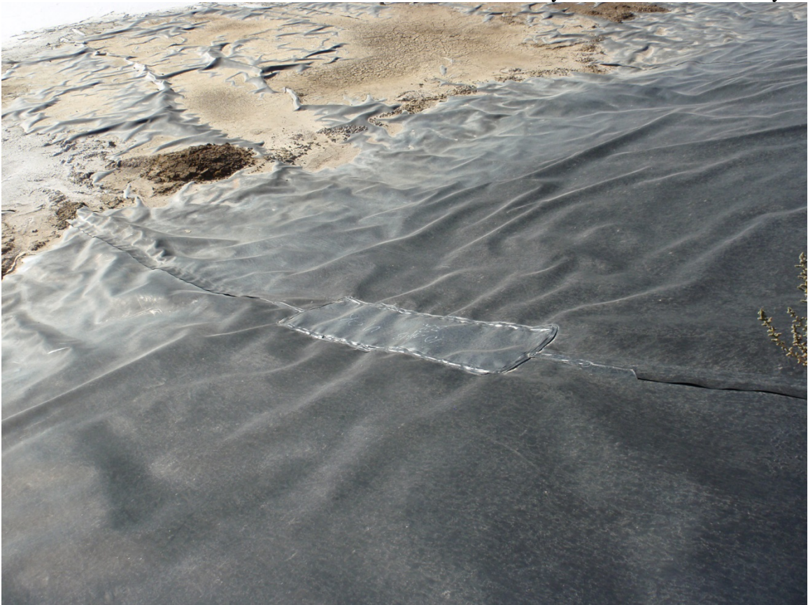
Photo 36. Older patch in liner on west site of pit.
