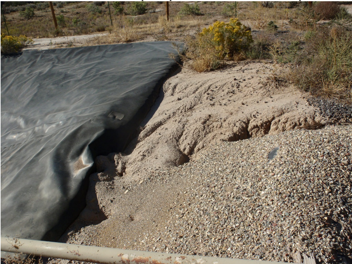
Photo 34. Erosion next to 300 bbl tank soils migrating under pit liner.
