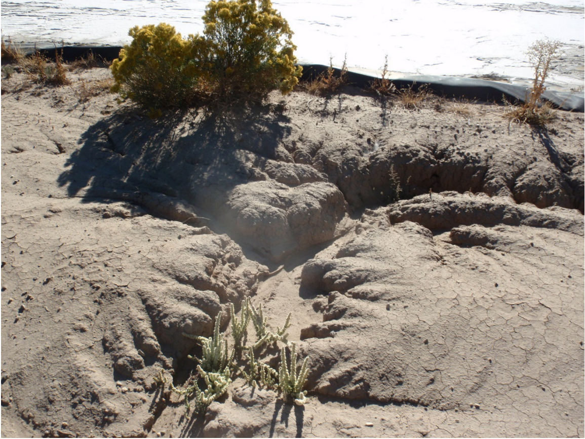
Photo 39. Erosion on berm on west side of pit, Halogeton in foreground.
