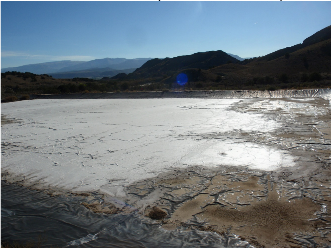
Photo 32. View of central part of pit, soil and salt accumulation in pit.
