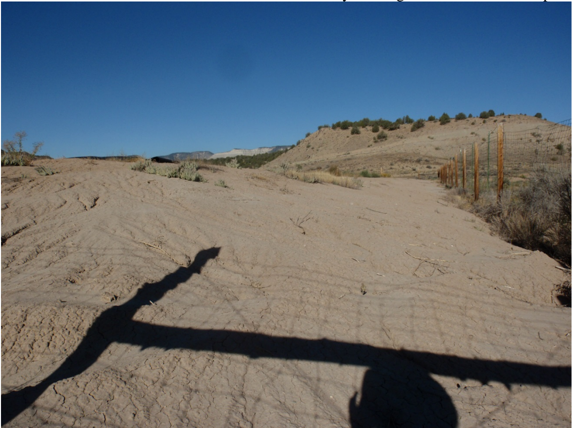
Photo 16. Northeast corner of facility looking west. Erosion occurring along entire berm.
