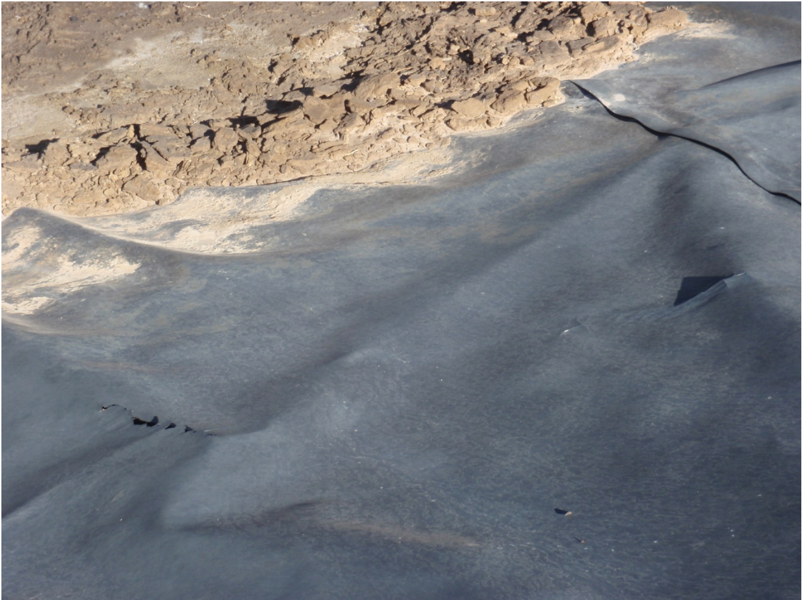
Photo 91. Damage to liner at northeast corner of pit.
