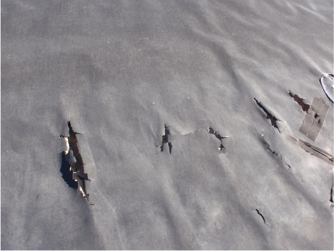
Photo 67. Damage to liner along north side of pit
