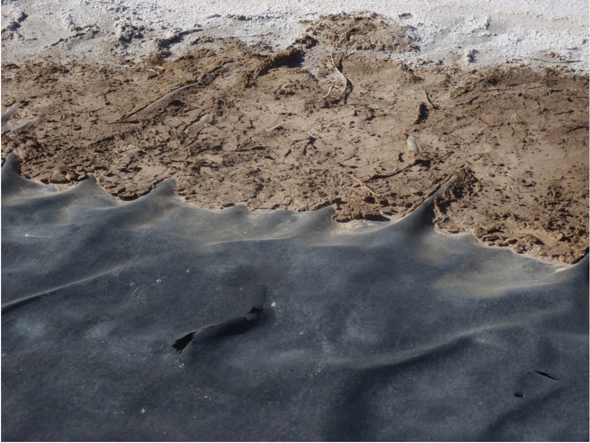
Photo 55. Damage to liner along north side of pit
