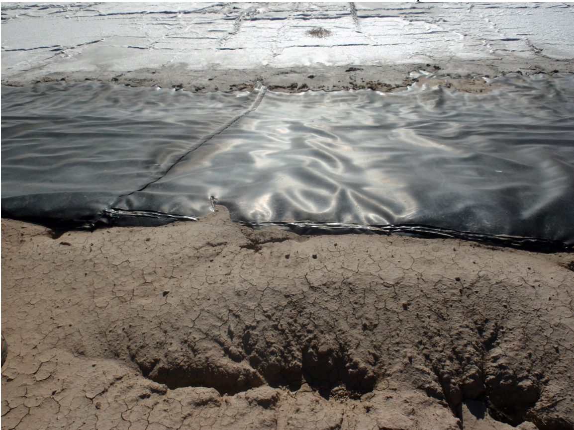
Photo 42. Erosion on berm on west side of pit
