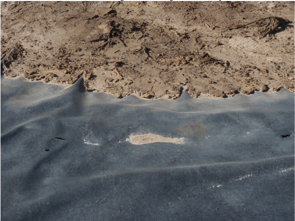
Photo 54. Damage to liner along north side of pit
