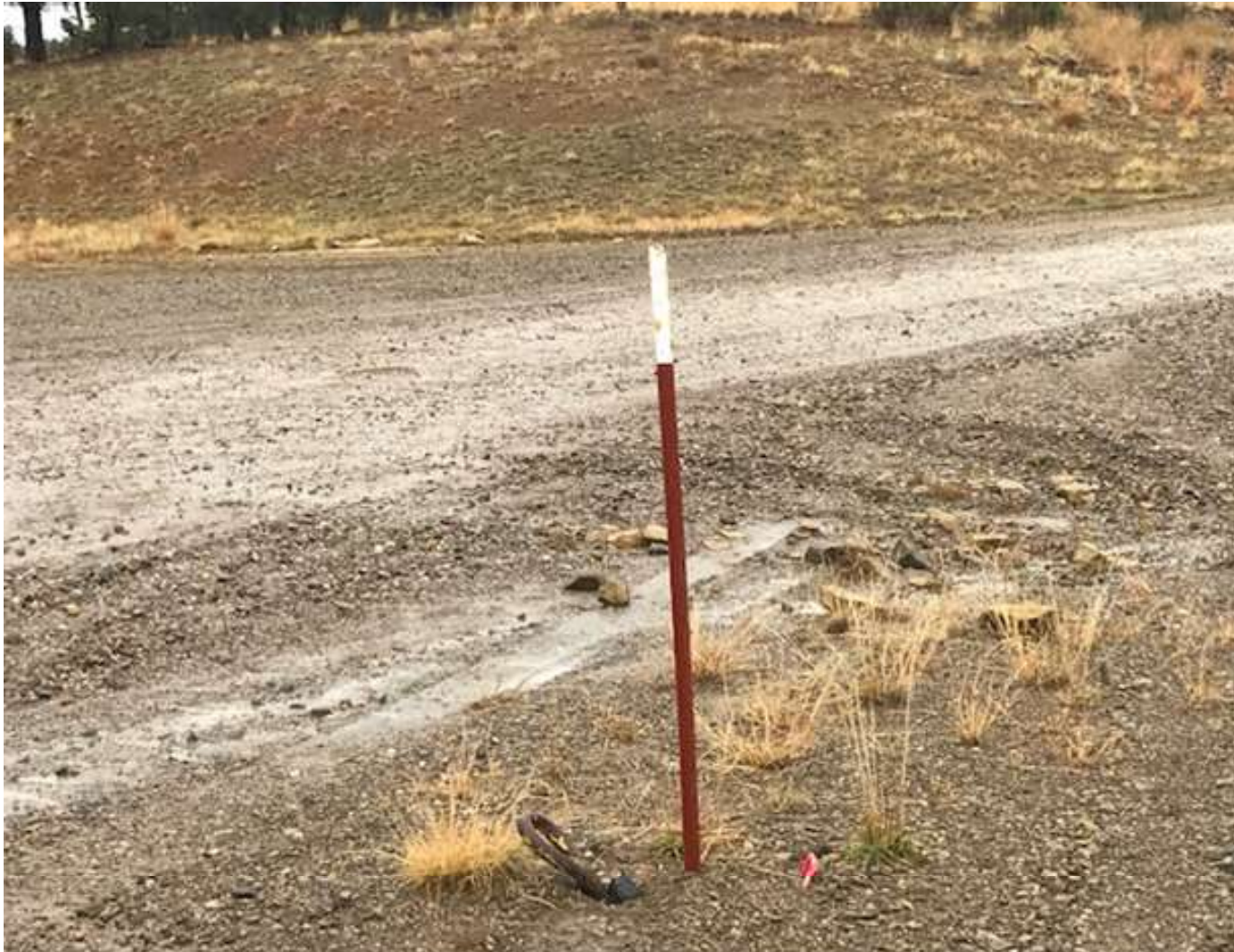
A RED POST WAS INSTALLED ON THE DEADMAN ANCHOR IN COMPLIANCE WITH RULE 604.c.Q.
