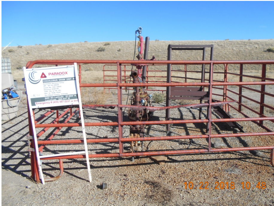
Wellhead with fence and sign
