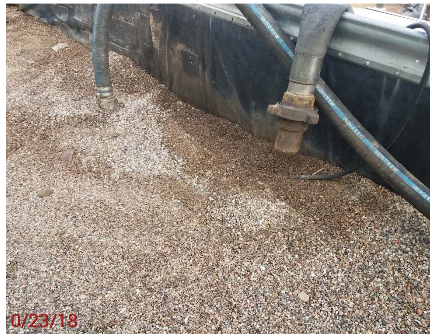
Location Photo #6, stained oily material in containment battery.
