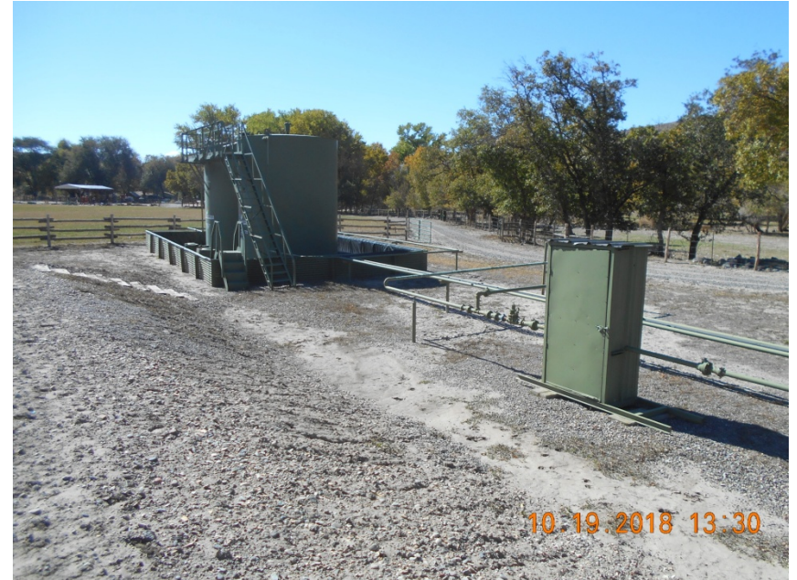
Meter housing and Tank battery
