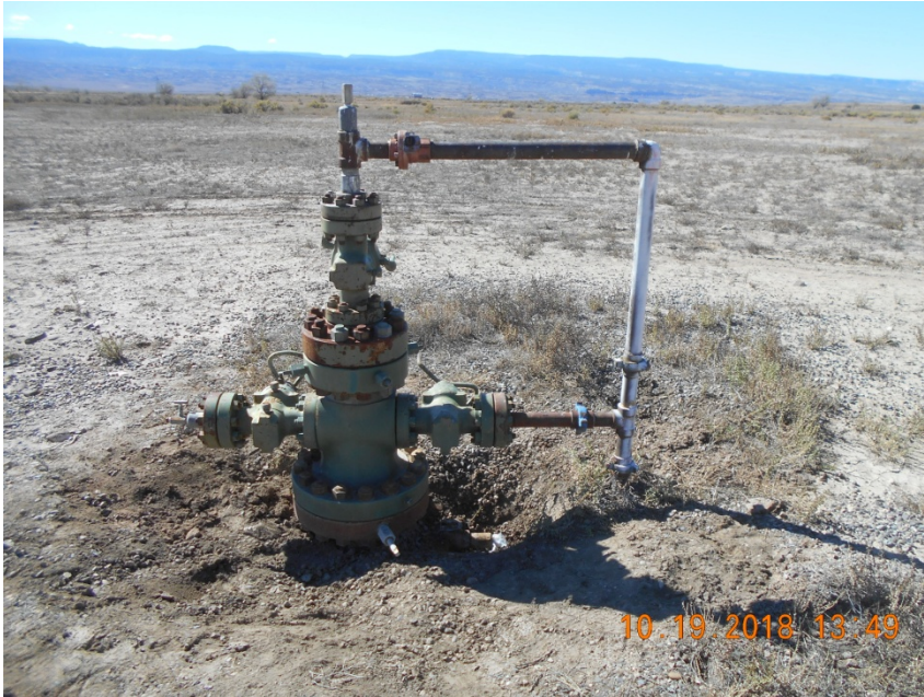
Wellhead with bradenhead valve exposed.
