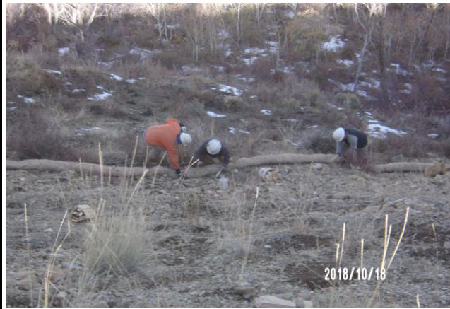
Wattle Installation on the C.C. 608-41 Pad
