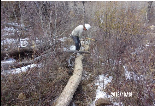
Wattle Installation on the C.C. 608-41 Pad
