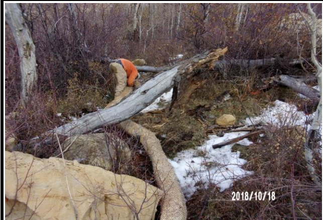
Wattle Installation on the C.C. 608-41 Pad
