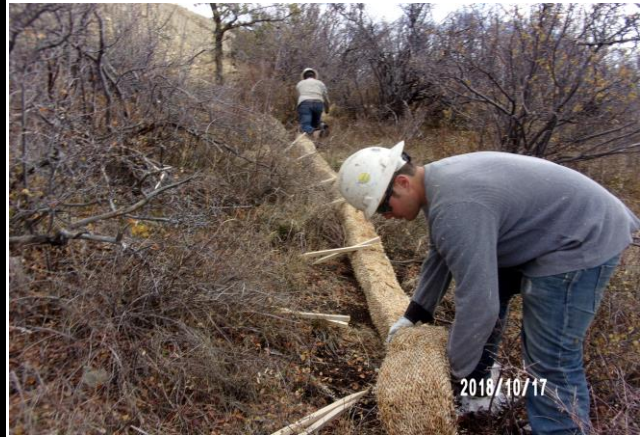
Wattle Installation on the C.C. 608-41 Pad
