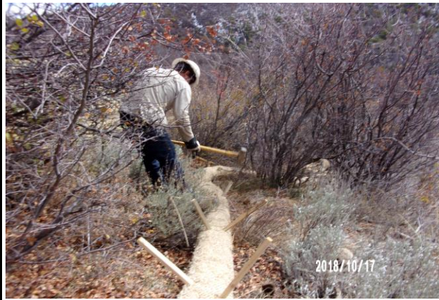
Wattle Installation on the C.C. 608-41 Pad
