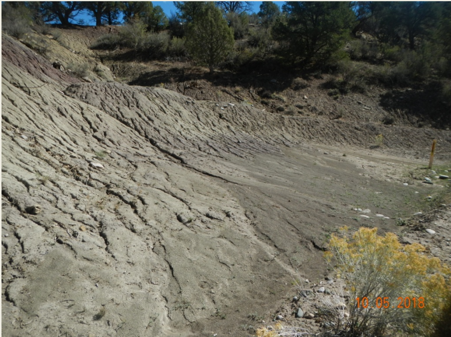
Photo 5. View of the northeastern project area where soils are not stabilized and berms/stormwater controls are not functioning properly.
