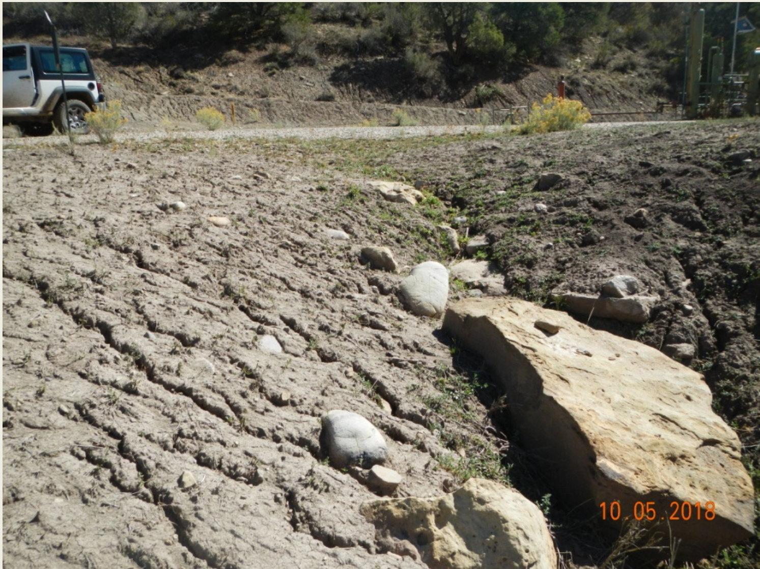
Photo 6. View of erosional channel in the northwestern project, facing upslope, area where adjacent soils are not stabilized and stormwater flows erode the slope toward the western drainage.
