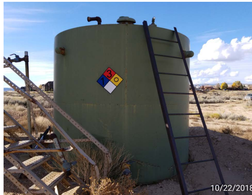
Tank not in use without signage of capacity and contents
