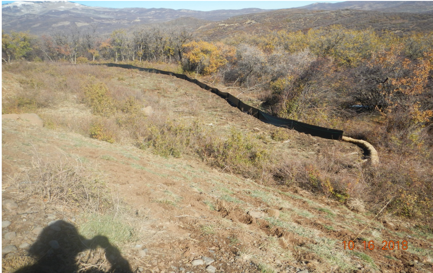
Photo#2: View of Silt fence installed as perimeter control.
