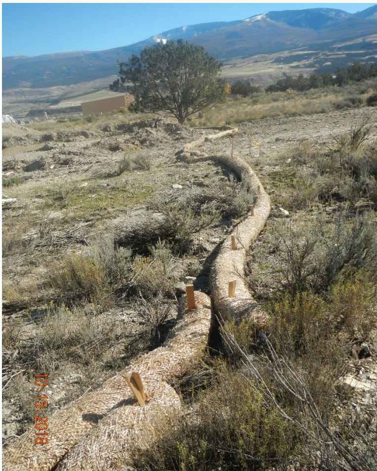
Photo#3: Wattles are installed on location perimeter.
