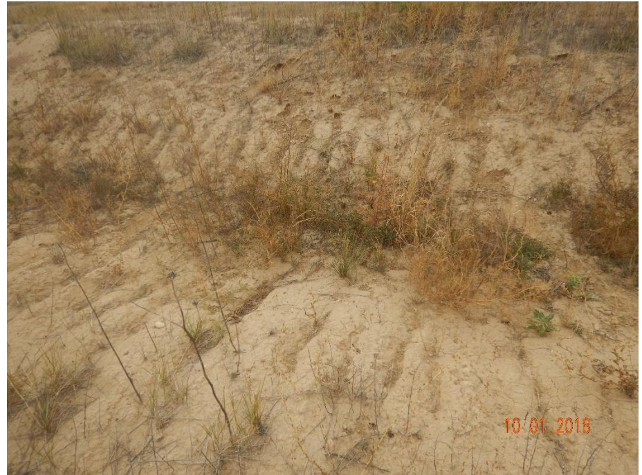
Photo 42: Photo taken from the ditch on the west end of the pad. Photos show stormwater runoff from the pad into the ditch has created rill erosion.
