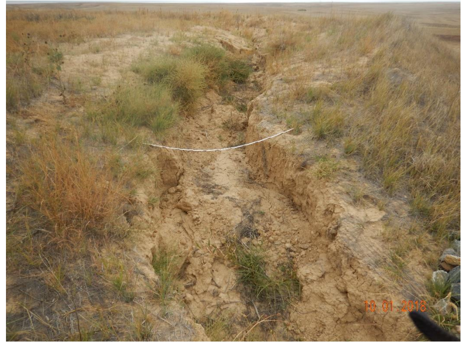
Photo 49: Photos taken from the gully erosion on the northwest end of the pad, facing south. Photo to left dated 2/27/2018 shows stormwater runoff erosion from the pad has blown out the ditch, velocity checks and erosion control blanket, creating a large gully. Photo on the right shows progression of the erosion degradation. 6 foot measuring stick for reference.
