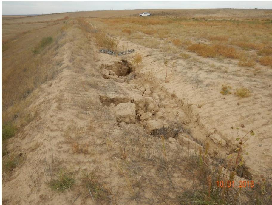
Photo 35: Continued from photo 32. Photo shows erosion degradation occurring, and sinkhole forming within the ditch on west end of the pad.
