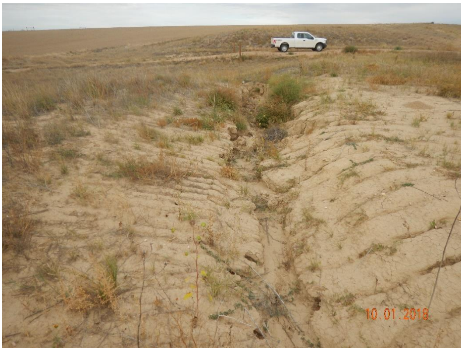
Photo 44: Photo taken from the northwest corner of the pad, facing east. Photo shows erosion degradation within the ditch. Stormwater runoff has blown out controls (erosion blanket, velocity checks) and has created a large gully on the north end of the pad.
