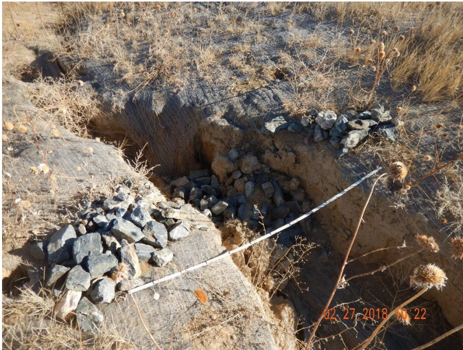
Photo 48: Photos taken from the gully erosion on the northwest end of the pad. Photo to left dated 2/27/2018 shows stormwater runoff erosion from the pad has blown out the ditch, velocity checks and erosion control blanket, creating a large gully. Photo on the right shows progression of the erosion degradation. 6 foot measuring stick for reference.
