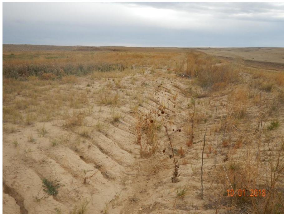
Photo 45: Photo taken from the northwest corner of the pad, facing. Photo shows erosion degradation within the ditch.
