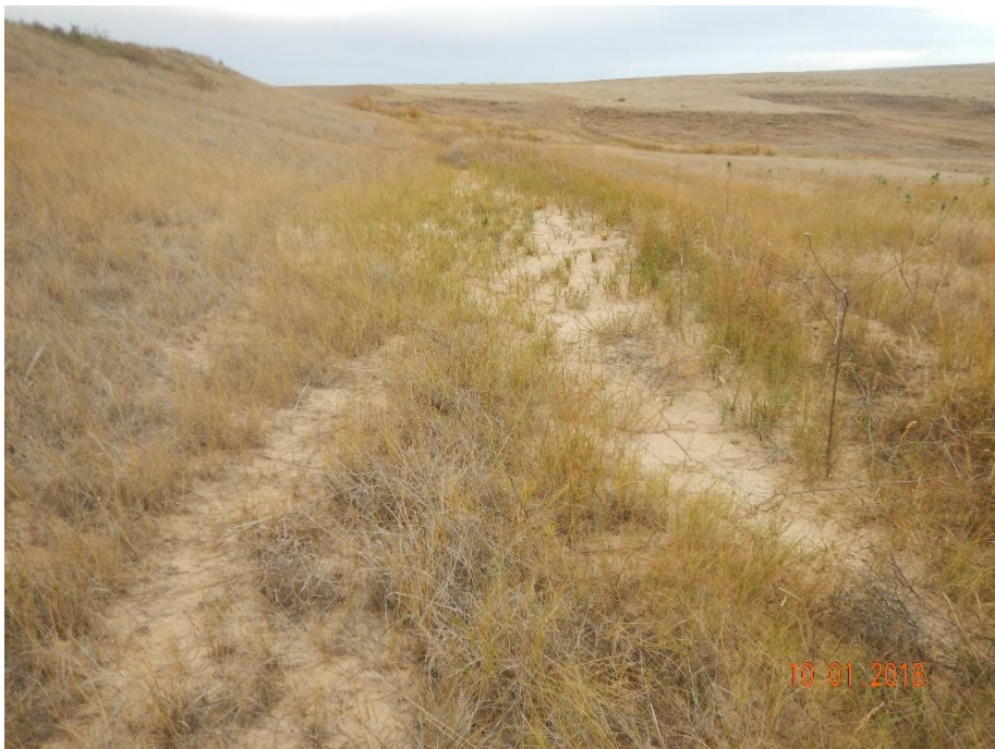
Photo 57: Photo taken from the west end of the location, facing south. Photo shows stormwater ditch along perimeter of location has filled with sediment and is no longer in proper functioning condition.
