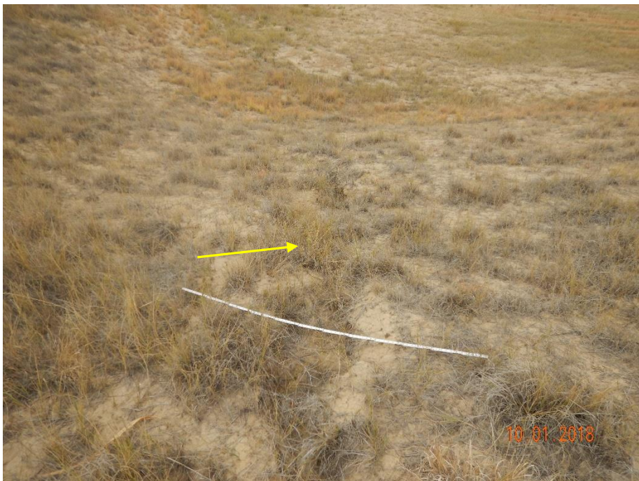
Photo 17: Photo taken from the southeast end of the location. Photo shows cut slopes on the location do not appear to be stabilized; stormwater erosion degradation is forming rill/gully erosion on the slopes and creating pedestal formations around what vegetation has established. 6 foot measuring stick for reference.
