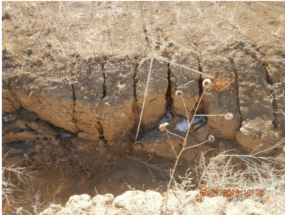
Photo 46: Photos taken from the gully erosion on the northwest end of the pad. Photo to left dated 2/27/2018 shows rill/gully erosion beginning to cut eastward into the pad. Photo on the right shows erosion degradation has progressed further into the pad. 6 foot measuring stick for reference.
