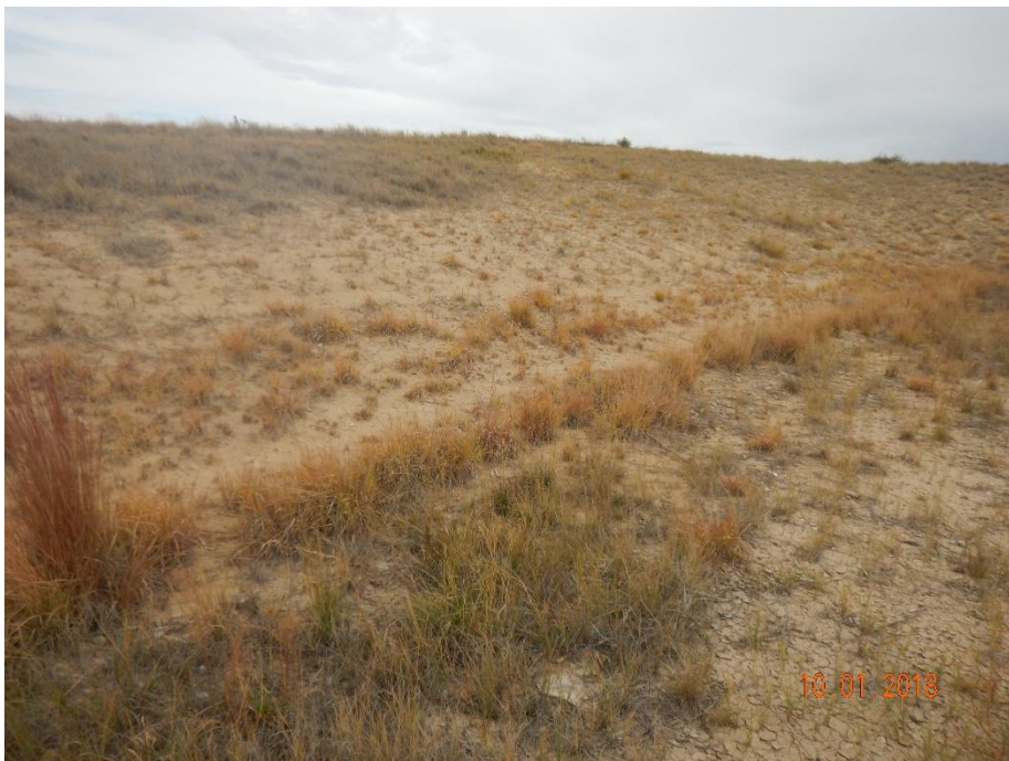
Photo 11: Photo from the northeast corner of the location, facing northeast. Photo shows cut slopes on the location do not appear to be stabilized; vegetation has not achieved a uniform establishment and stormwater erosion degradation is forming rill/gully erosion on the slopes. These areas remain predominantly bare and exposed soil and are at risk for further erosion degradation.
