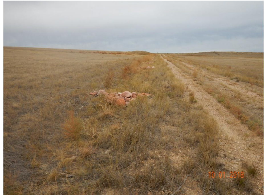
Photo 4: Photo taken from the access road, facing southeast. Photo shows velocity checks and ditch along access road. BMPs appear to be in proper functioning condition.
