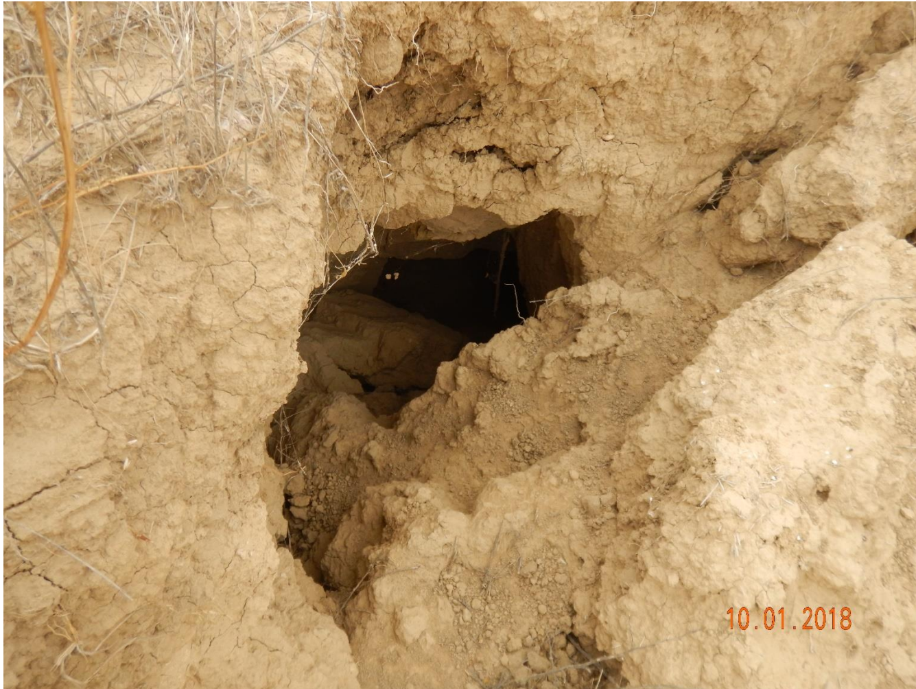
Photo 34: Continued from photo 33. Photo shows depth at which stormwater has created a sinkhole and cut under the pad, appears to exceed 10 feet down.
