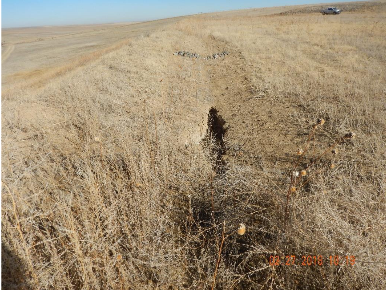
Photo 31: Photo date 2/27/2018. Photo taken from the west end of the location, facing north. Photo shows stormwater incision within the ditch.
