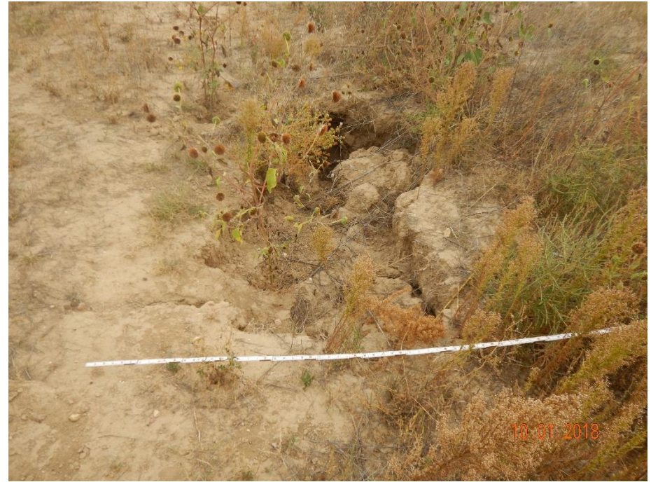
Photo 29: Photos taken from the stormwater ditch on the west end of the location. Photos shows stormwater runoff has incised the ditch along the west end of the pad. Photo on left (facing west) taken during a site visit 2/27/2018. Photo on right (facing north) shows progression of the degradation since February 2018. 6 foot measuring stick for reference.
