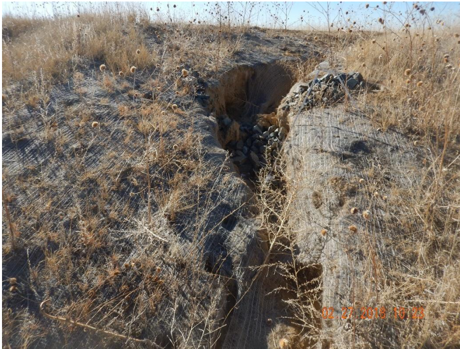
Photo 49: Photos taken from the gully erosion on the northwest end of the pad, facing south. Photo to left dated 2/27/2018 shows stormwater runoff erosion from the pad has blown out the ditch, velocity checks and erosion control blanket, creating a large gully. Photo on the right shows progression of the erosion degradation. 6 foot measuring stick for reference.
