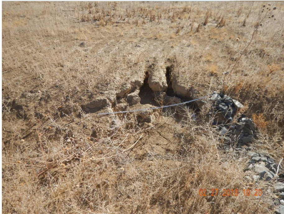
Photo 43: Photos taken from the stormwater ditch on the west end of the pad. Photo on the left dated 2/27/2018 shows stormwater runoff from the pad was creating rill and gully erosion that was beginning to cut eastward into the pad. Photo on the right shows erosion degradation has progressed further into the pad. 6 foot measuring stick for reference.
