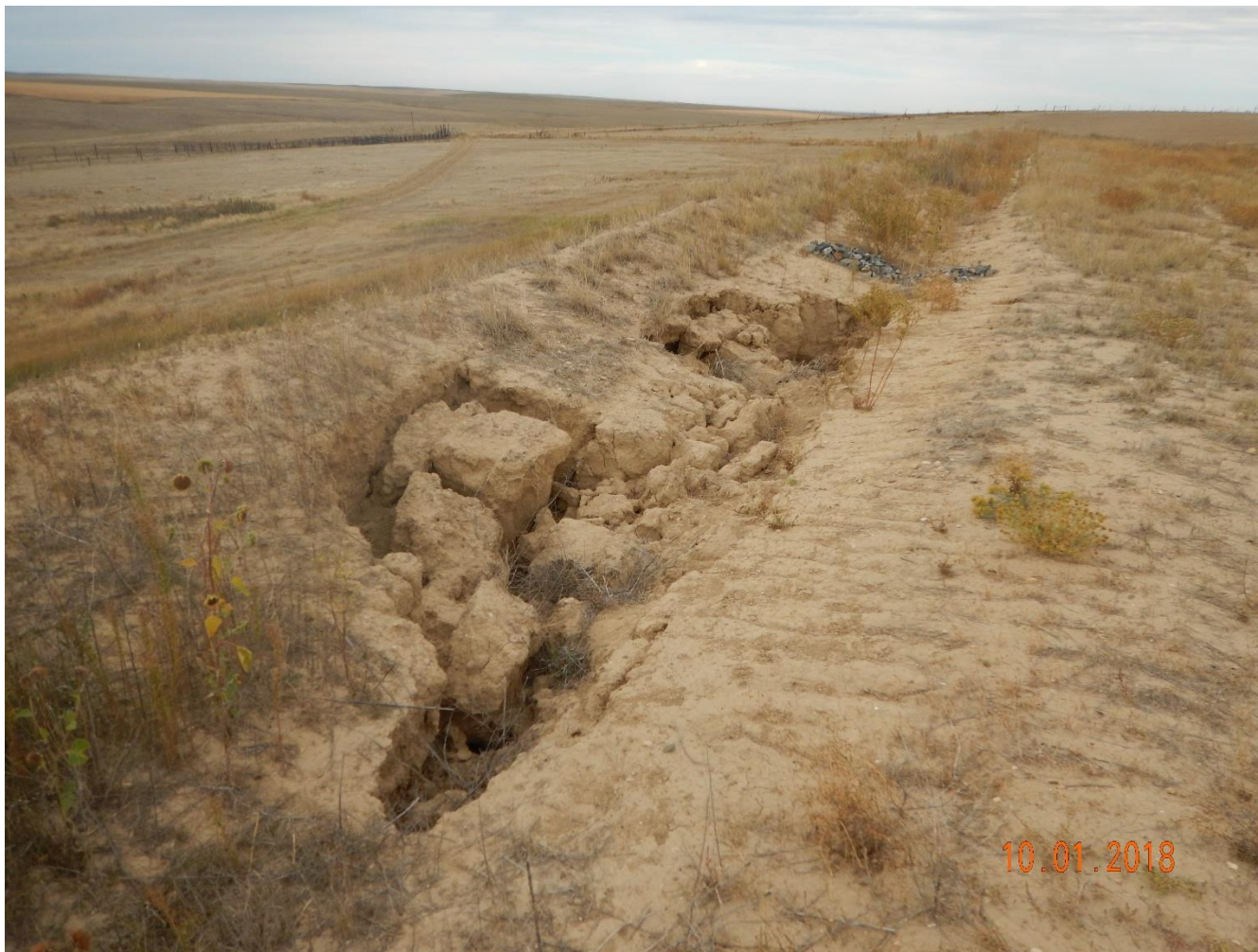
Photo 32: Continued from photo 31. Photo shows progression of the stormwater degradation since February 2018. Please note: water appears to be focusing within this area of the ditch. There is not evidence to suggest stormwater is flowing out of the ditch onto the pad, or off the location. Water appears to be traveling sub-gradient into what appears to be a sinkhole. Pad does not appear to be stable.
