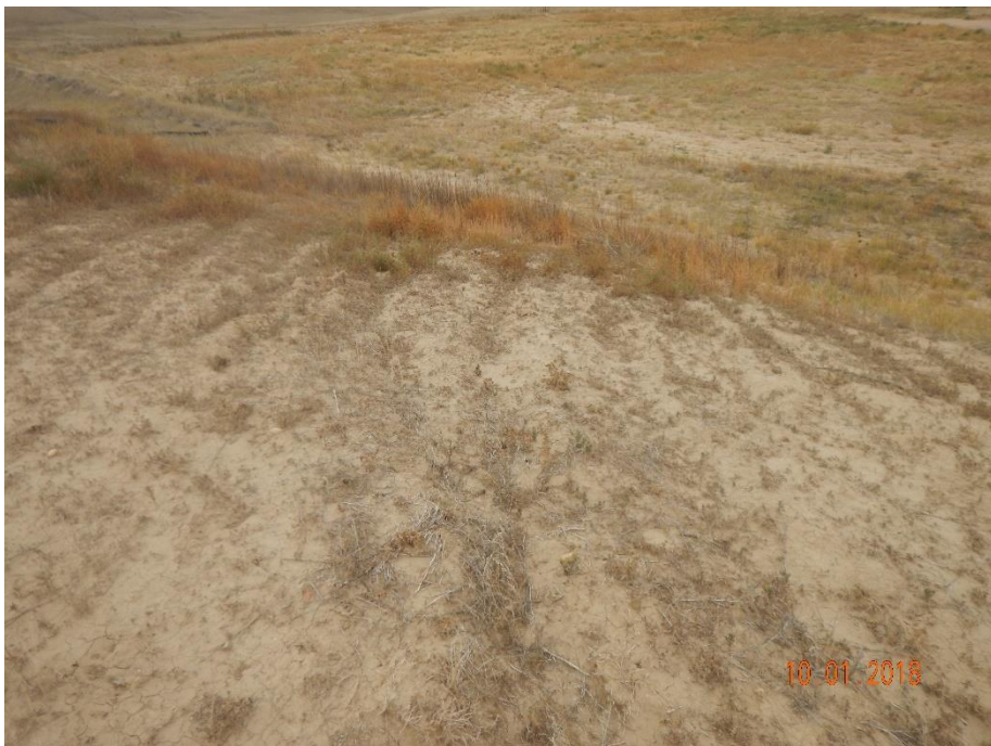
Photo 19: Photo taken from area of the “spoils” stockpile on the south end of the location, facing northwest. Photo shows areas of bare and exposed soil with large furrows. These furrows are similar to those seen after a ripper has roughened soils. This surface roughening has not been performed along the contour of the slope and has created channels to promote stormwater gully erosion degradation. Stockpile is not sufficiently stabilized.
