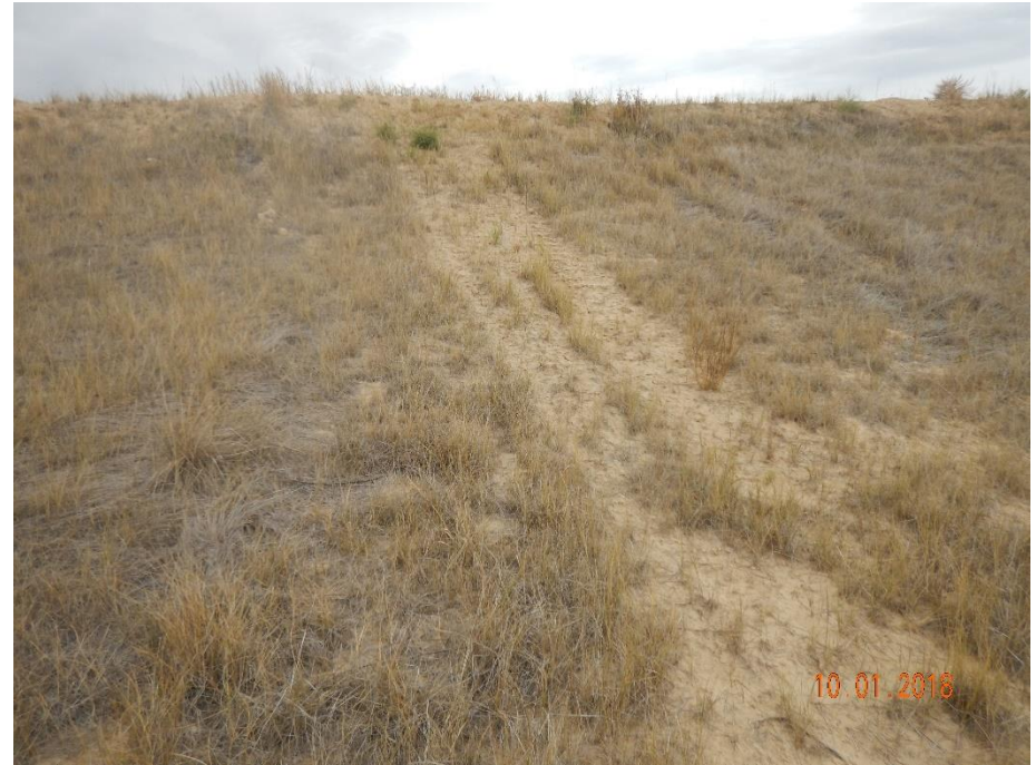
Photo 54: Photo taken from the west end of the location, facing east and upslope. Photo shows areas of the slope that remain predominantly bare and exposed soil. Operator has indicated that these areas had work conducted to repair erosion in 2016.
