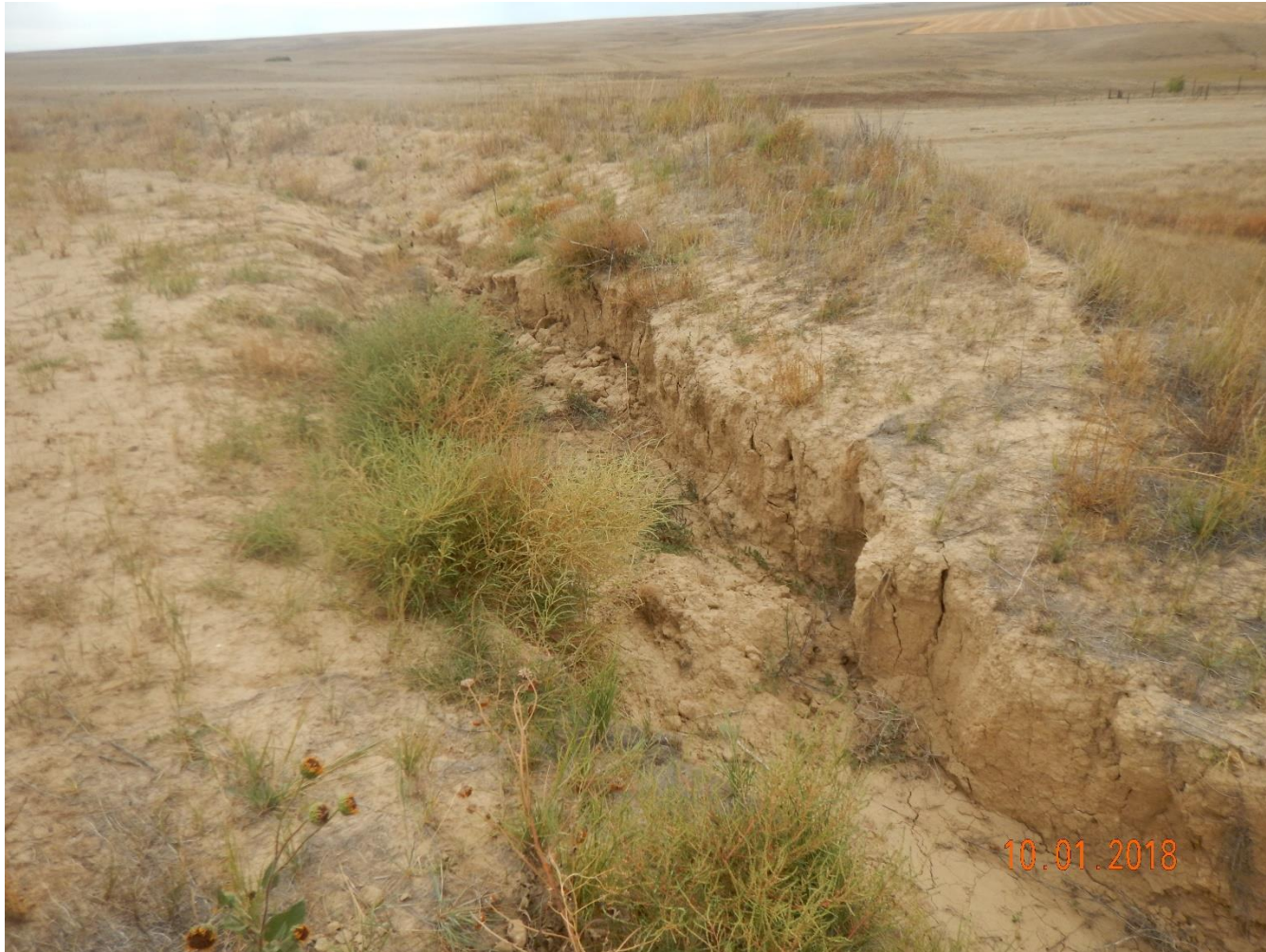
Photo 47: Photo taken from the northwest end of the pad, facing west. Photo shows stormwater runoff from the pad has blown out the ditch, velocity checks and erosion control blanket, creating a large gully.
