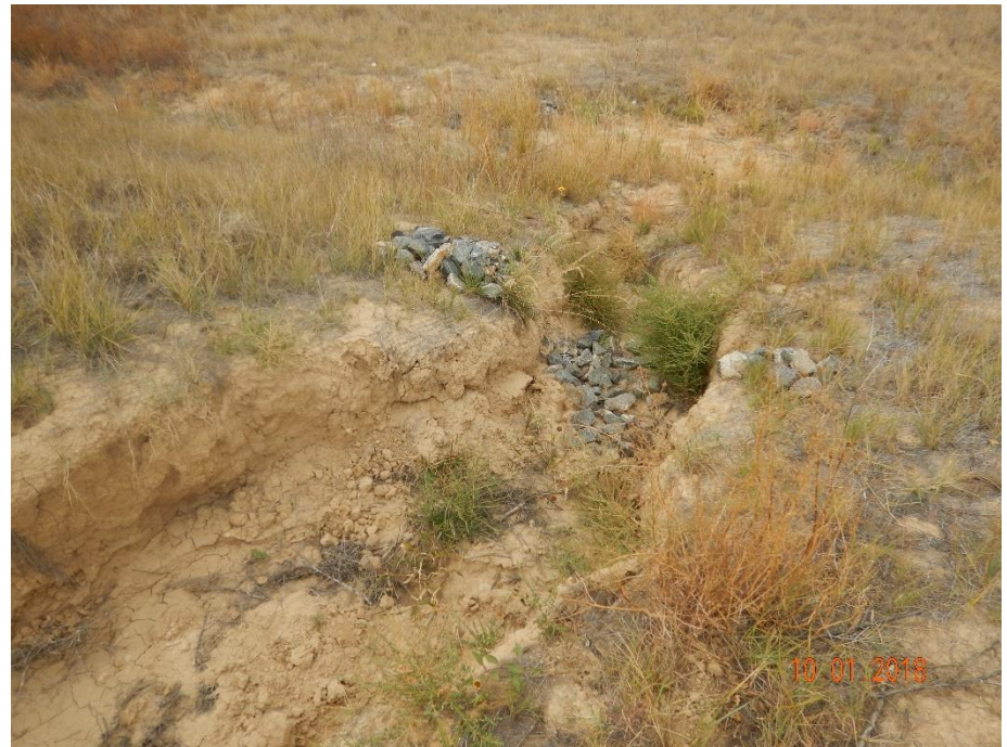
Photo 48: Photos taken from the gully erosion on the northwest end of the pad. Photo to left dated 2/27/2018 shows stormwater runoff erosion from the pad has blown out the ditch, velocity checks and erosion control blanket, creating a large gully. Photo on the right shows progression of the erosion degradation. 6 foot measuring stick for reference.
