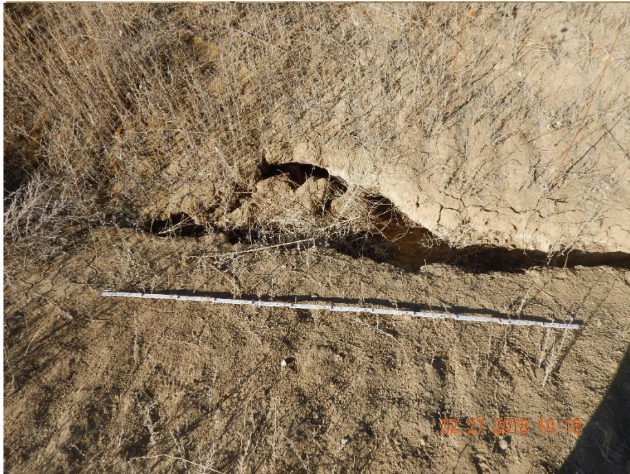
Photo 29: Photos taken from the stormwater ditch on the west end of the location. Photos shows stormwater runoff has incised the ditch along the west end of the pad. Photo on left (facing west) taken during a site visit 2/27/2018. Photo on right (facing north) shows progression of the degradation since February 2018. 6 foot measuring stick for reference.
