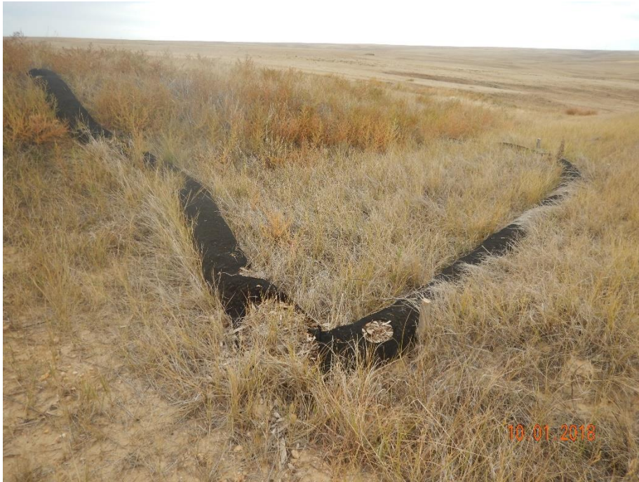
Photo 25: Photo taken from the south end of the location, facing southwest. Photo shows wood-mulch wattle stormwater ponding BMP. BMP showing signs of degradation,
