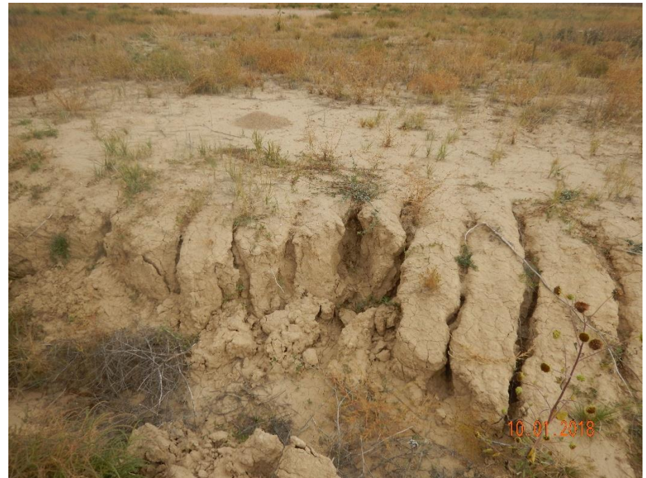
Photo 46: Photos taken from the gully erosion on the northwest end of the pad. Photo to left dated 2/27/2018 shows rill/gully erosion beginning to cut eastward into the pad. Photo on the right shows erosion degradation has progressed further into the pad. 6 foot measuring stick for reference.
