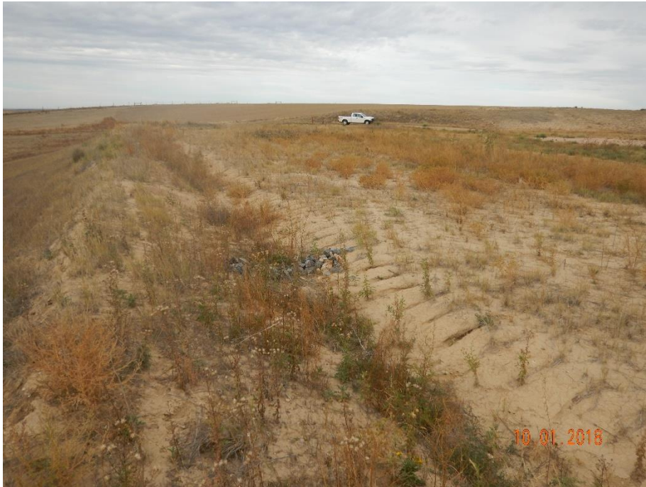
Photo 37: Photo taken from the west end of the pad, facing north. Photos 37-40 provide an overview of the location from north, east, so south. Photos also show stormwater runoff from the pad into the ditch has created rill formations on the slopes of the ditch.
