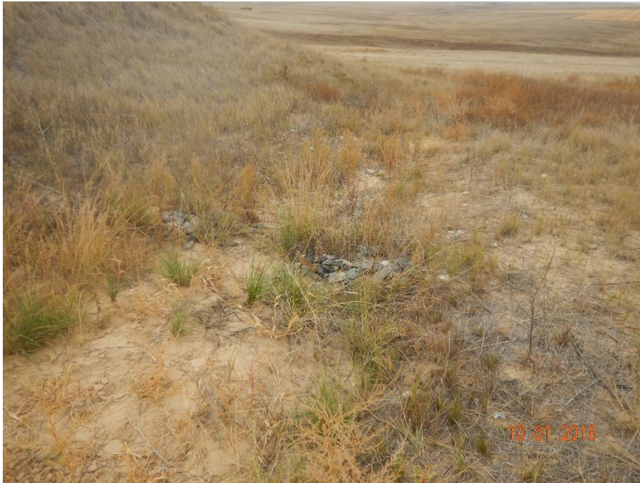
Photo 51: Photo taken from the north end of the location, facing west. Photo velocity check has filled with sediment and is not longer in proper functioning condition.
