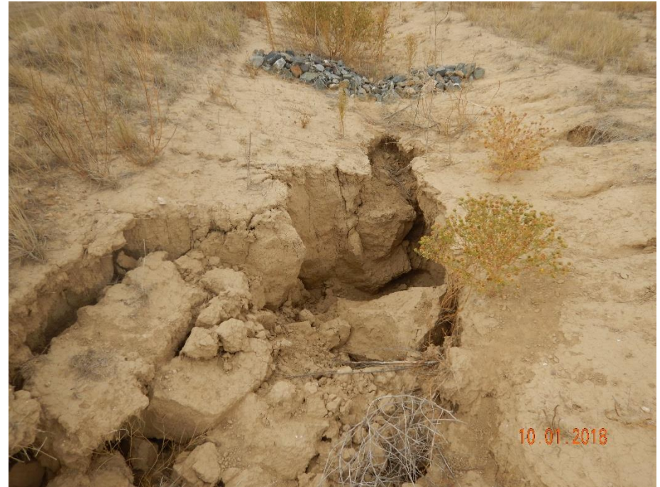
Photo 36: Continued from photo 32. Photo shows erosion degradation occurring, and sinkhole forming within the ditch on west end of the pad.
