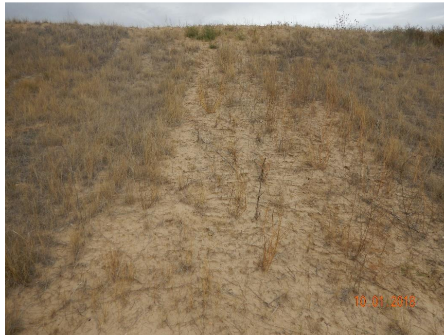
Photo 58: Photo taken from the west end of the location, facing east and upslope. Photo shows areas of the slope that remain predominantly bare and exposed soil. Operator has indicated that these areas had work conducted to repair erosion in 2016.
