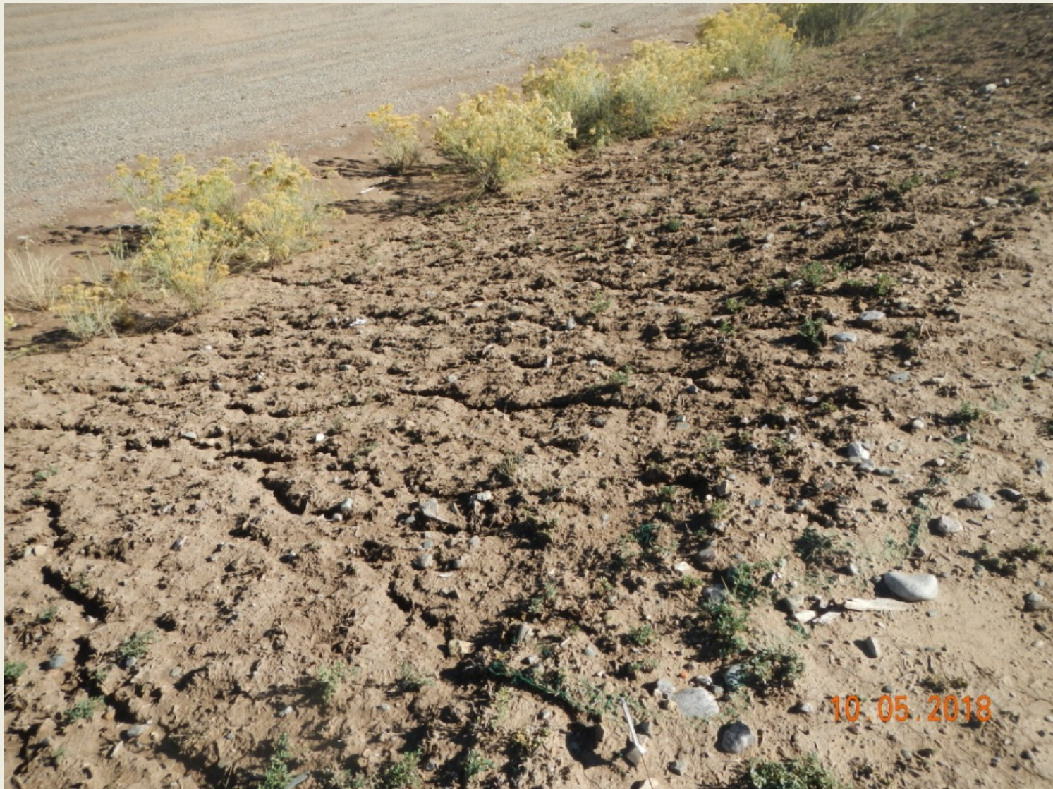
Photo 5. View of rilling in the central fill slope and poor revegetation facing down-slope.
