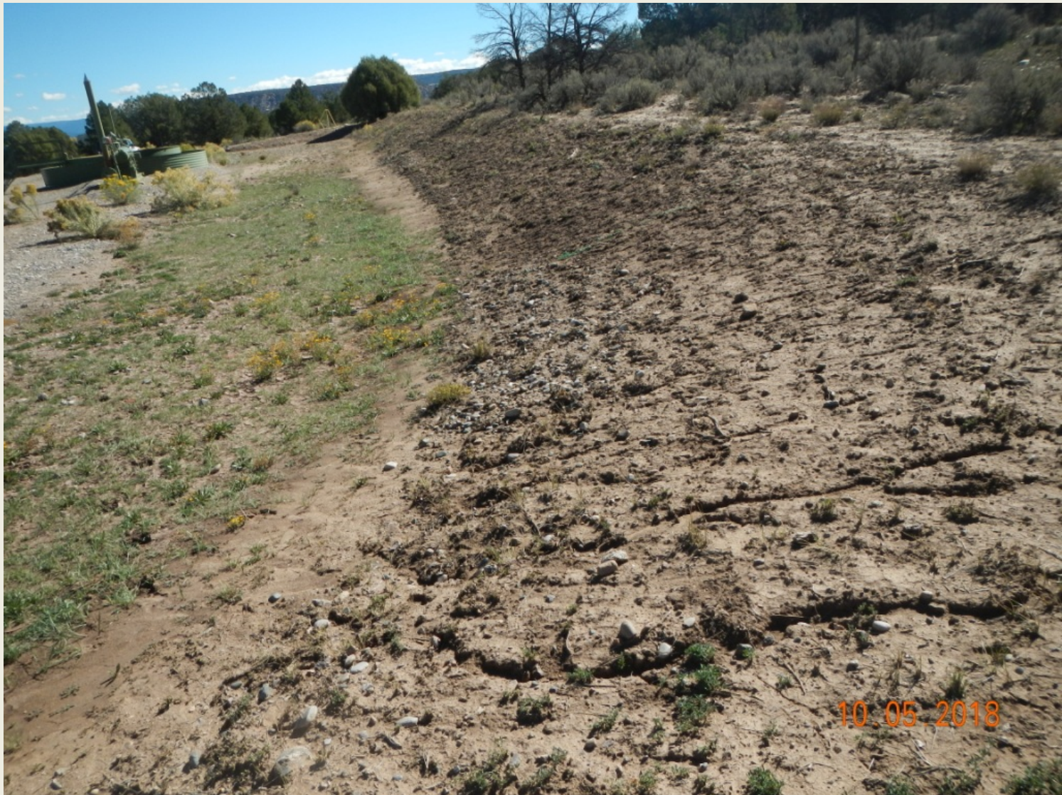
Photo 1. View of the southern portion of the project area from the southwestern corner facing eastward. Revegetation on well pad cut and fill slopes is sparse and appears to be drought stressed. This needs to be monitored and re-vegetation efforts conducted if vegetation is not increasing during the 2019 growing season. Rilling is occurring on the cut-slope.
