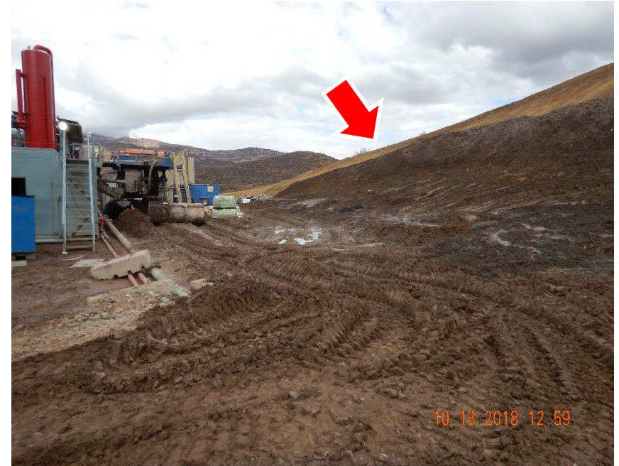
Photo #2 – View of cuttings pile (red arrow) from the south. Note absence of secondary containment berms and stormwater BMPs to isolate sediment and stormwater runoff from cuttings or to prevent tracking of material throughout pad.
