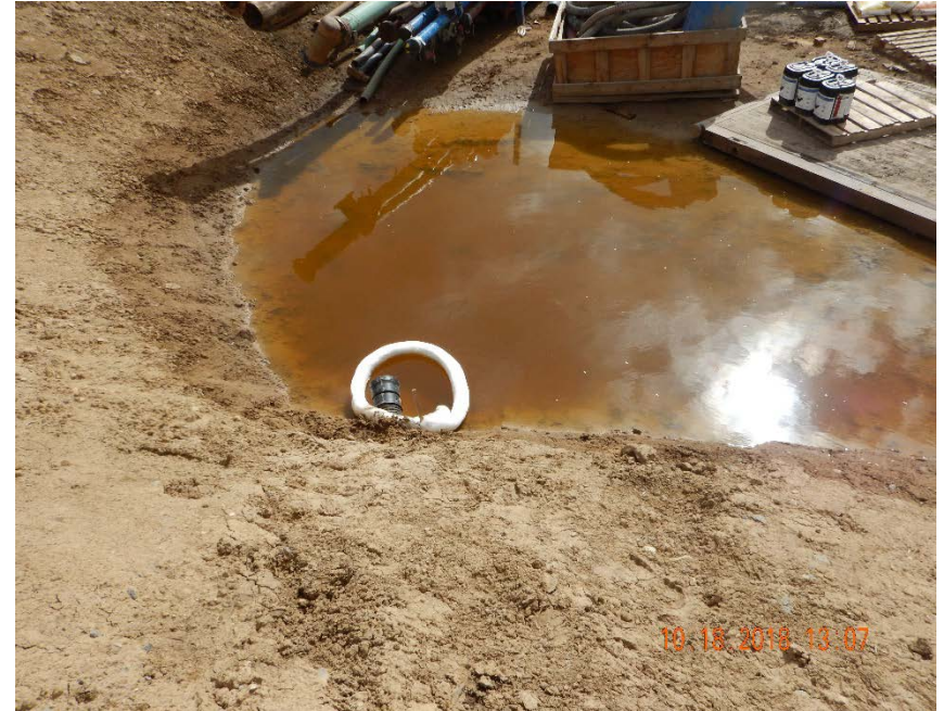
Photo #4 – Stormwater drain located at NE corner of pad. Note that there were no stormwater BMPs or secondary containment devices in place to prevent commingling of fluids from cuttings management pile with this area of the pad.
