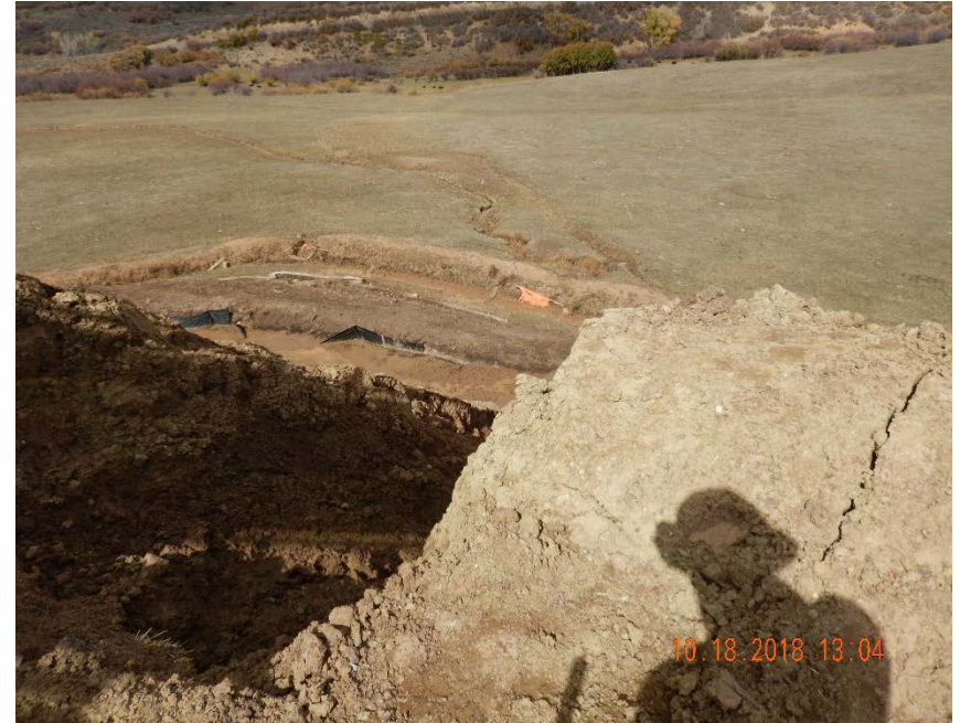
Photo #6 - Collapsed section of pad containment berm and fill slope located on north side of pad.
