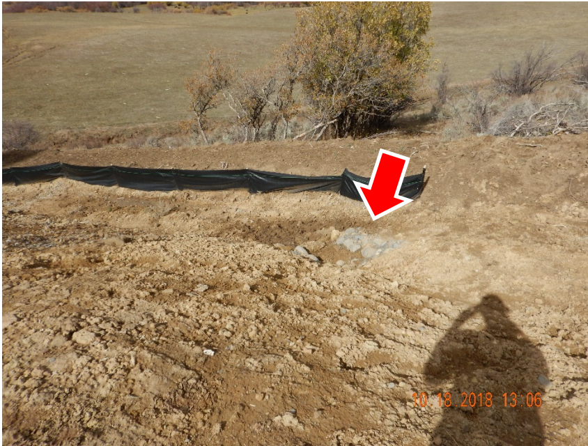
Photo #5 – Outlet of stormwater drain from previous photo (red arrow) and silt fence located north of pad.
