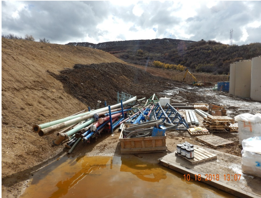
Photo #3 – View of cuttings pile (dark material) from NE corner of pad. Note storage of chemicals and equipment at NE corner of pad identical to Photo #9 included in 10/16/2018 Field Inspection Report (doc #692400233) photo log.
