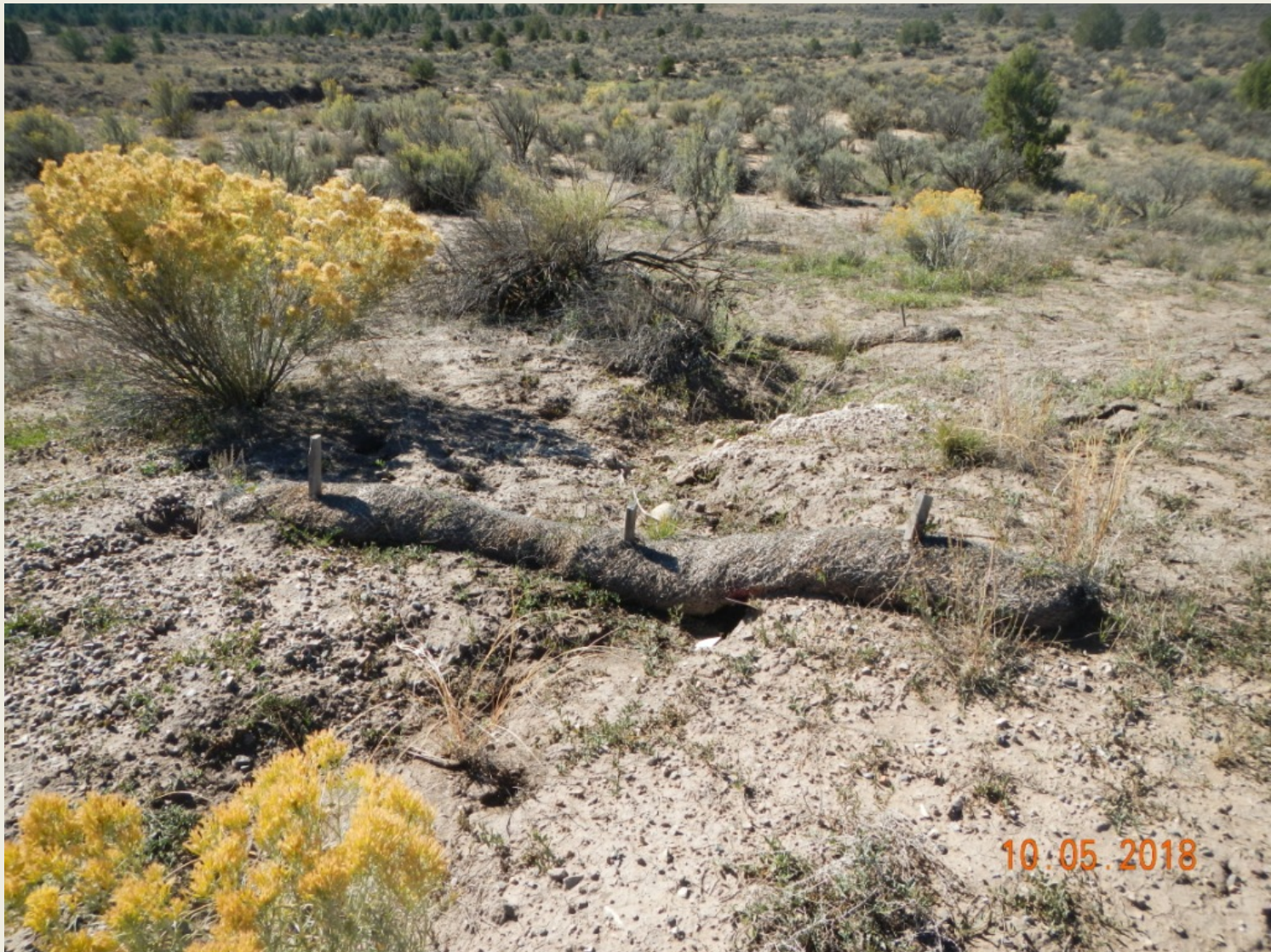
Photo 6. View of wattle in the southern project area that is no longer functioning. Soils are not stabilized.
