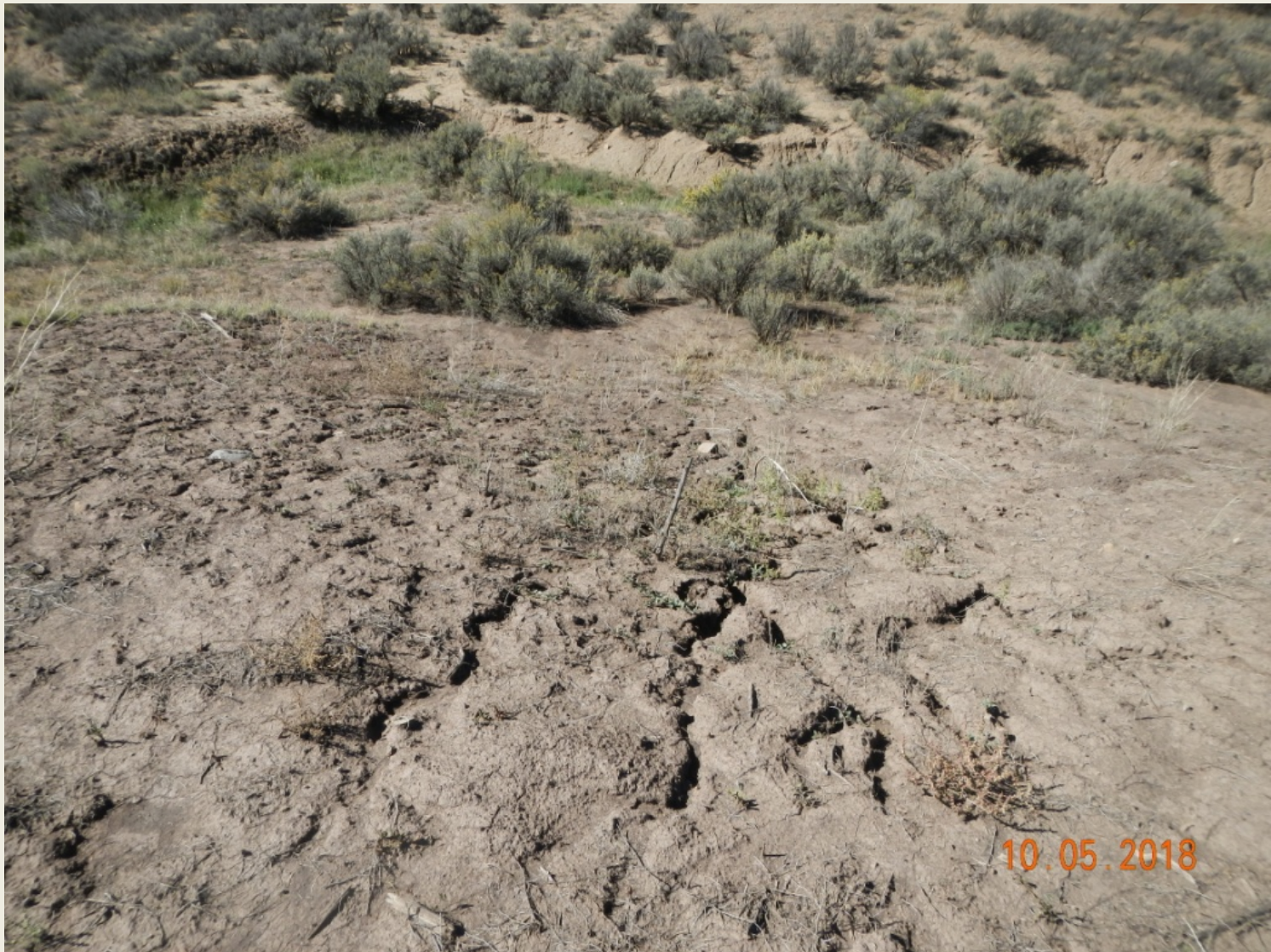
Photo 5. View of rilling in the southeastern fill slope. Erosion control measures are needed to stabilize erosion on fill slopes.
