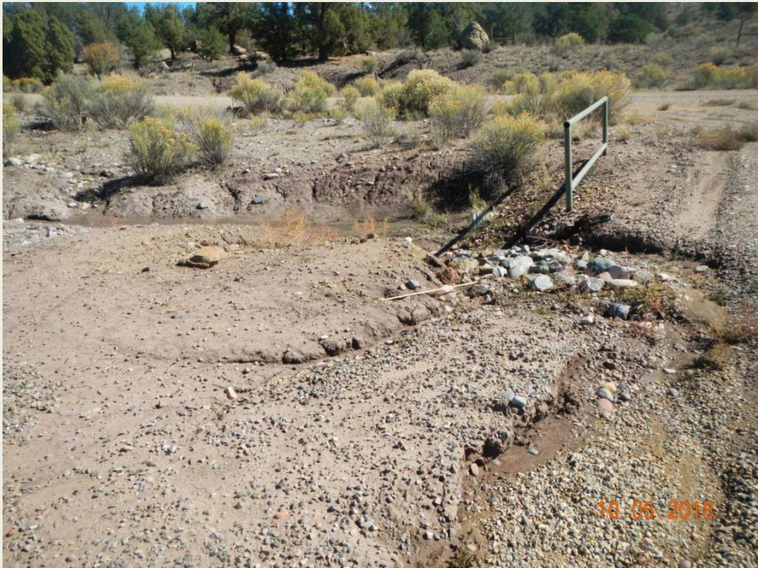
Photo 8. View of erosional channeling at southeastern entrance to southern portion of the well pad. Stabilization measures are needed here.
