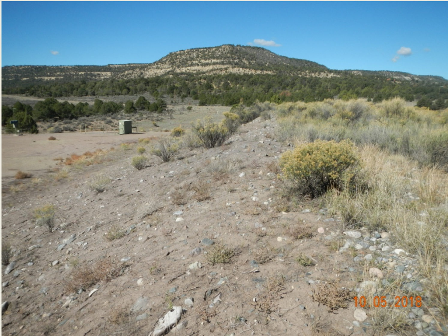
Photo 2. View of the fill slope within the central portion of the project area from the eastern edge facing westward. Rilling is occurring on the fill slope from the northern portion of the well pad.
