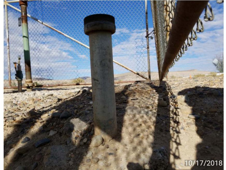
Riser uncapped and no lock out tag out
