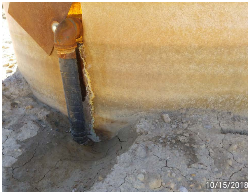
Tank leaking fluid
