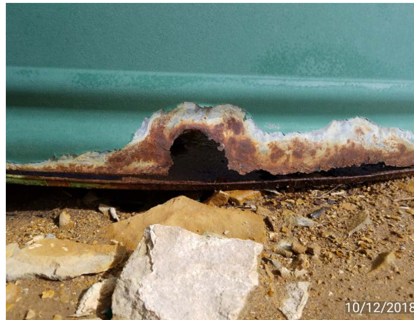
Hole in side of 25 bbl tank
