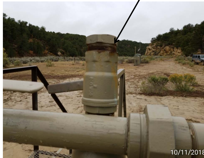
Gas leaking around threads of cap.
