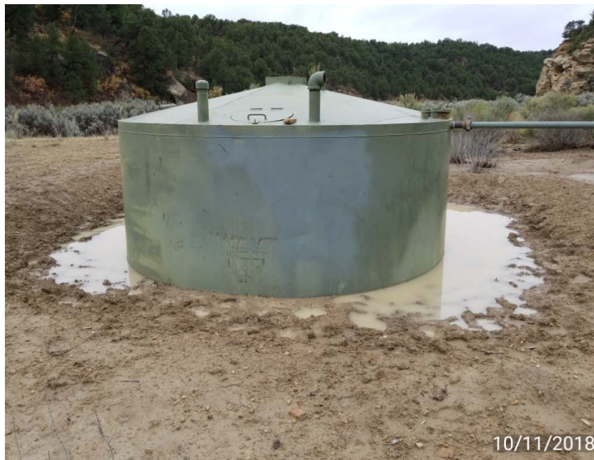
Tank missing labeling. Storm water passing through berm during heavy rainfalls.
