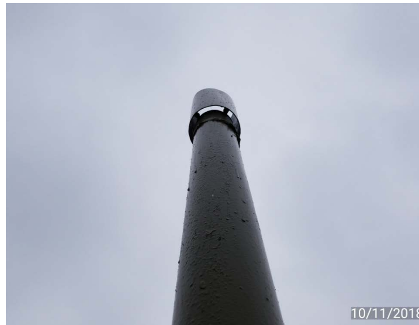
Missing bird protection on separator stack.
