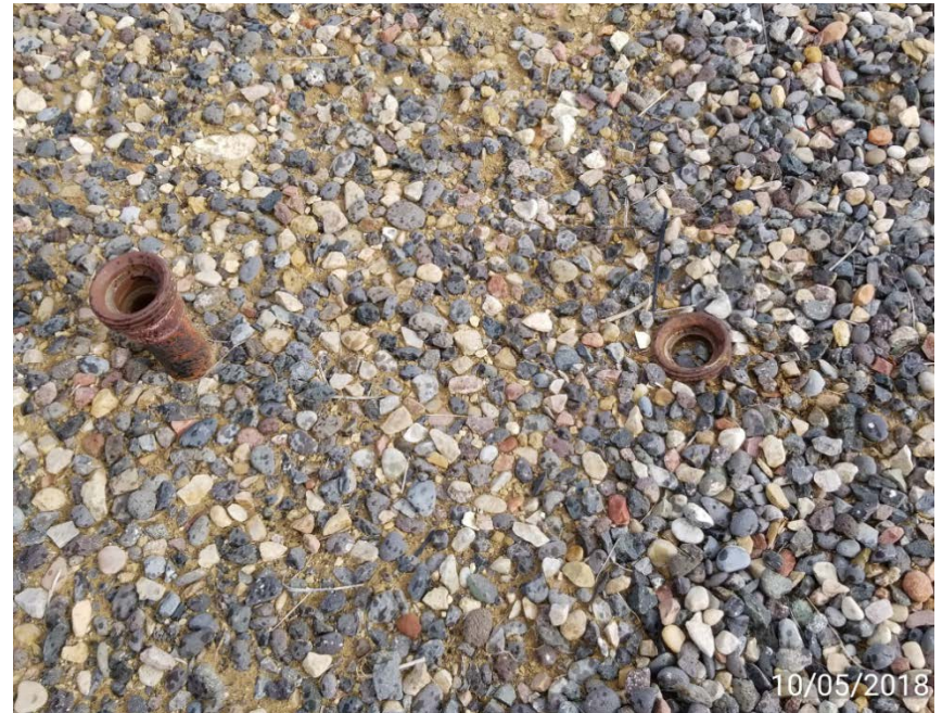
Risers without ends sealed or locked out tag out. Located next to well head.
