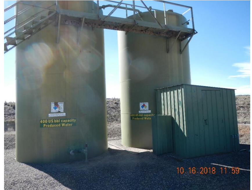
Quintana 32-6 #15-2 tank battery.
