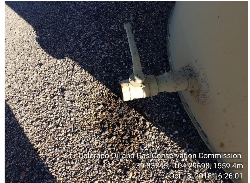
Photo 4 Stained soil load line crude oil tank
