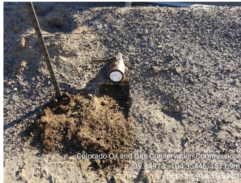
Photo 4 Stained soil crude oil load out line
