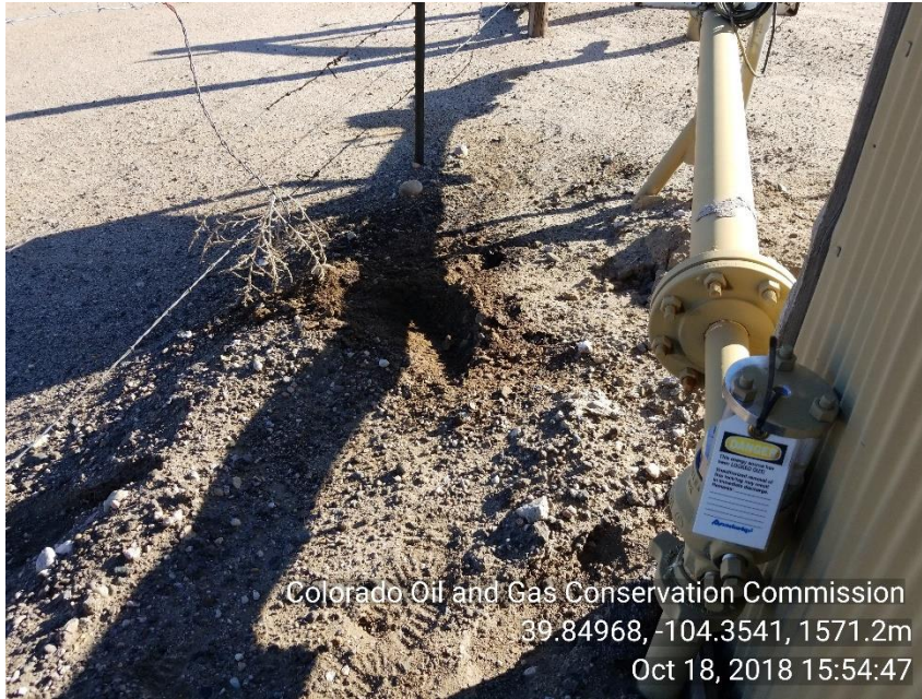
Photo 5 Stained soil by meter run. Meter run locked out tagged out
